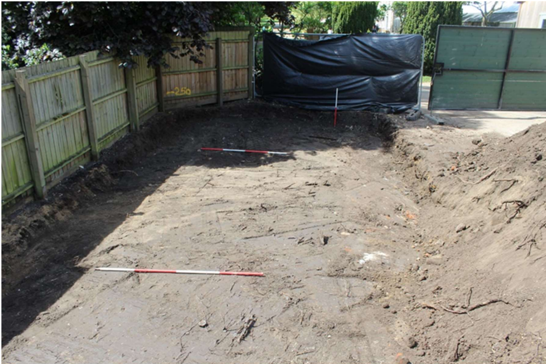
Plate 8. Area 3 (the efford bed) following excavation looking west. The depth of the ground level reduction coincided with the top of a dark earth layer, 016, an extensive layer of town rubbish deposited across the site sometime during the 17-18th century.
