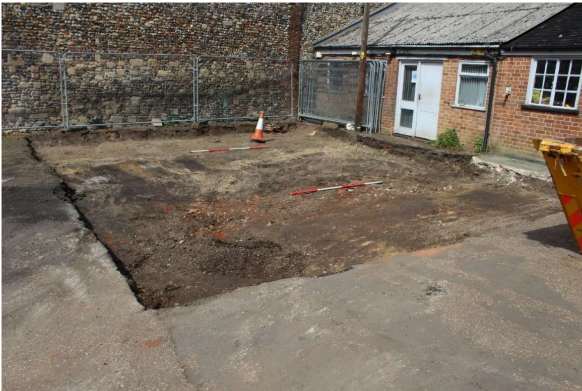
Plate 6. Area 2, excavation of the skip hardstands looking NE, scales 2m.
