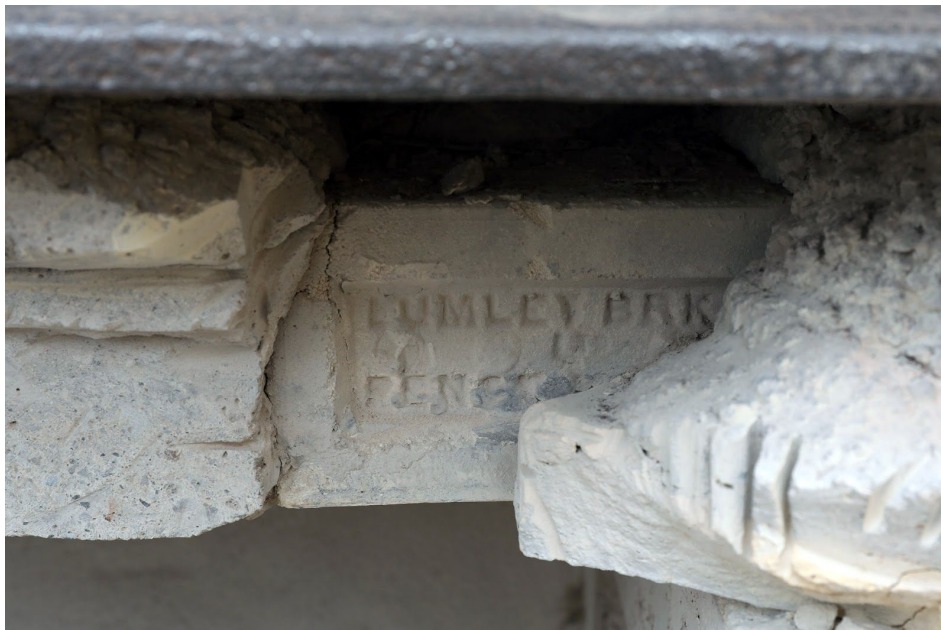
Figure 12 Lumley Brick forming the soffit of the opening, immediately behind the composite capital at the right side of the entranceway. © Solway Past
