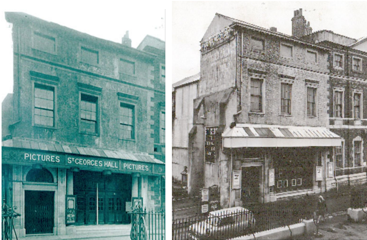
Figure 7 (Left) A photograph of the site in the 1920s showing the original design and canopy for St George's Hall, and (Right) the same canopy in 1965 © York Press
