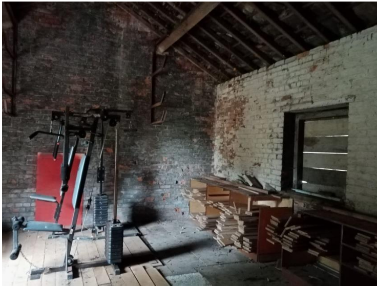
Figure 20 View of the first floor space
