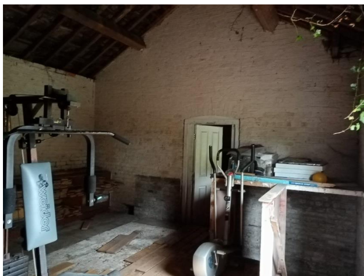
Figure 19 View of the first floor space
