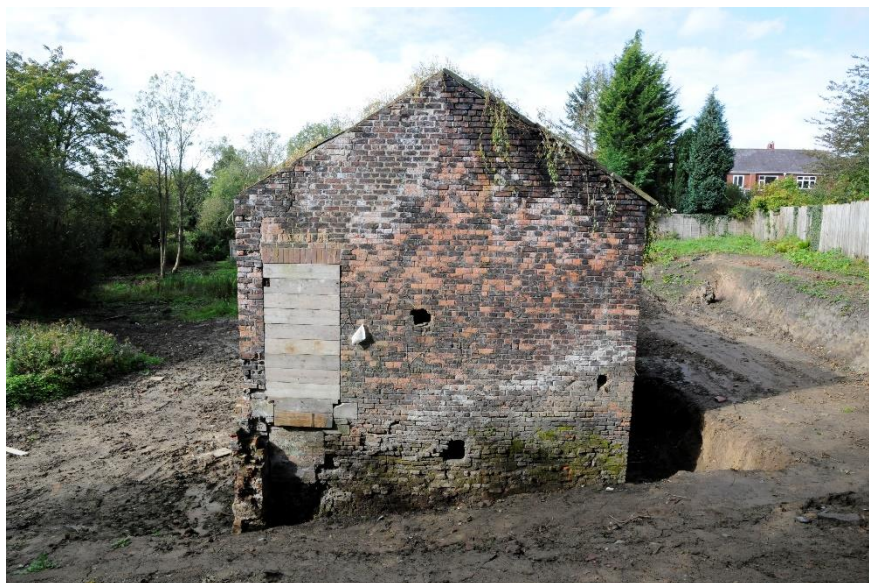
Figure 12 The east gable elevation with elevated opening
