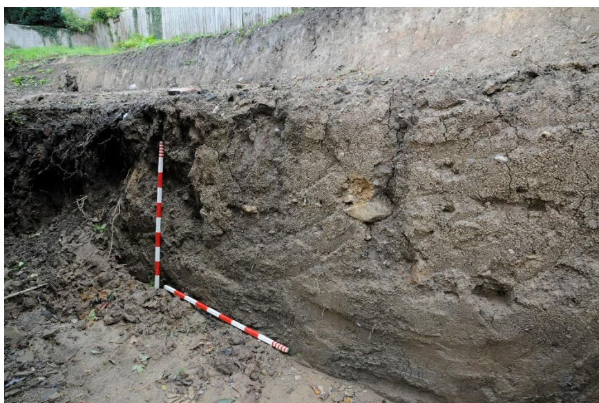
Figure 14 The section / face of the embankment at the north side of the building
