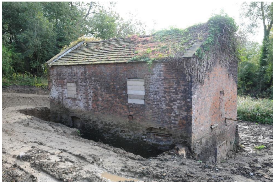
Figure 10 The north-facing elevation; note the height of ground level
