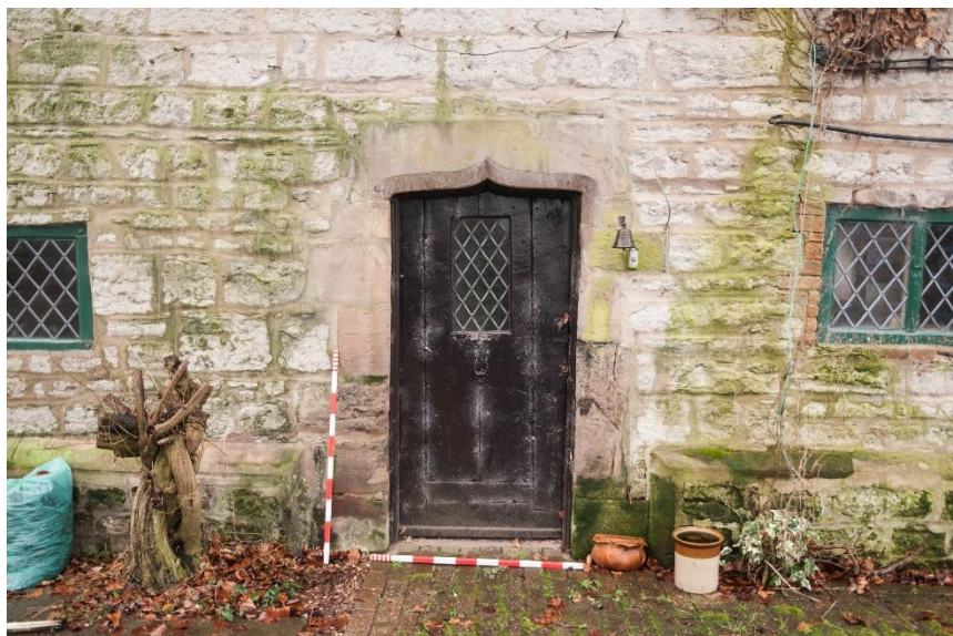
Figure 18 The through passage opening on the east elevation
