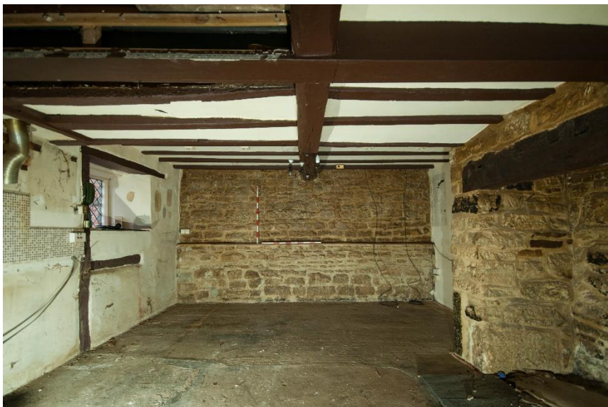
Figure 29 Room G4, looking north
