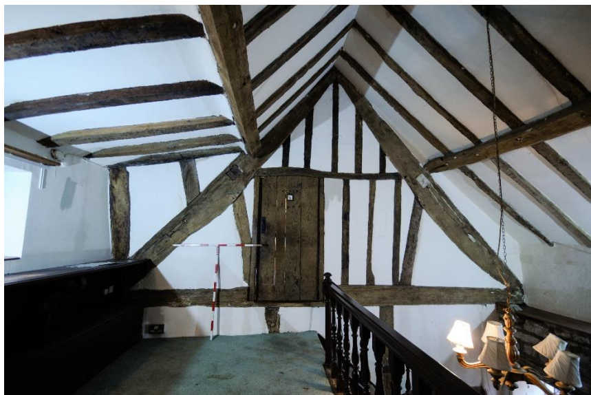
Figure 34 Room F1, looking south and showing one of the original partitions
