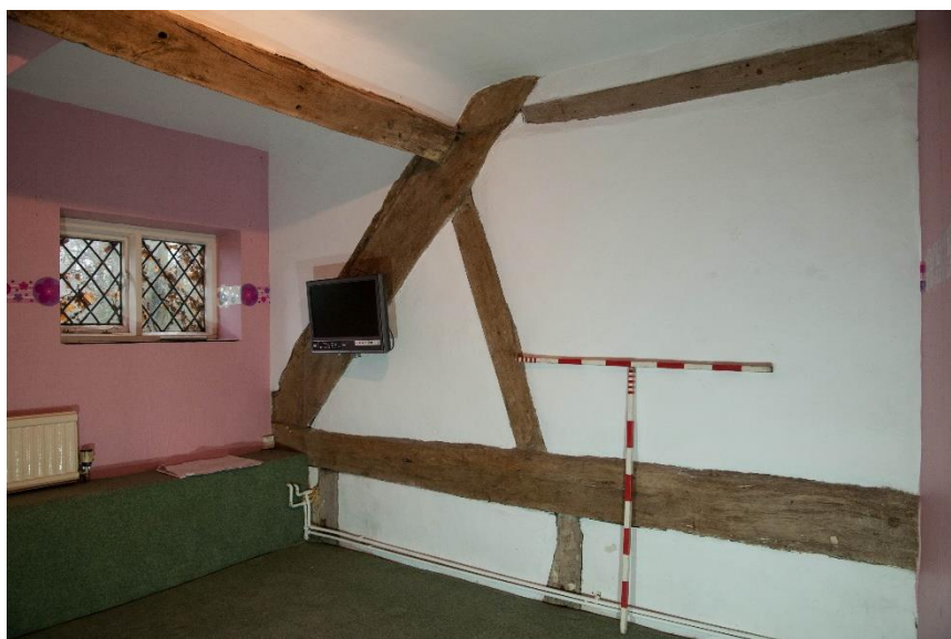
Figure 49 Room F7, showing the partition to Room F6
