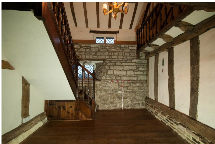
Figure 22 Room G2, looking east, showing the stair up and projecting galleried walkway
