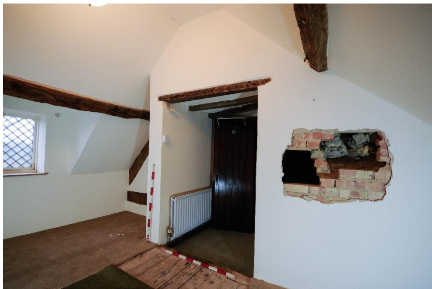
Figure 51 Room F8, looking south-east. Note modern brick flue
