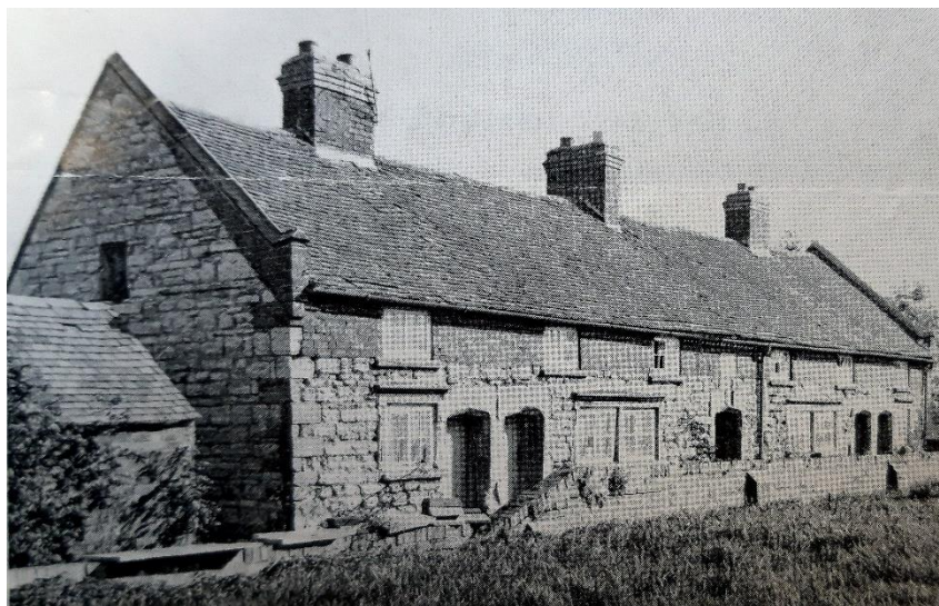
Figure 4 Undated early 20th century view of the west and north elevations (Ensor 2020)
