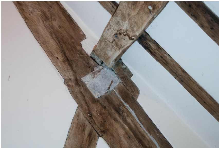
Figure 42 Room F2, detail of altered purlin on south partition
