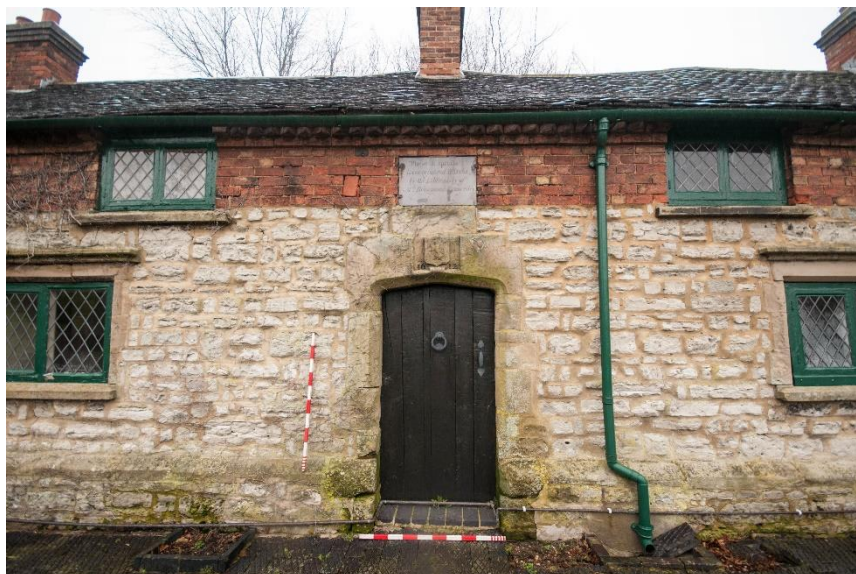
Figure 6 The central doorway to the former through passage with commemorative plaques above
