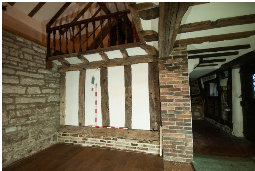
Figure 23 Room G2, looking north and showing modern brickwork with a modern stud partition behind the modern fireplace
