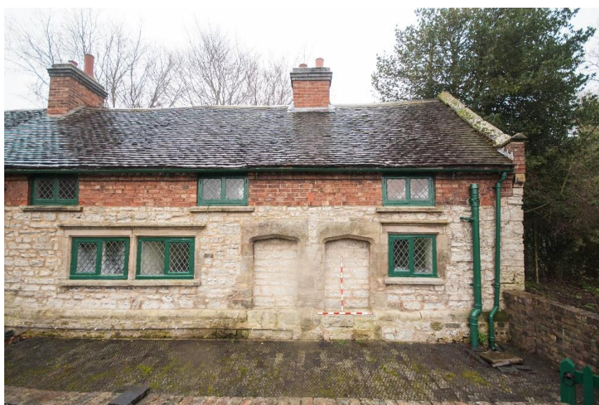
Figure 5 The southern end of the west elevation, showing blocked paired doors and the raised eaves
