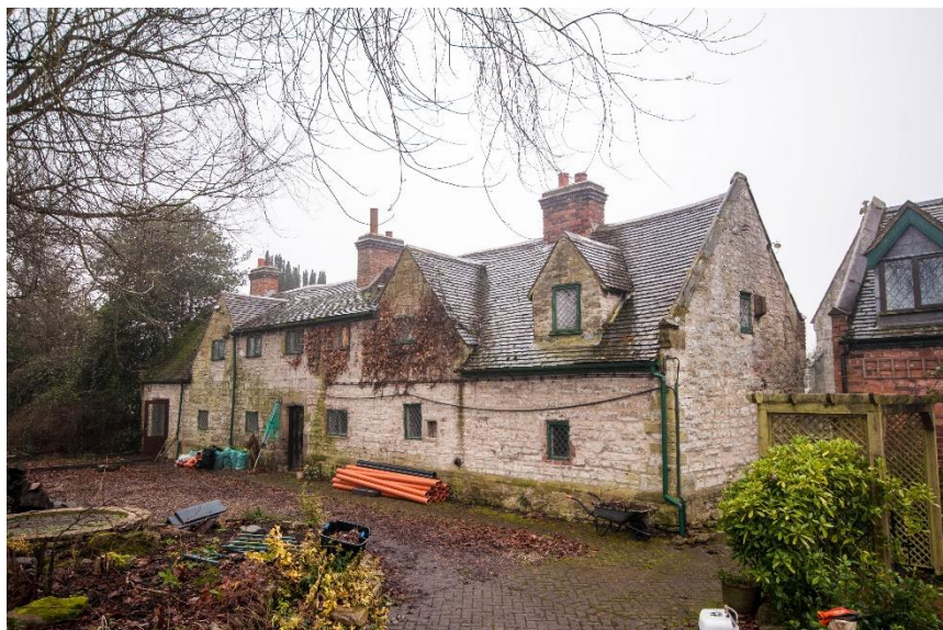
Figure 14 General view of the building from the north-east, showing the north and east elevations
