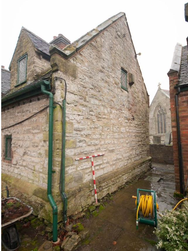
Figure 13 The north elevation, looking south-west
