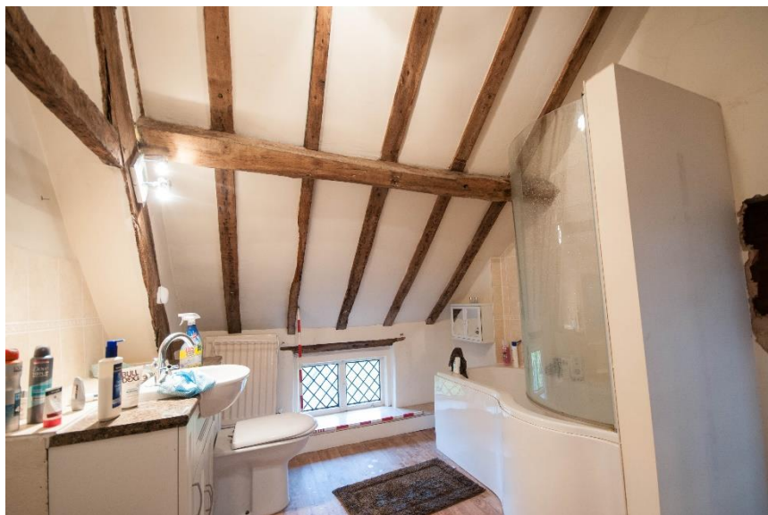
Figure 45 Room F2, looking west and showing purlin and rafters
