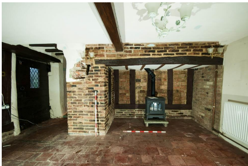
Figure 25 Room G3, looking south and showing the modern brick built 'inglenook'
