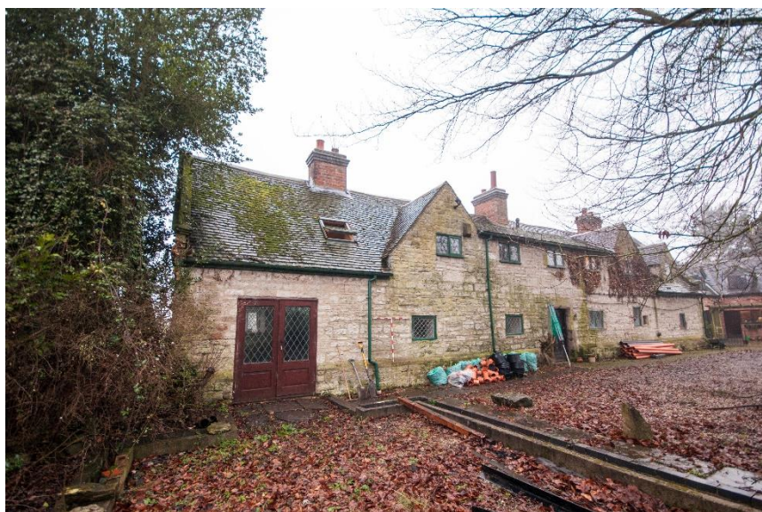
Figure 19 View of the east elevation, looking north-west
