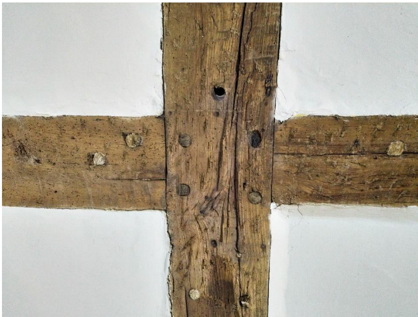
Figure 28 Detail of the timber joins on the north wall of Room G3, showing pegs and faint set-out lines
