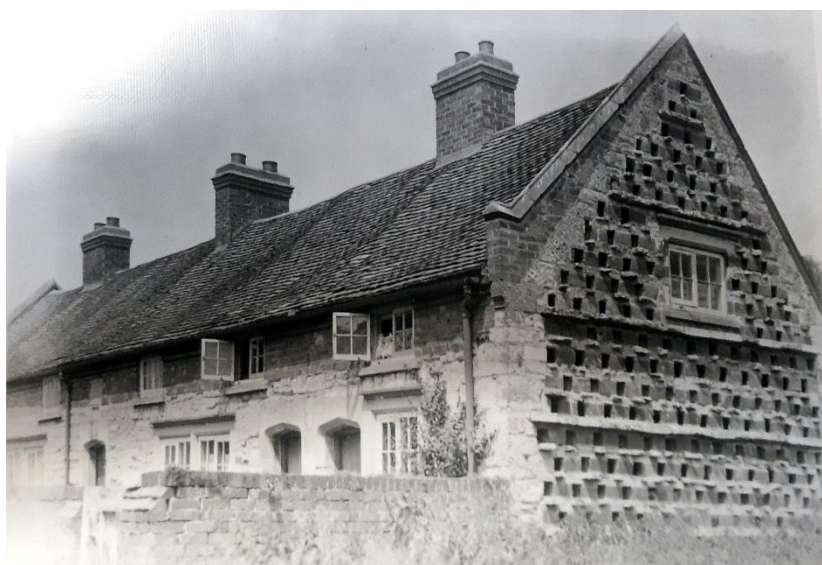
Figure 11 Undated early 20th century of the south elevation (Ensor 2020)
