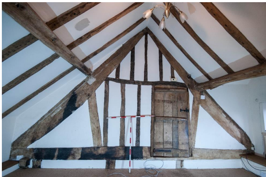
Figure 36 Room F2, the south side of the historic partition
