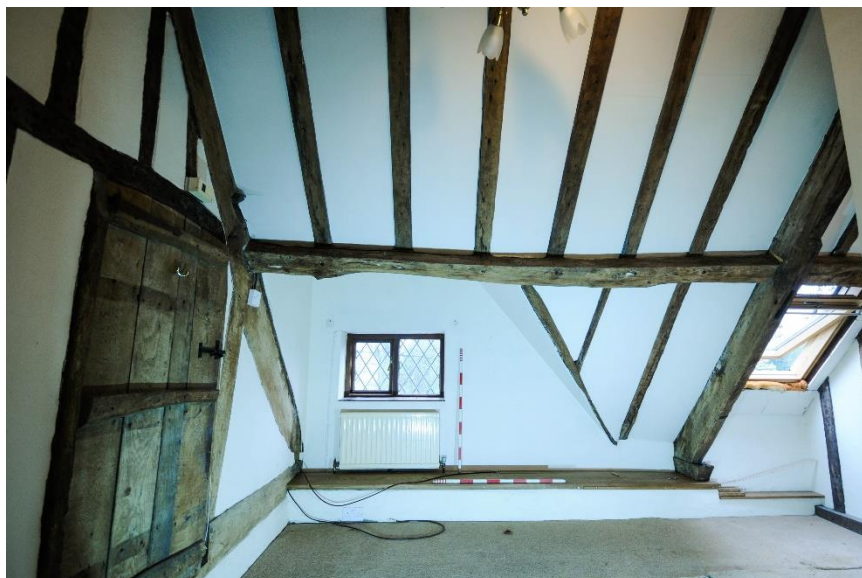
Figure 40 Room F2, looking east; note removed joists to accommodate modern dormer
