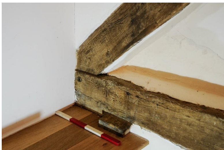
Figure 53 Rom F8, detail of rafter / tie beam join with remnant wallplate
