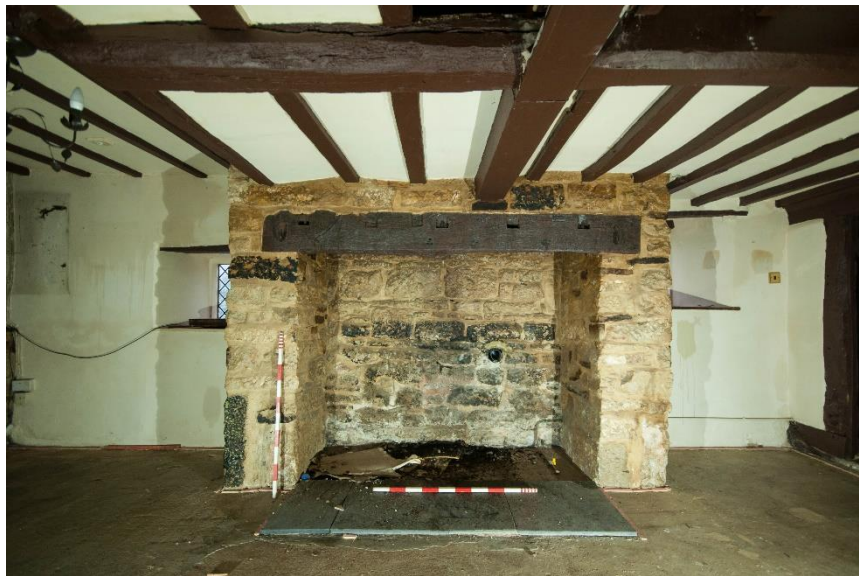
Figure 30 Room G4, showing the modern fireplace with re-used lintel
