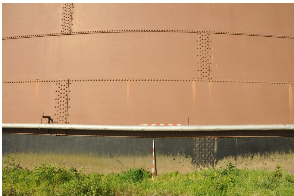
Figure 5: Detail of the tank structure.
