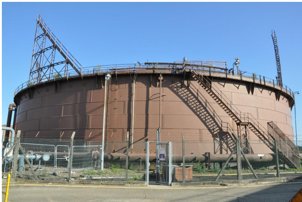
Figure 4 General view of the gasholder, looking north-west.
