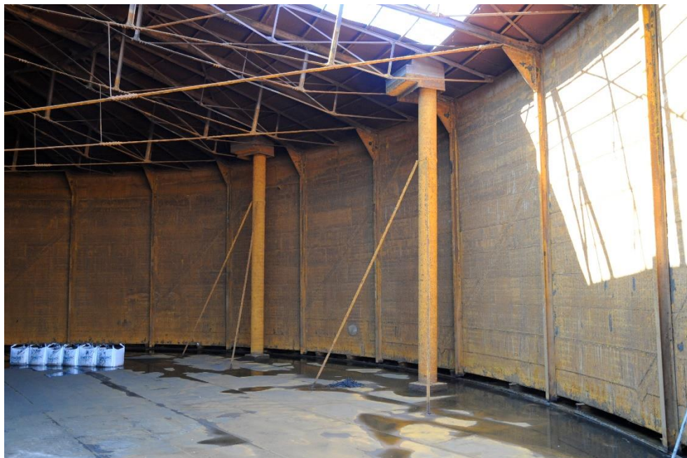
Figure 16 The inlet and outlet pipes.
