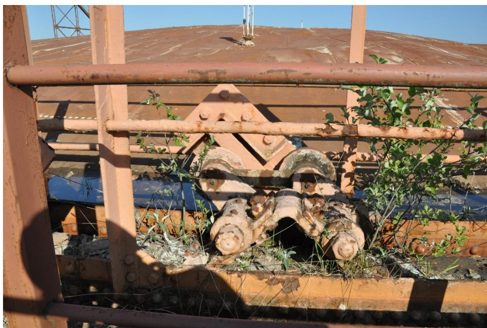
Figure 13: Example of the lift roller carriages.
