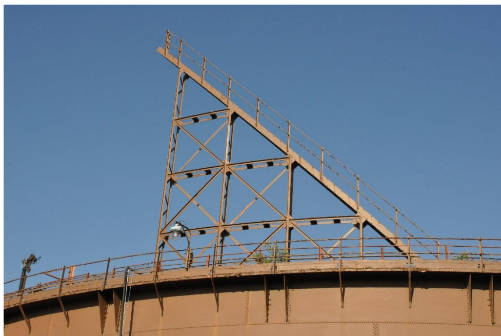
Figure 9: Example of the lift stairs.
