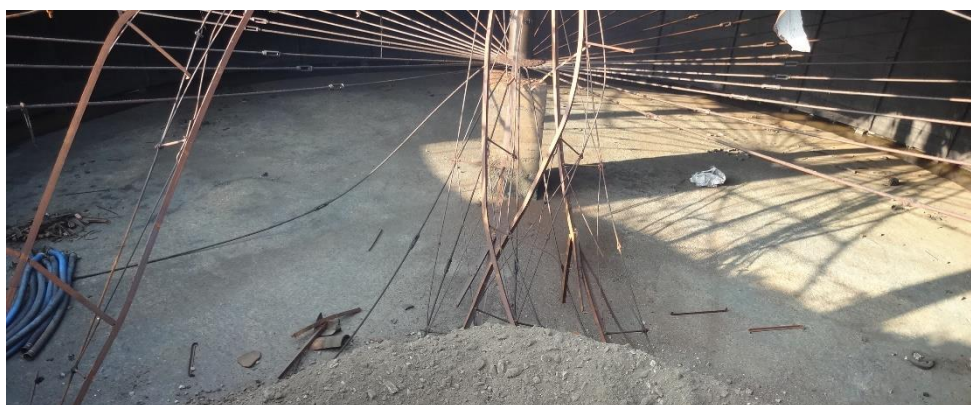
Figure 6 Gasholder 2, view of the central crown frame supporting column
