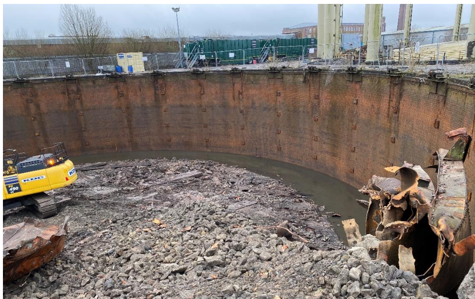
Figure 4 Gasholder 1, view of the brick tank with lifts removed
