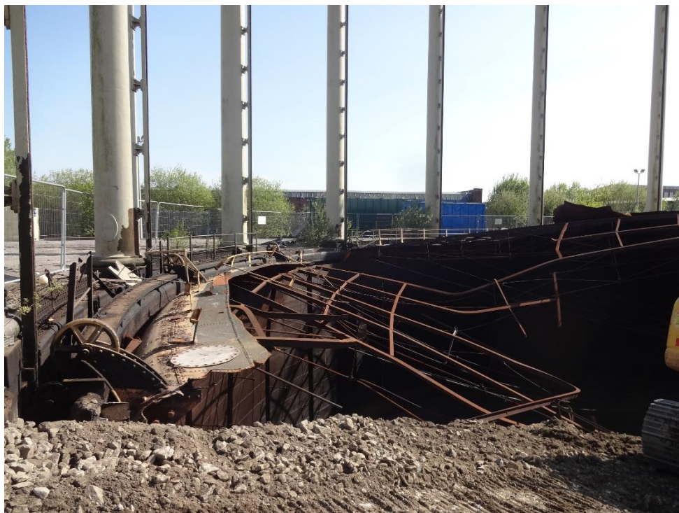
Figure 5 Gasholder 2, the crown frame during demolition
