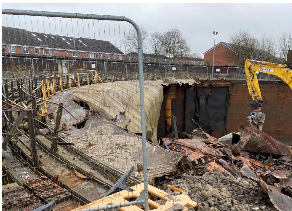
Figure 2 Gasholder 1, the crown during removal. Note hydraulic lid to pipe
