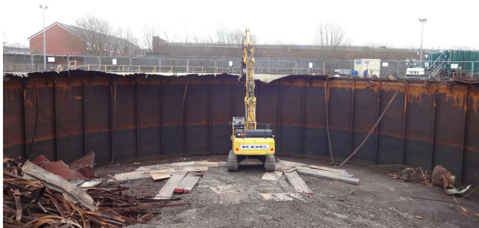
Figure 3 Gasholder 1, the gasholder interior with crown frame removed
