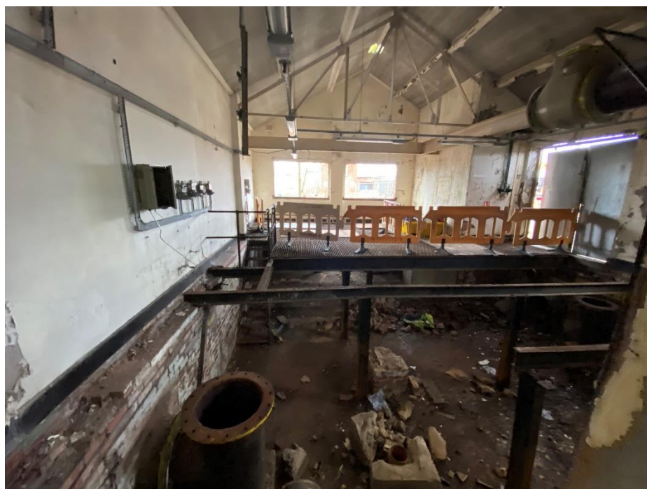
Figure 11 Interior of the Governor House with floor removed
