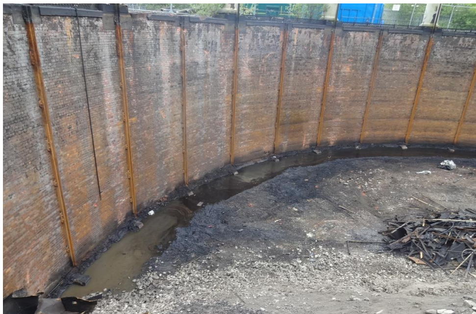
Figure 8 Gasholder 2, view of the brick tank following removal of the ifts
