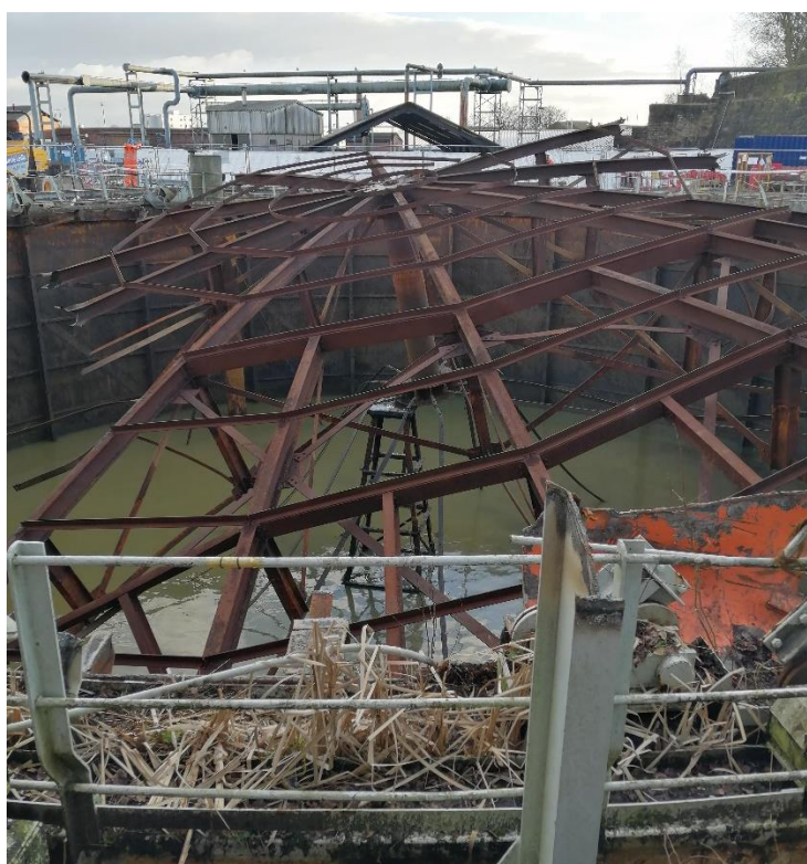
Figure 12: Gasholder 1, view of the crown frame and stanchion.
