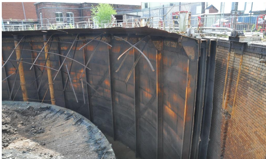
Figure 23: Gasholder 3, view of lifts and tank, also showing inlet / outlet pipes.
