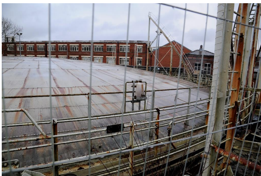
Figure 22: Gasholder 3, general view of the crown, looking east.
