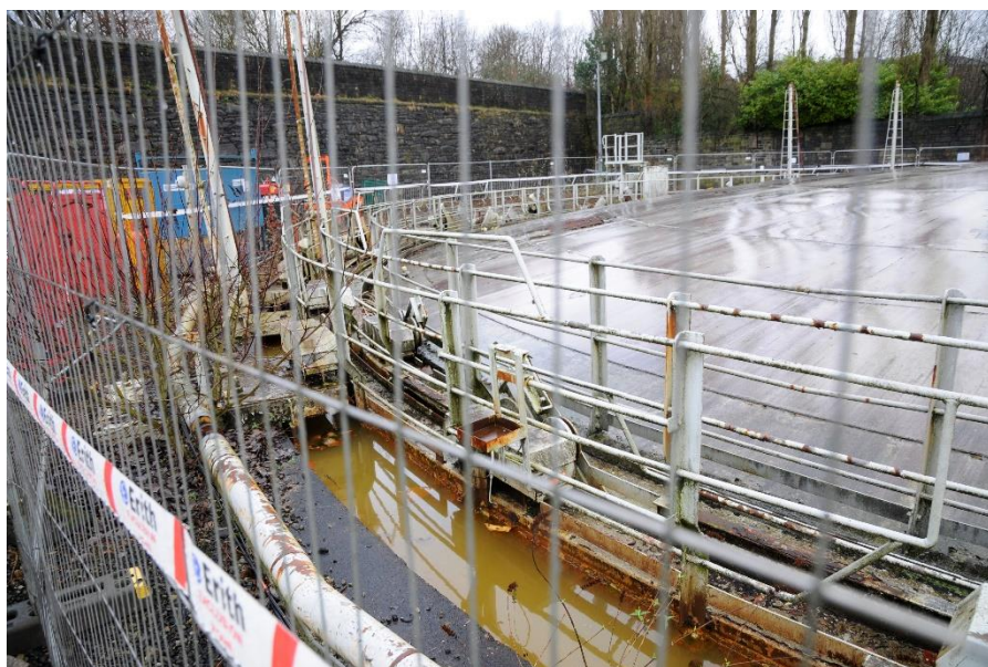
Figure 10: Gasholder 1, view of the lifts and crown.
