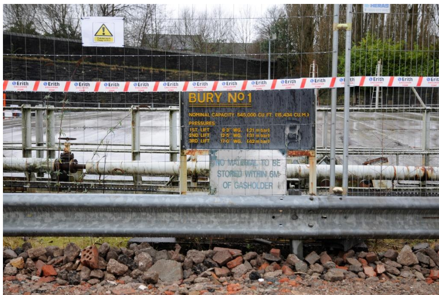
Figure 6: Gasholder 1 designation plaque and information.
