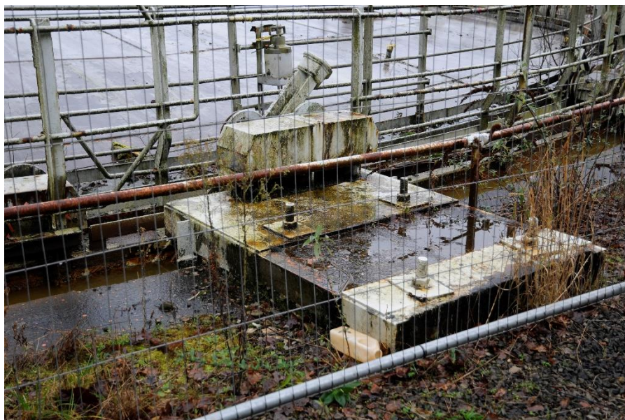
Figure 9: Gasholder 1, an example roller carriage on a former column pad.
