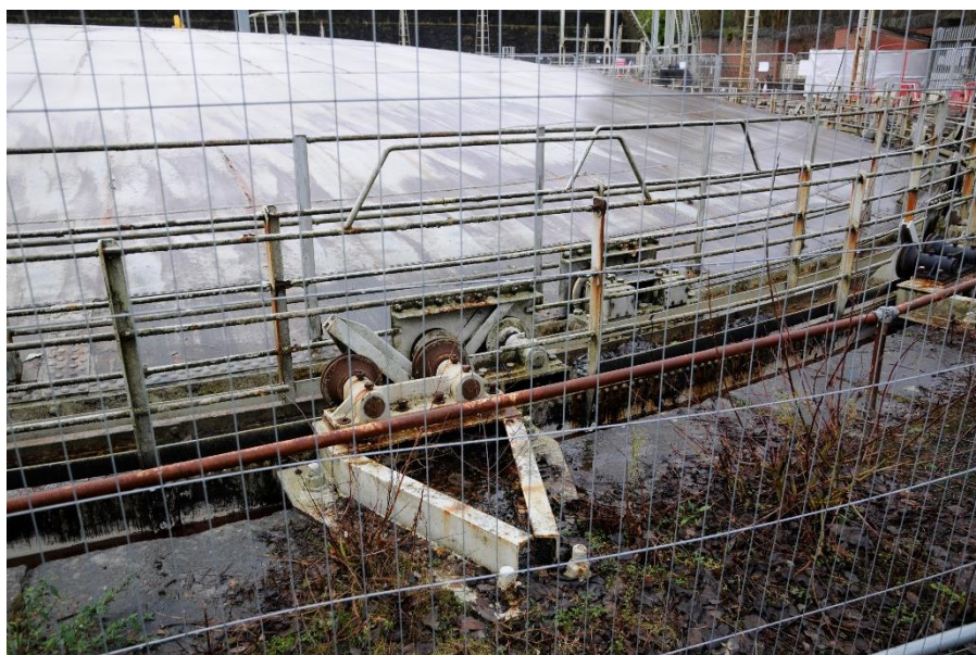
Figure 20: Example of the roller carriages with tapered design.
