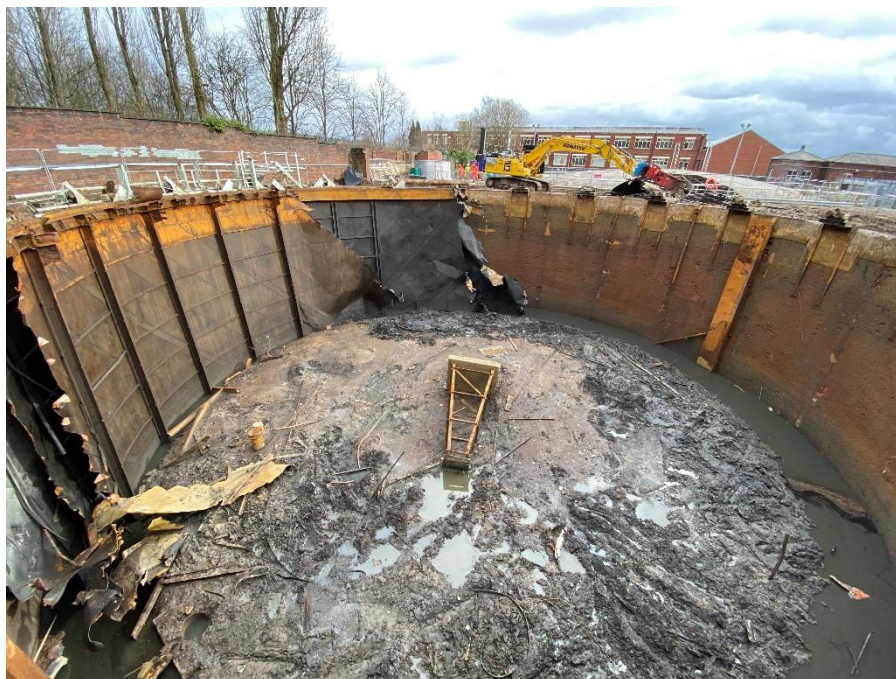
Figure 13: Gasholder 1, view of the tank.
