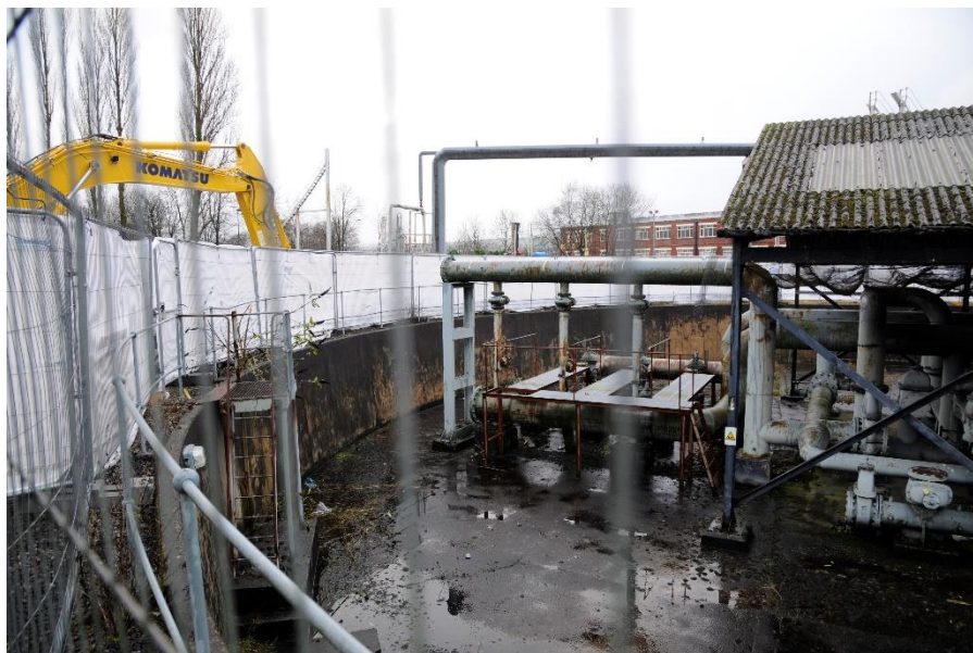
Figure 15: View of the former tank to Gasholder 2 with PRS Station.
