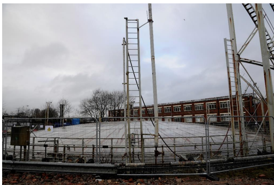
Figure 18: Gasholder 3, looking north-east, showing one of the anti-freeze supports.
