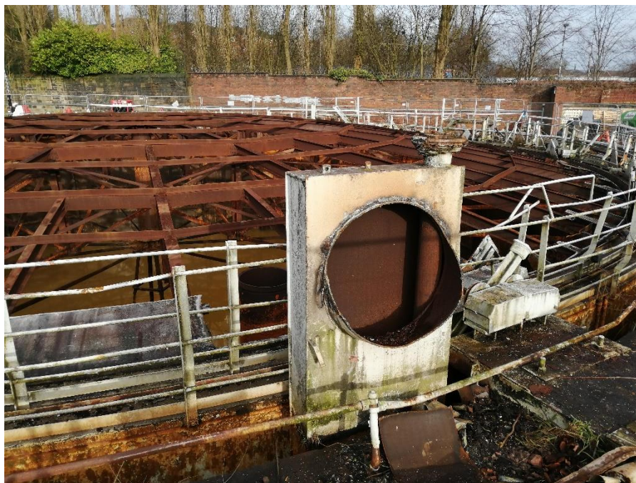
Figure 11: Gasholder 1, view of the crown frame, looking north.
