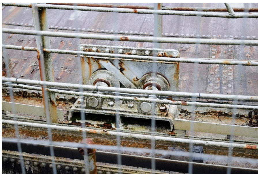
Figure 21: Gasholder 3, example of the lift rollers with run-out stop plate.
