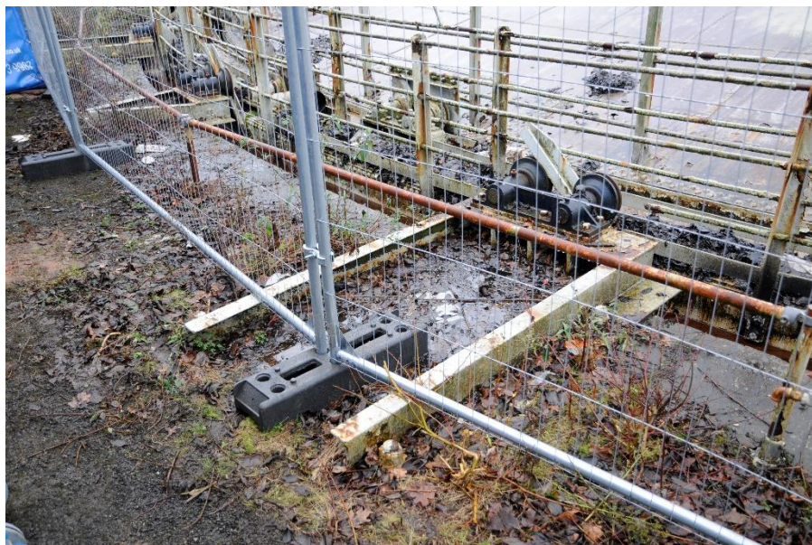
Figure 19: Example of the roller carriages located on a former column base.
