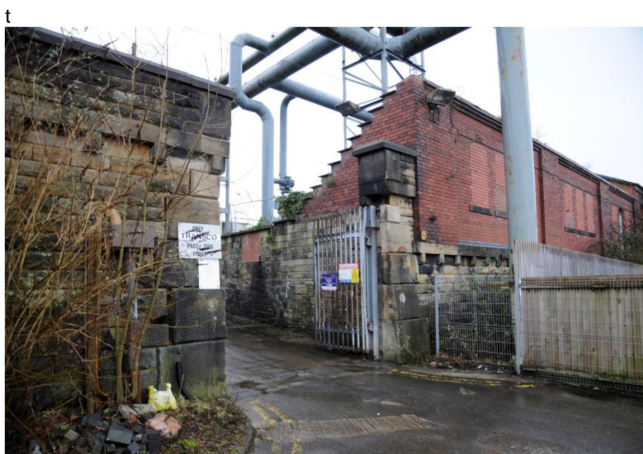
Figure 27: The south wall of the laboratory building and the site entrance.
