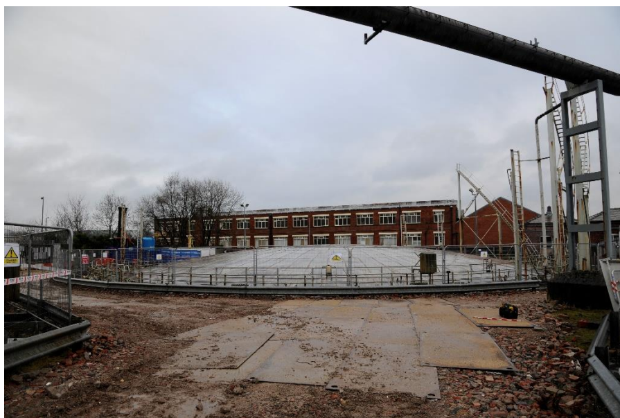
Figure 16: Gasholder 3, looking east.
