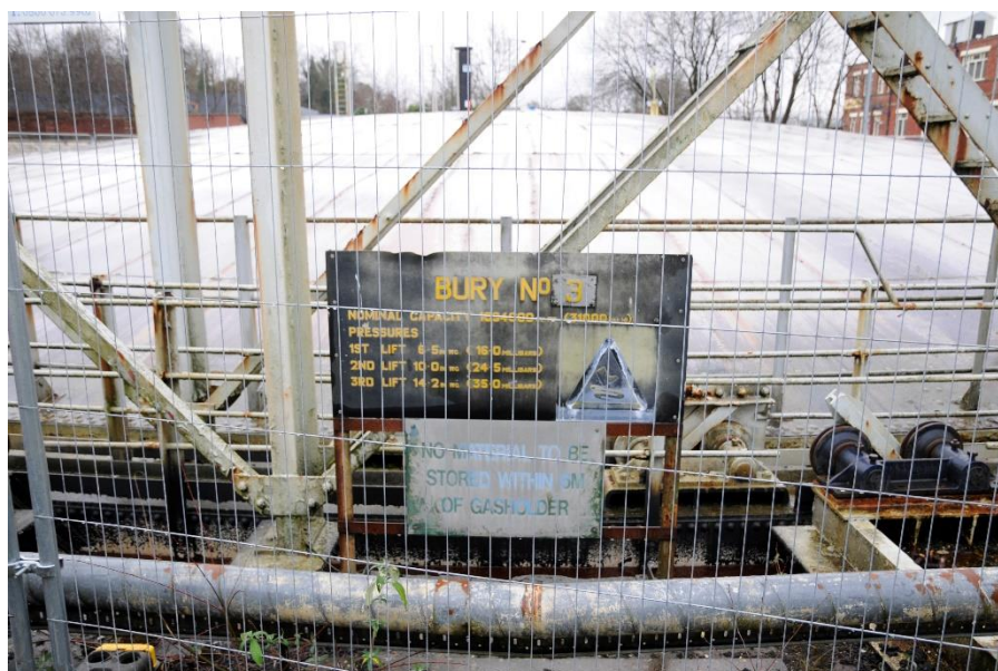
Figure 17: Gasholder 3 designation plaque and information.
