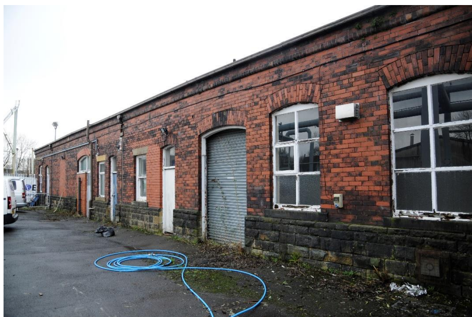
Figure 26: The west elevation of the former laboratory building, looking north-east.
