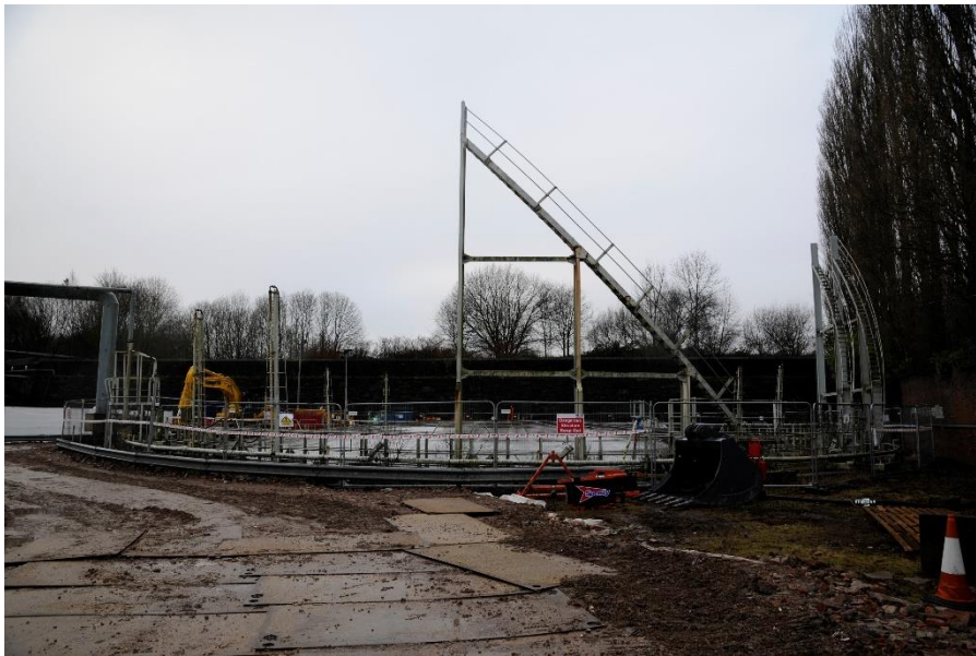
Figure 5: Gasholder 1, looking west.
