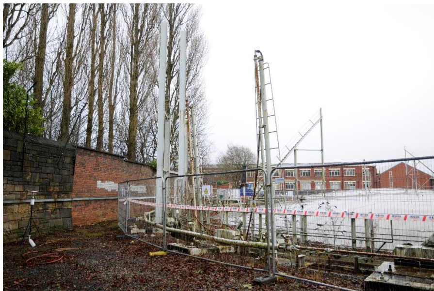
Figure 7: Gasholder 1, anti-freeze pylons at the north side of the gasholder.
