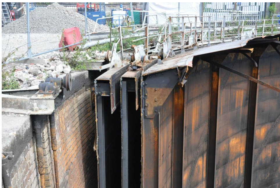
Figure 25: Gasholder 3, detail of the top curb and lift grips.
