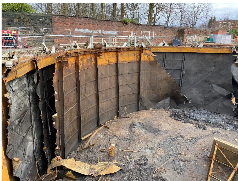
Figure 14: Gasholder 1, view of the lifts and grips.
