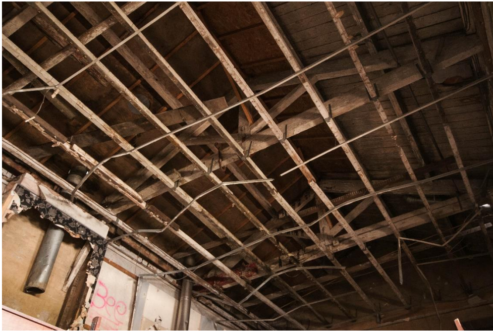
Figure 35 View of the roof structure
