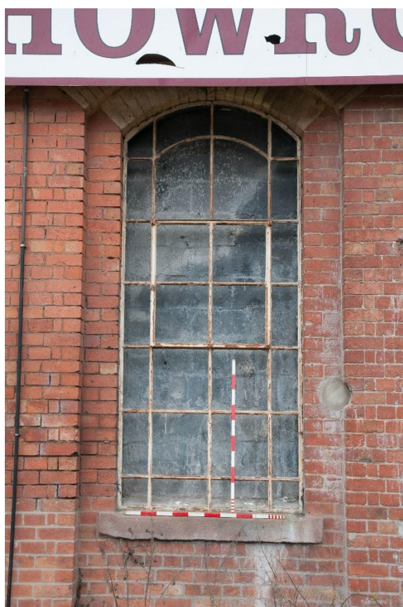
Figure 15 Detail of the windows
