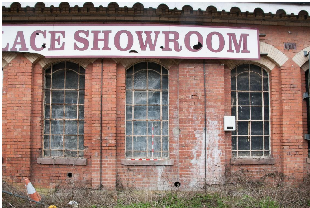
Figure 14 View of the windows
