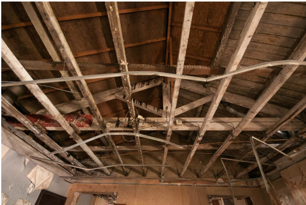
Figure 36 Example of the roof trusses
