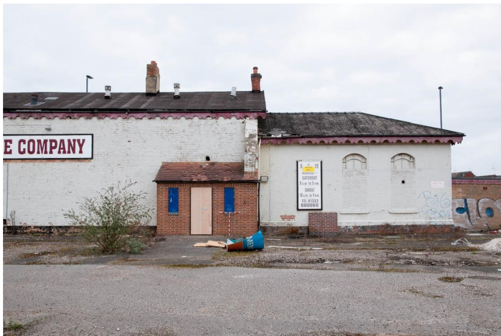
Figure 4 The east end of the south elevation with modern porch
