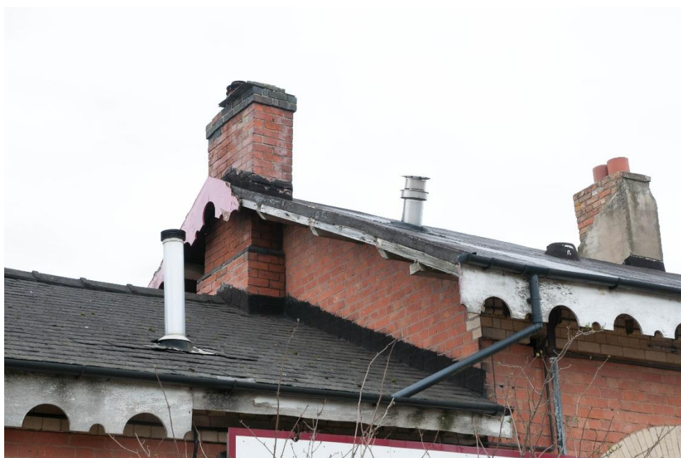
Figure 12 The east gable of the main block
