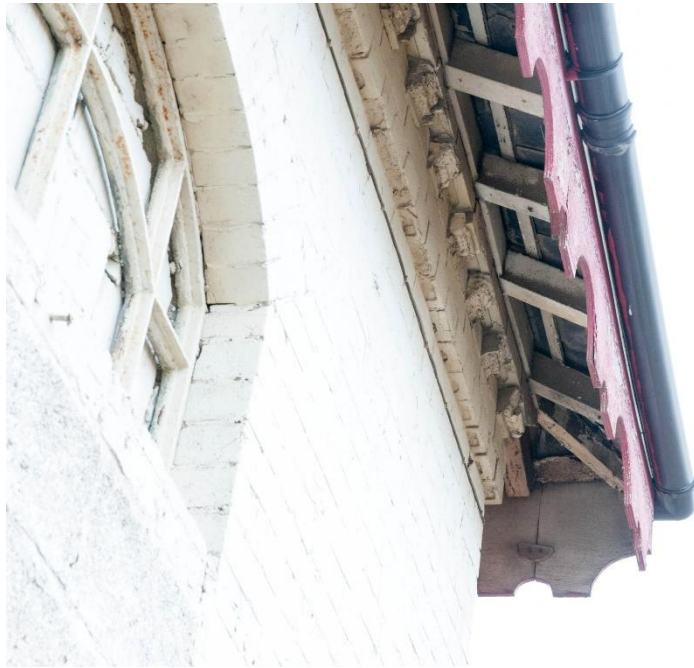
Figure 9 Detail of the cornice, dentils and projecting rafter ends
