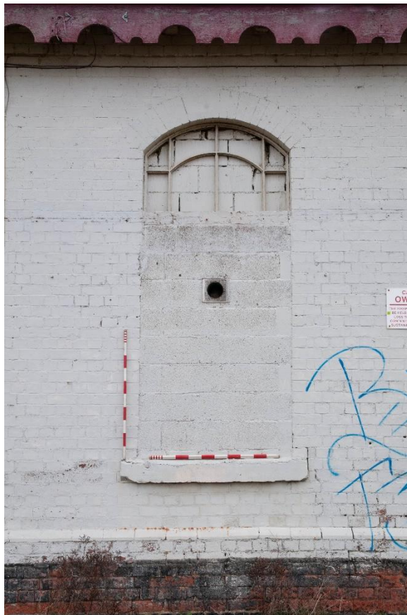
Figure 7 Detail of blocked window on single-storey block
