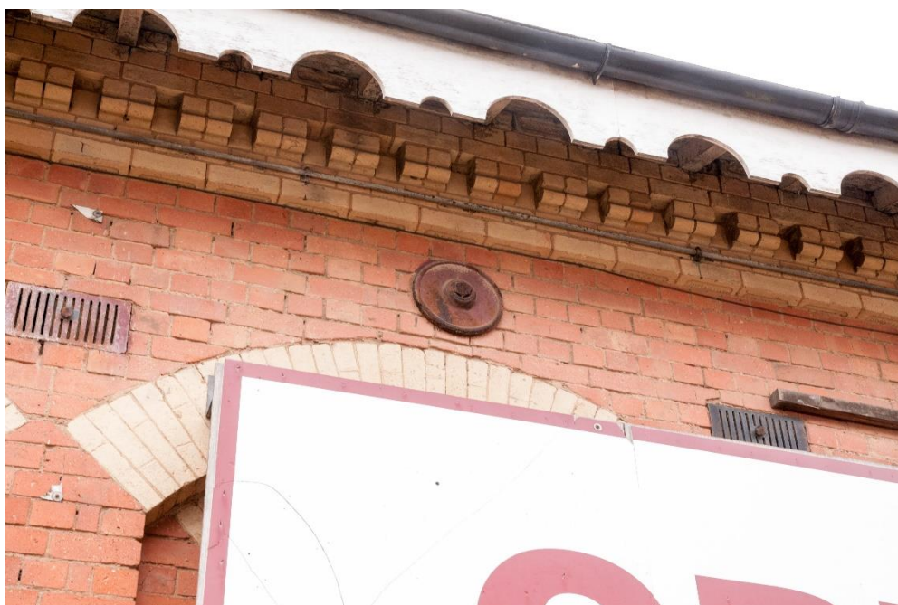
Figure 17 Detail of the ventilation grates and tie rod plate
