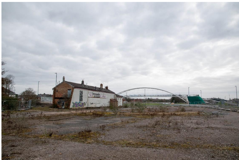
Figure 1 General view of the site across the former Chaddesden Sidings, looking east
