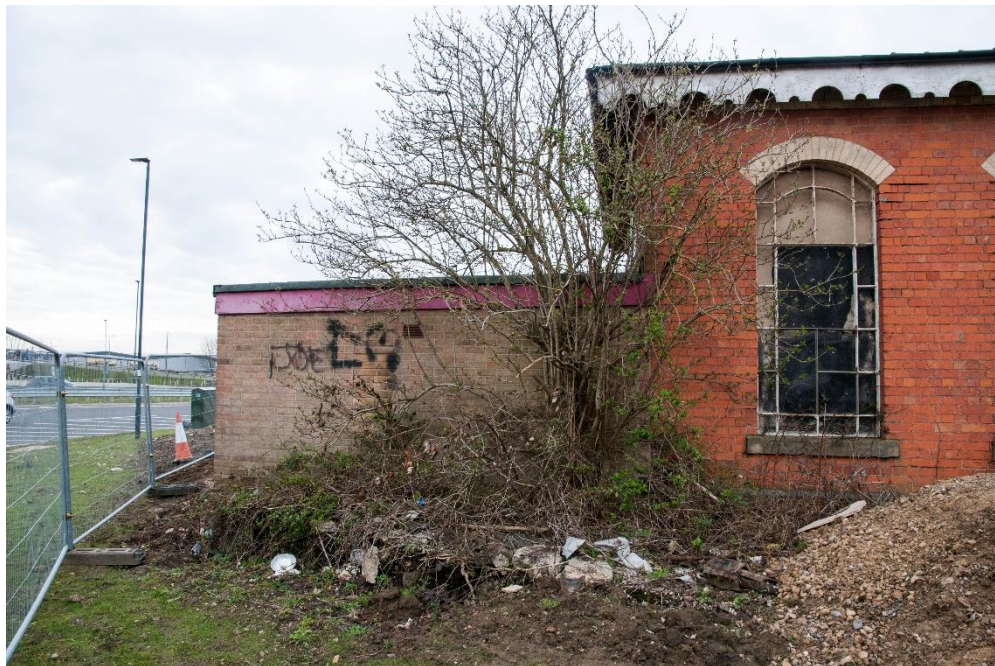
Figure 10 The modern extension, looking south
