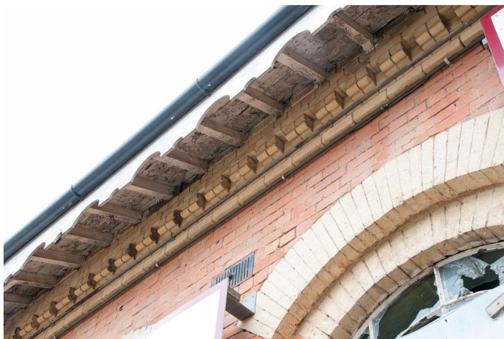
Figure 16 Detail of the cornice, dentils and projecting rafter ends
