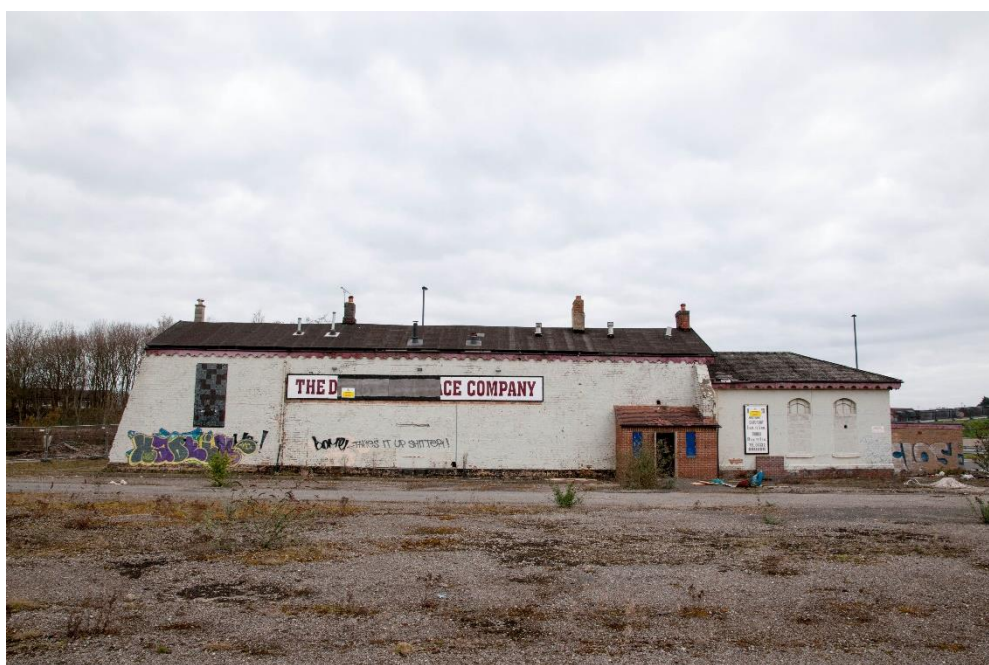
Figure 2 The south-facing elevation
