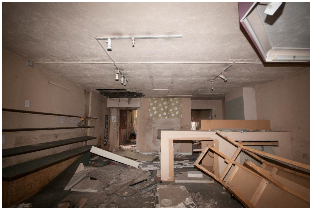
Figure 28 Room 2, looking east
