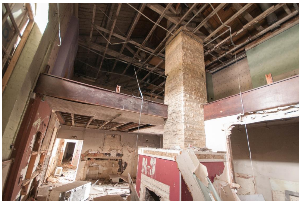
Figure 25 Room 1, looking east, showing inserted chimney and first floor platform
