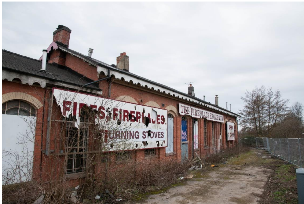
Figure 13 View of the north elevation, looking west
