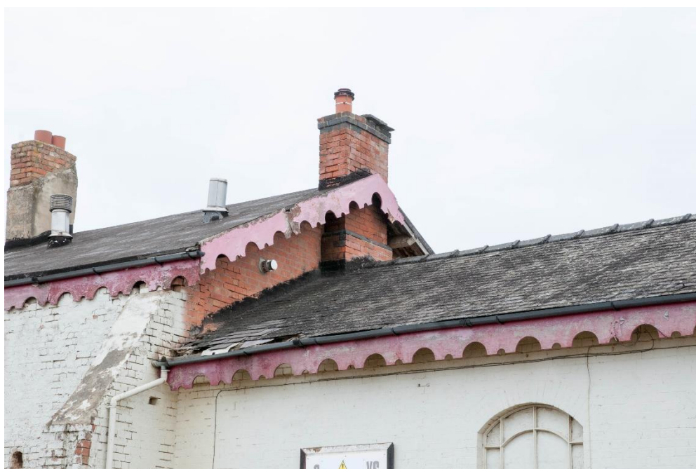
Figure 5 The east gable of the main building; note the remains of a former wall return
