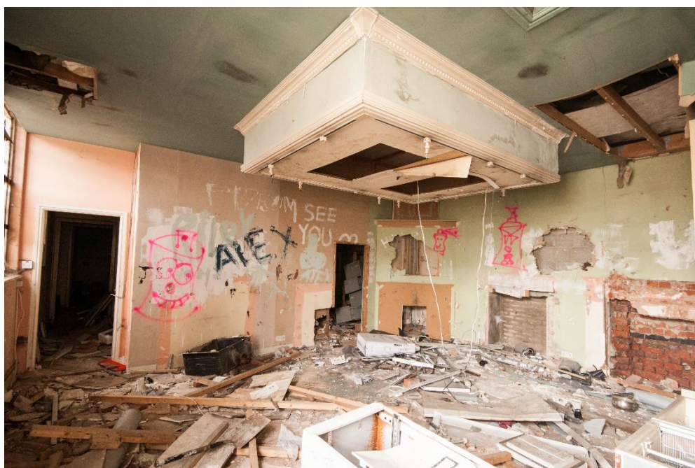
Figure 29 Room 3, looking east; showing lowered ceiling and modern alterations
