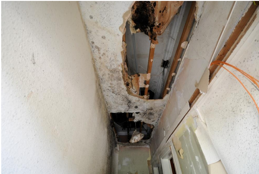
Figure 15 Detail of original ceiling over modern lowered ceiling
