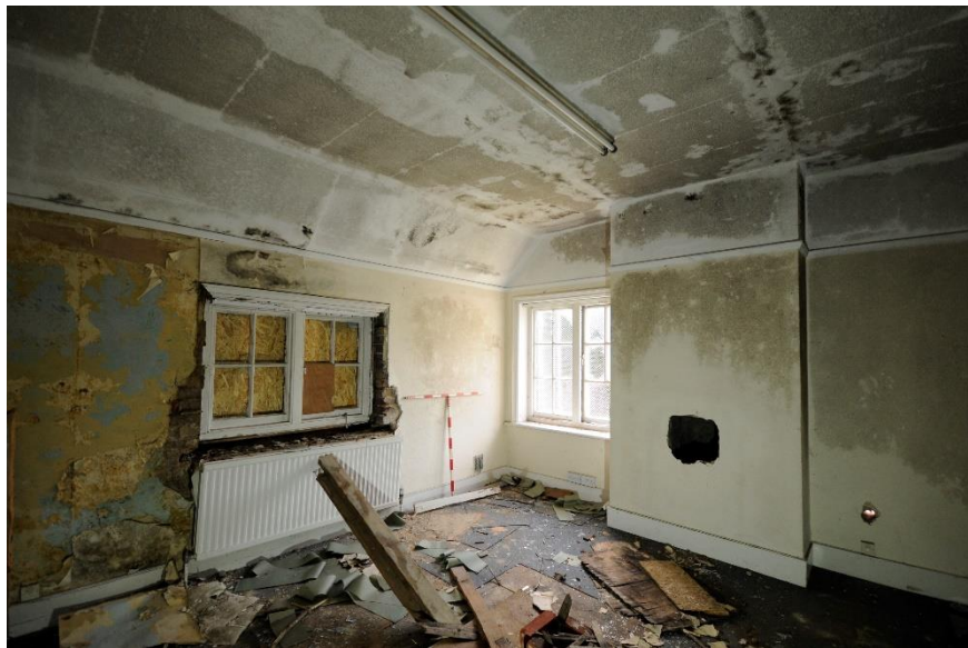
Figure 33 Room F2, looking south-east
