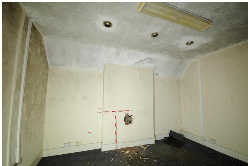
Figure 31 Room F1, looking east, showing blocked fire opening
