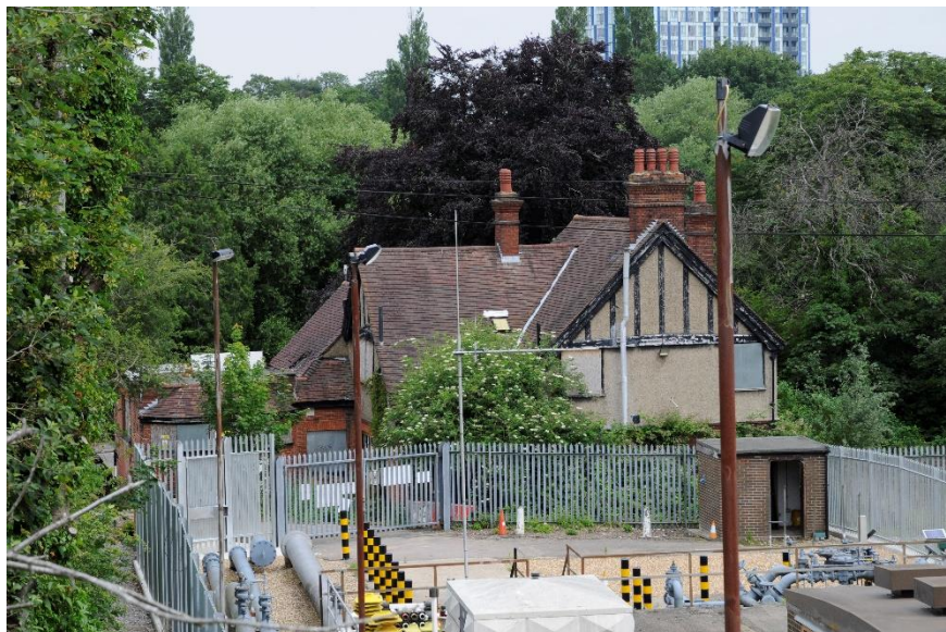
Figure 1 View of the building from the south, looking over the Cadent PRS station
