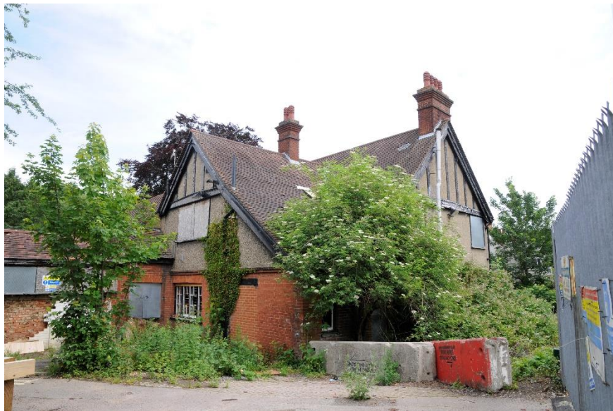
Figure 9 General view of the west and south elevations, looking north-east
