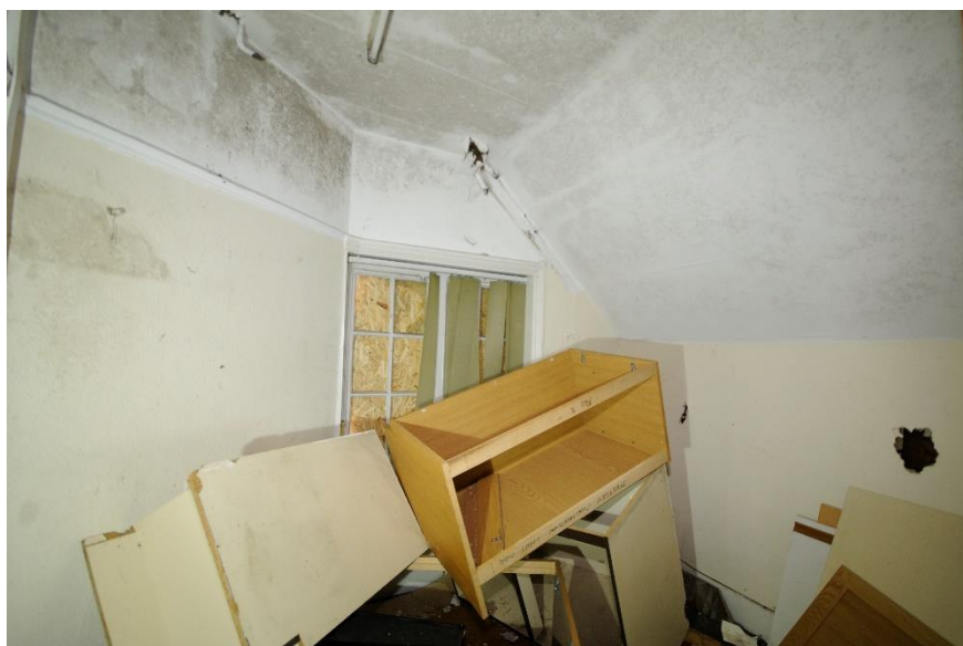
Figure 34 View of Room F4 showing angled wall
