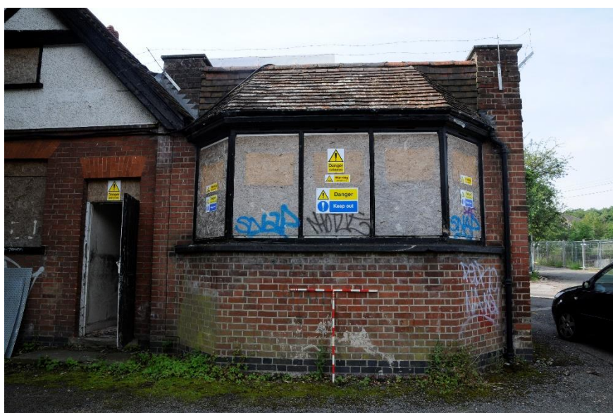
Figure 4 The north bay window of the single storey block
