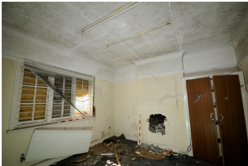
Figure 28 Room G9, looking south and showing blocked fireplace
