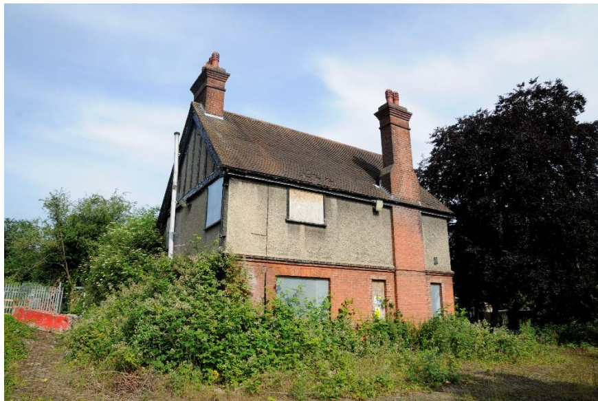
Figure 11 General view of the south and east elevations
