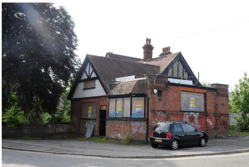
Figure 2 General view of the building from London Road, looking south-east
