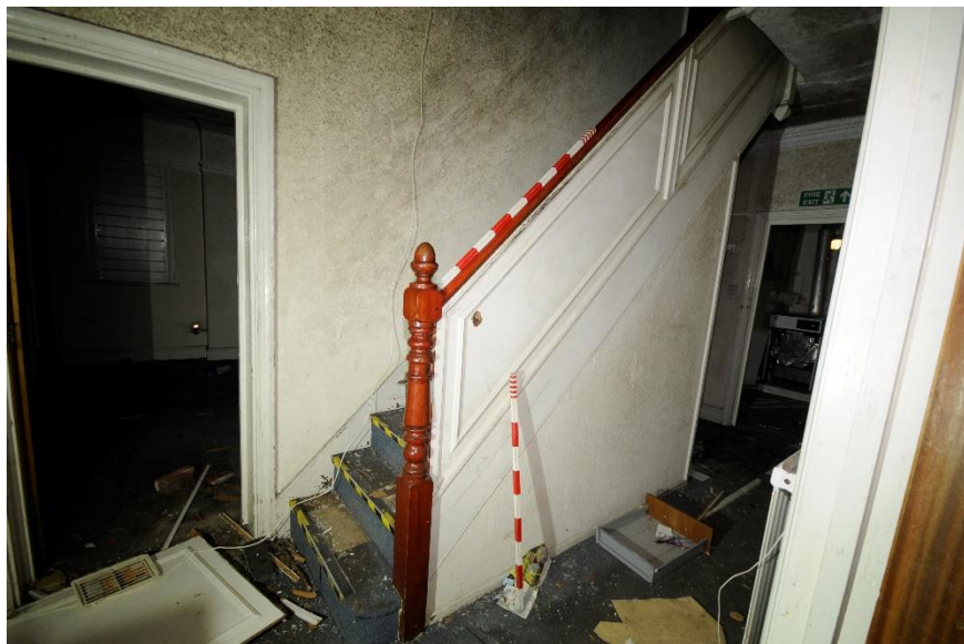
Figure 26 View of the stair
