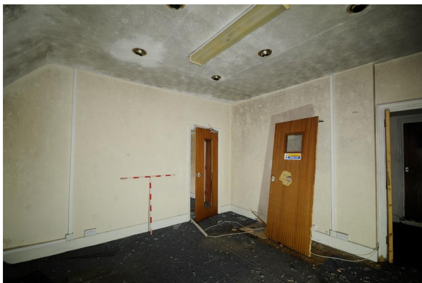
Figure 32 Room F1, looking south with doors to the landing and F2
