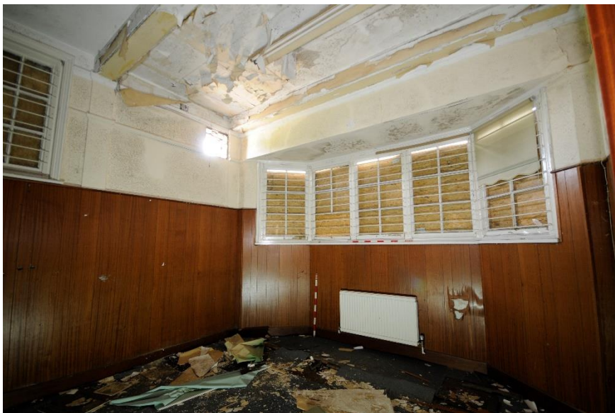
Figure 16 Room G1, looking north
