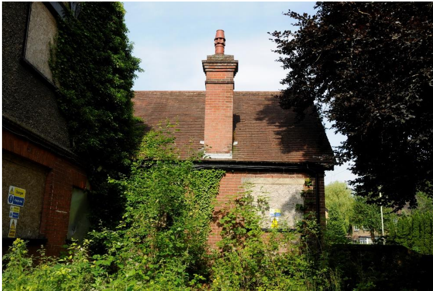
Figure 13 General view of the north elevation with the west block projecting forward
