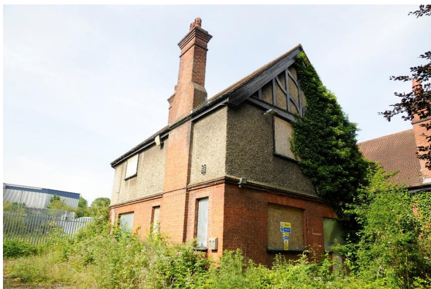
Figure 12 General view of the east and north elevations, looking south-west
