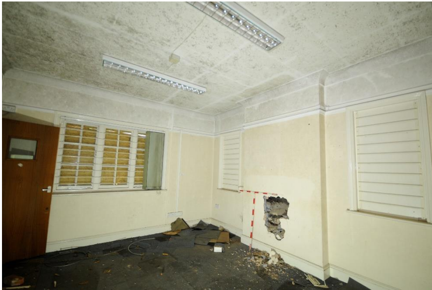
Figure 27 Room G8 showing blocked fireplace
