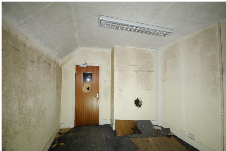
Figure 36 Room F5, looking east and showing chimney
