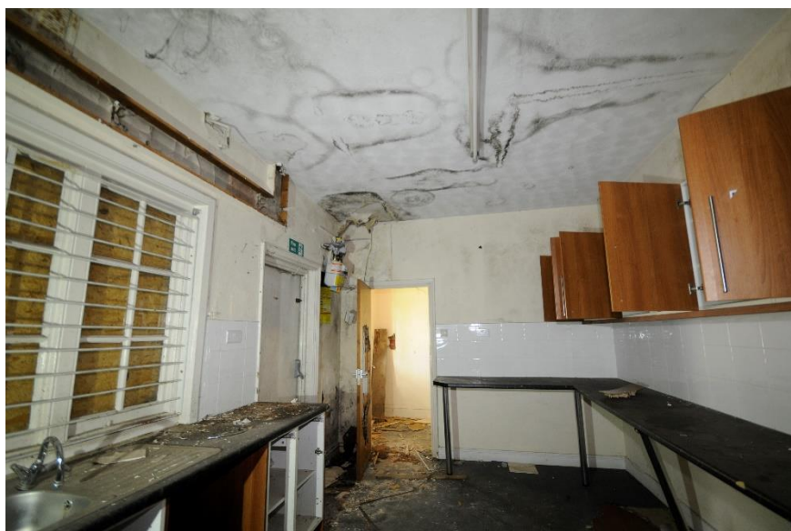
Figure 24 View of the kitchen, G7, looking west
