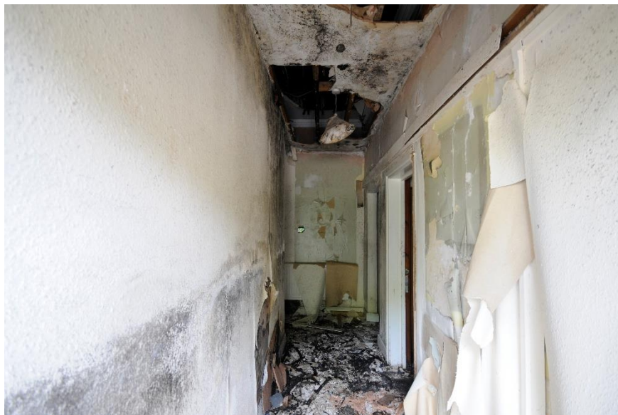
Figure 14 View of the corridor from entrance 1
