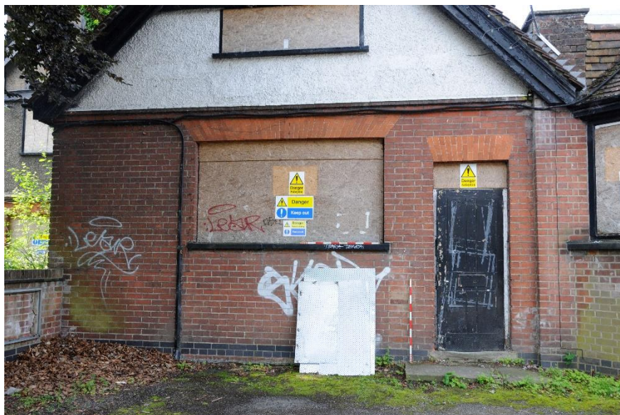
Figure 3 View of the north elevation and entrance 1
