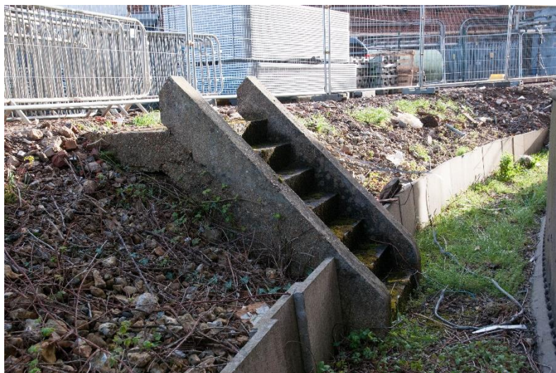
Figure 27 Example of the embankment stairs
