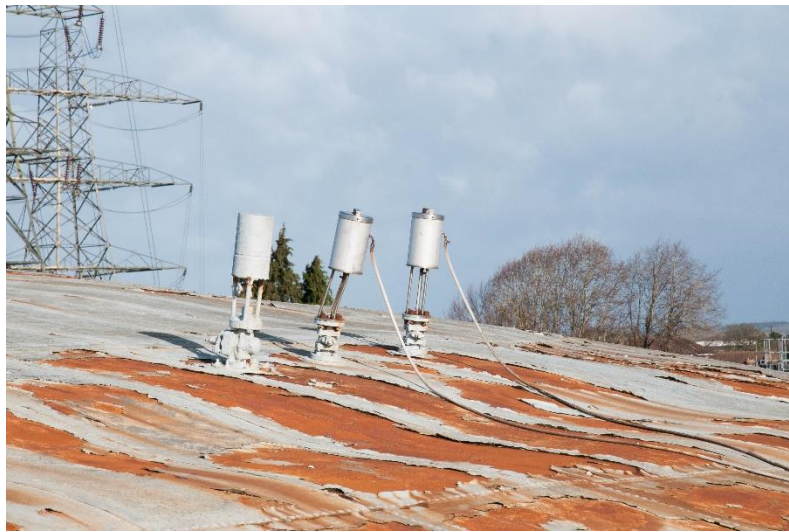
Figure 9 Detail of anti-freeze reservoirs
