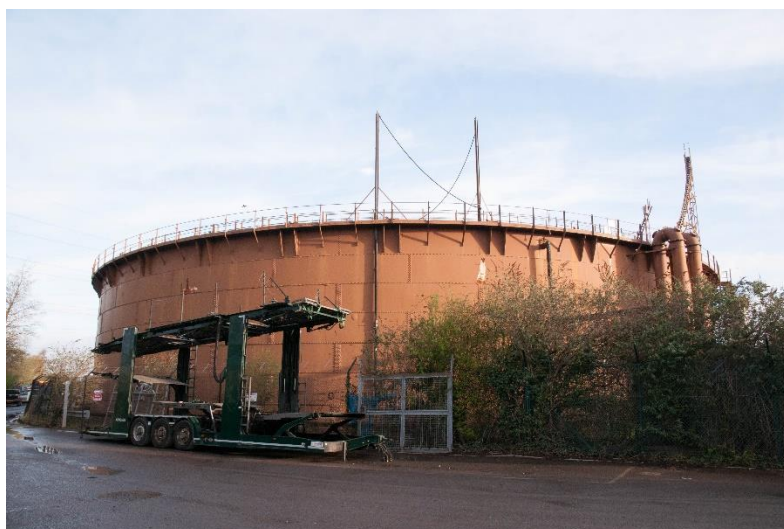
Figure 2 View of the gasholder from the west
