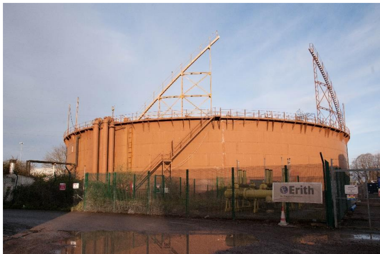
Figure 1 View of the gasholder from the east
