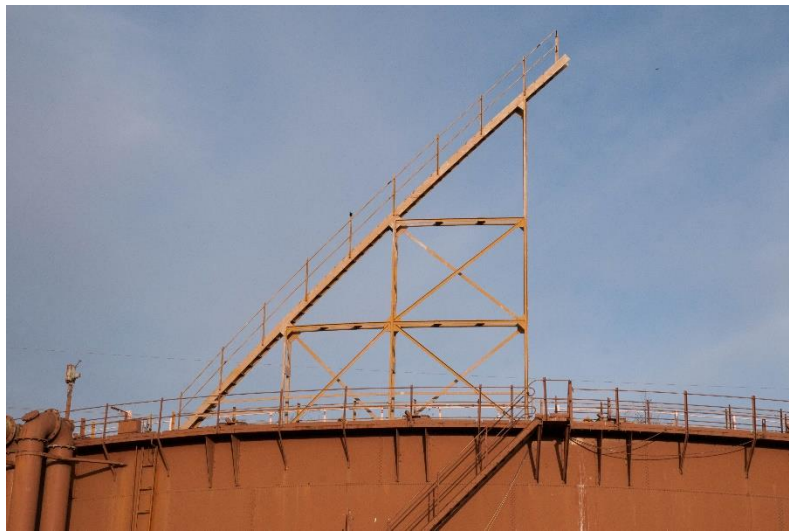
Figure 11 Example of the lift stairs
