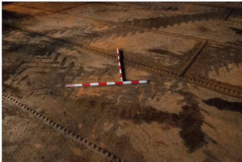
Figure 26 Detail of the riveted steel floor surface
