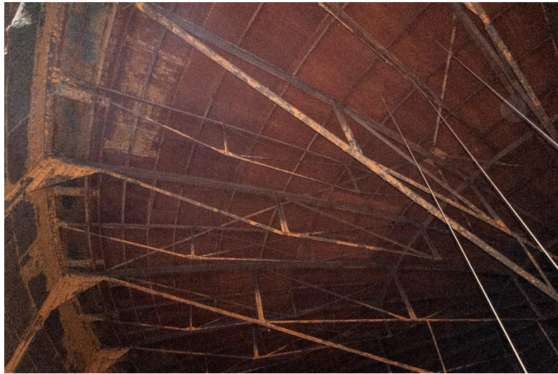
Figure 19 View of the crown frame trusses and join to vertical stiffeners
