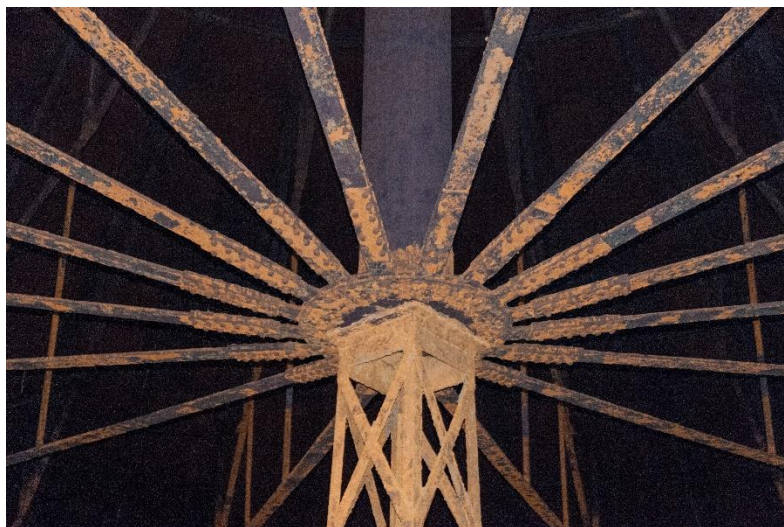
Figure 17 Detail of the crown frame support and lower anchor ring of the crown pin
