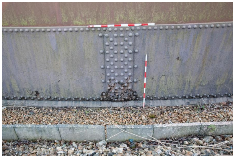
Figure 3 Detail of the tank construction at the base
