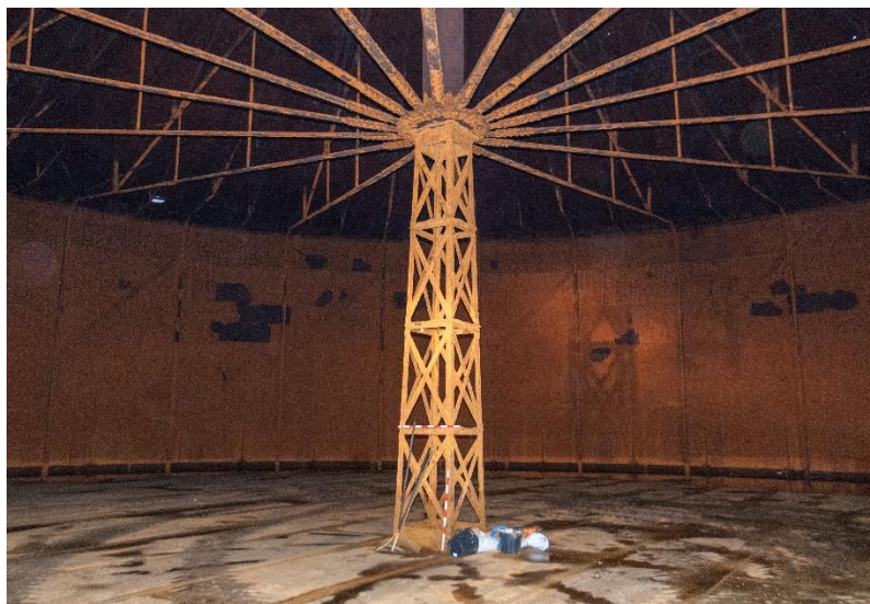
Figure 15 View of the crown support
