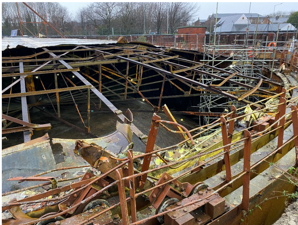
Figure 4: View inside Gasholder 1 showing trussed crown frame. Provided by demolitions contractor.
