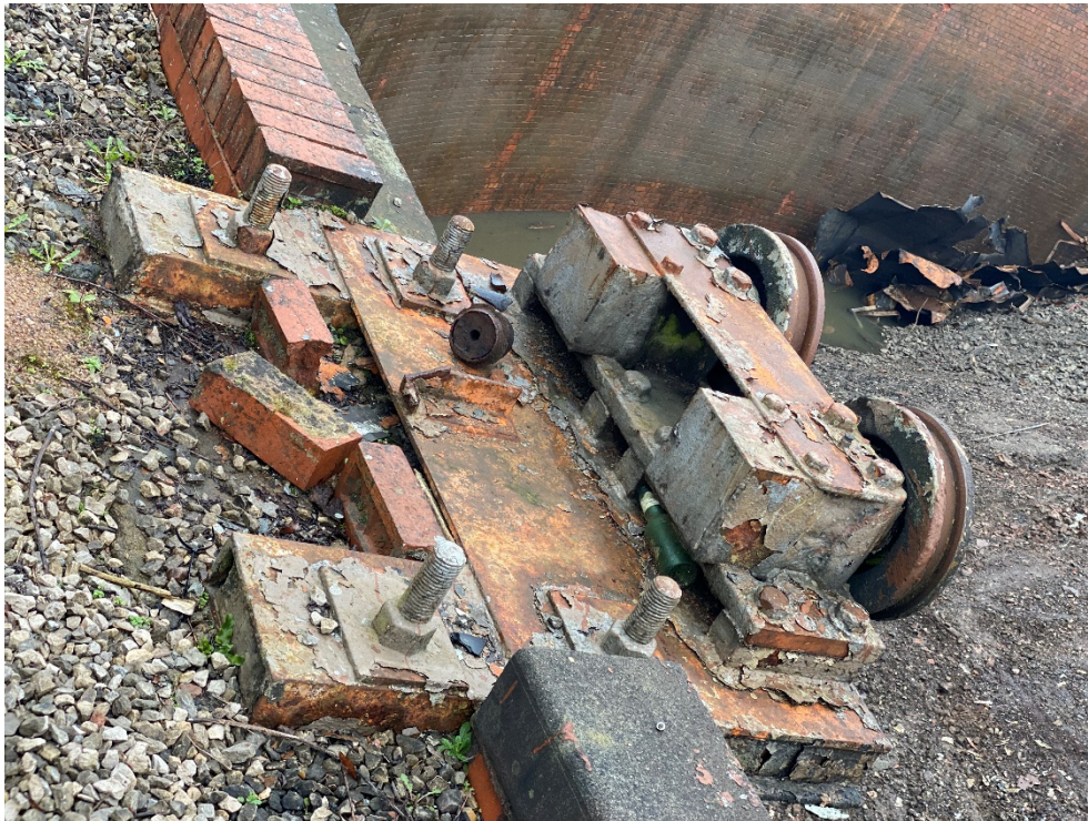
Figure 2: Extant Roller Carriage for Gasholder 1 projecting over the perimeter of the tank.
