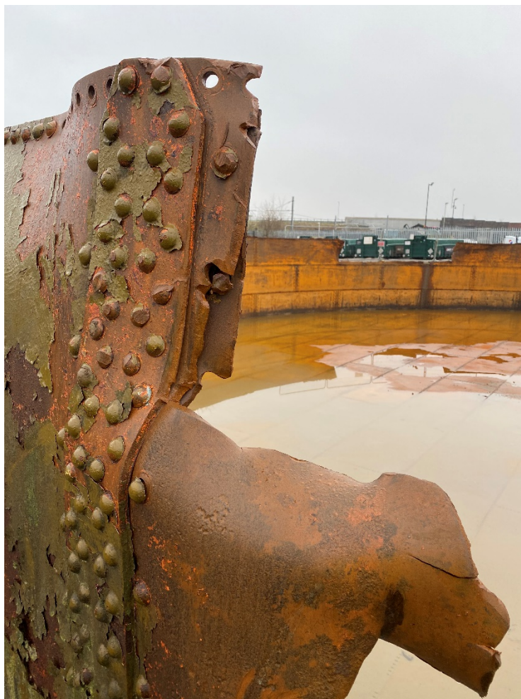
Figure 7: Riveted steel sheet construction of Gasholder 2.
