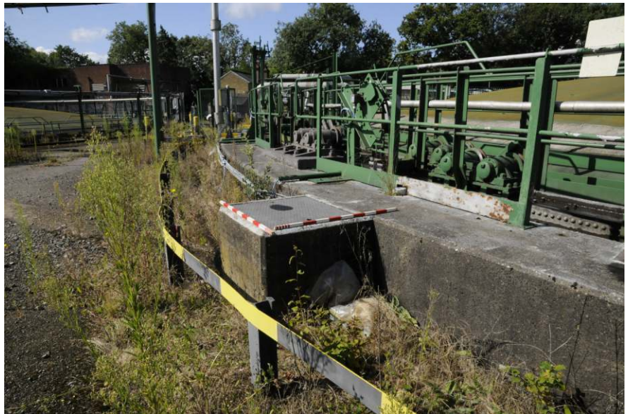
The raised tank kerb with access to well Fig 36
