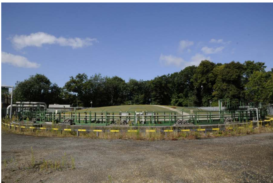
General view of Gasholder 3, looking west Fig 27
