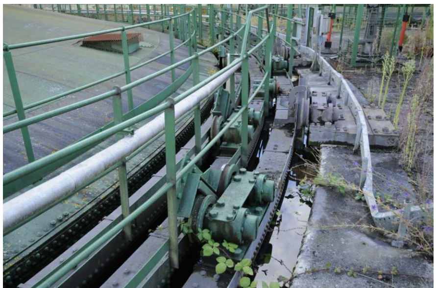
View of the tank kerb, lift grips and roller carriages Fig 11
