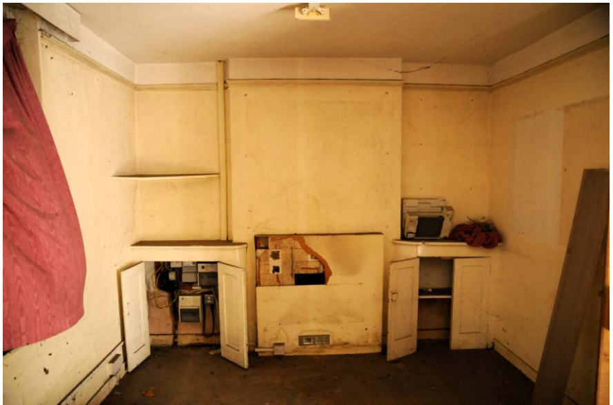
The ground floor living room with central tiled fireplace Fig 48
