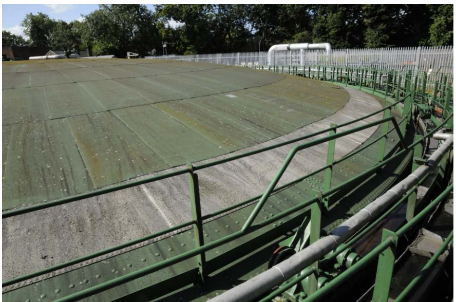
Pivoting steam pipe trays Fig 31
