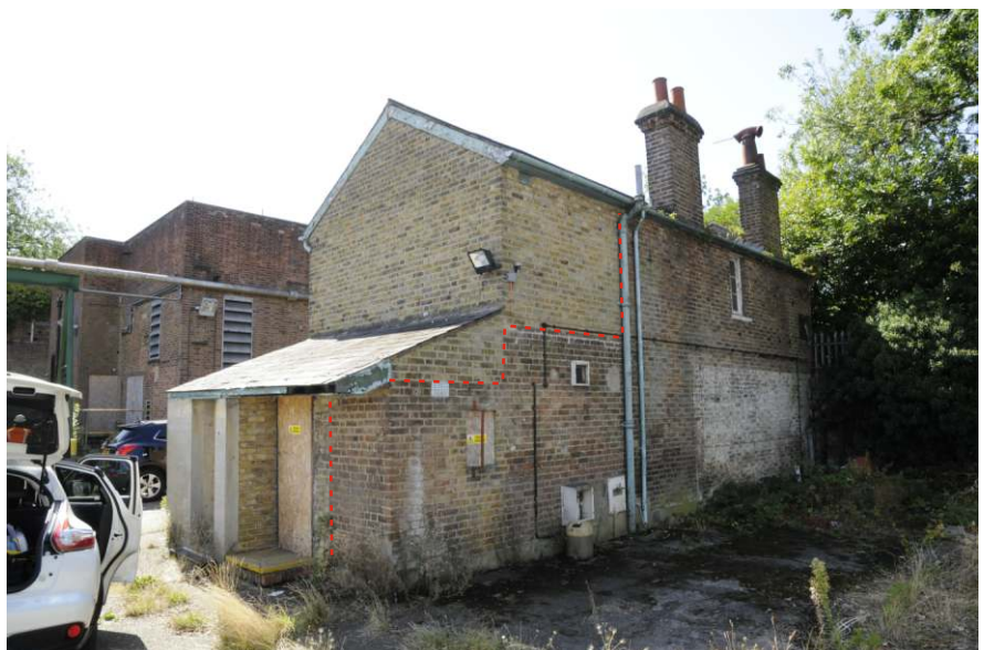
The north elevation; note joins denoting alteration of the building Fig 47
