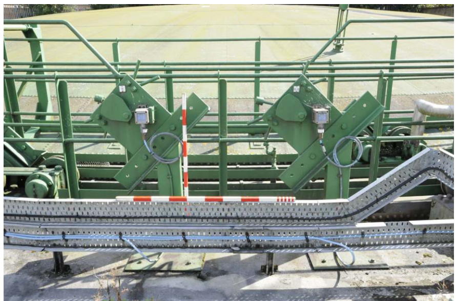
Detail of hammer switch / maglocks Fig 14
