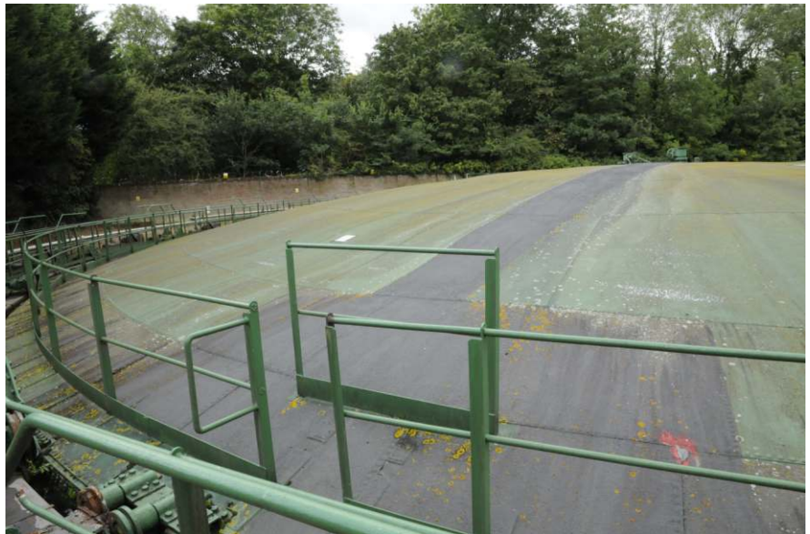
View of the crown, showing access and walkway to centre plate Fig 9
