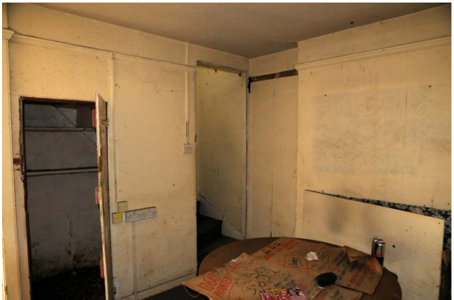
Understairs cupboard with stairs to first floor Fig 49
