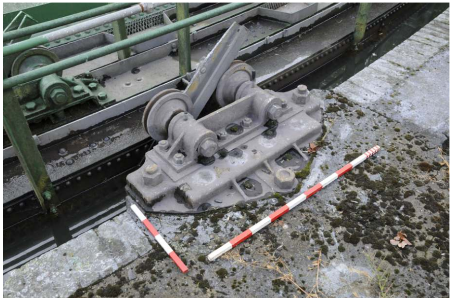
Example of the roller carriages, showing the tank kerb Fig 25
