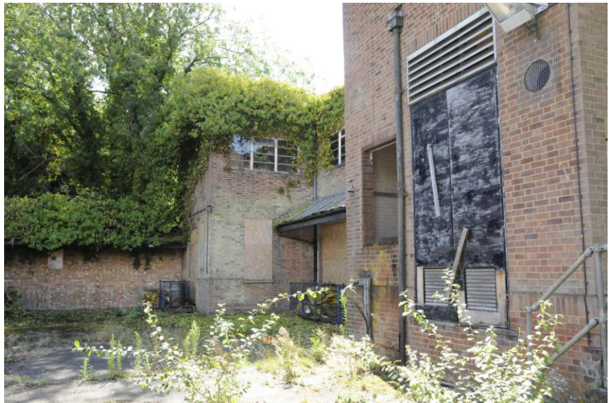
General view of the south elevation of the Booster House Fig 42
