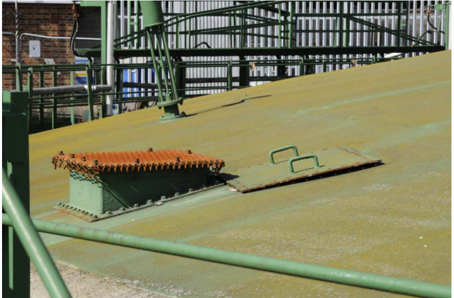
Detail of crown manhole Fig 33
