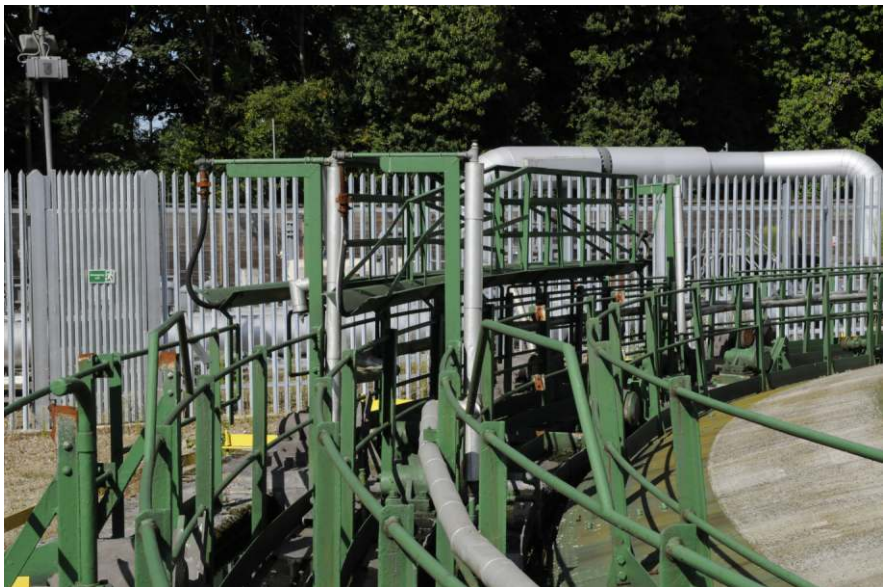
Pivoting steam pipe trays Fig 31
