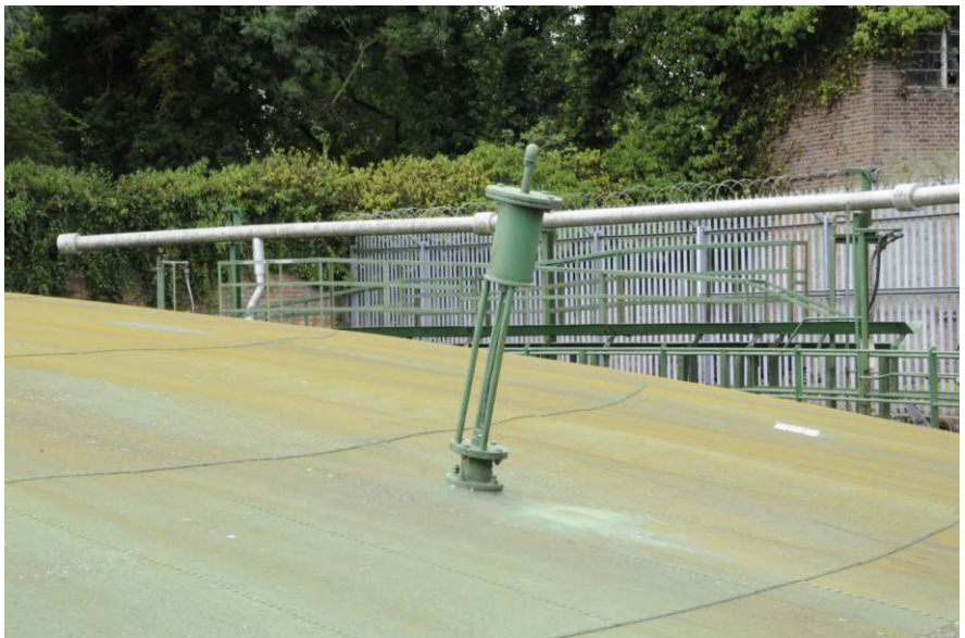
Detail of crown vent Fig 22
