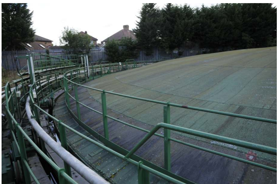
General view of the crown, looking east Fig 8
