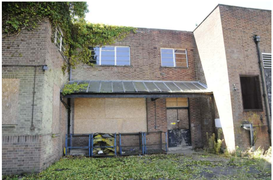
Entrance to the office area of the Booster House Fig 43
