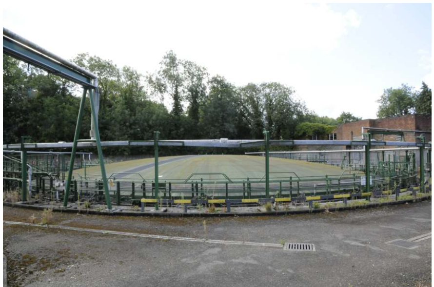
General view of Gasholder 2, looking south-west Fig 18
