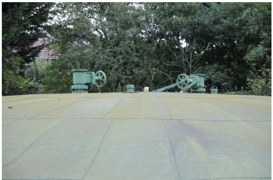
Valves at the crown apex Fig 10
