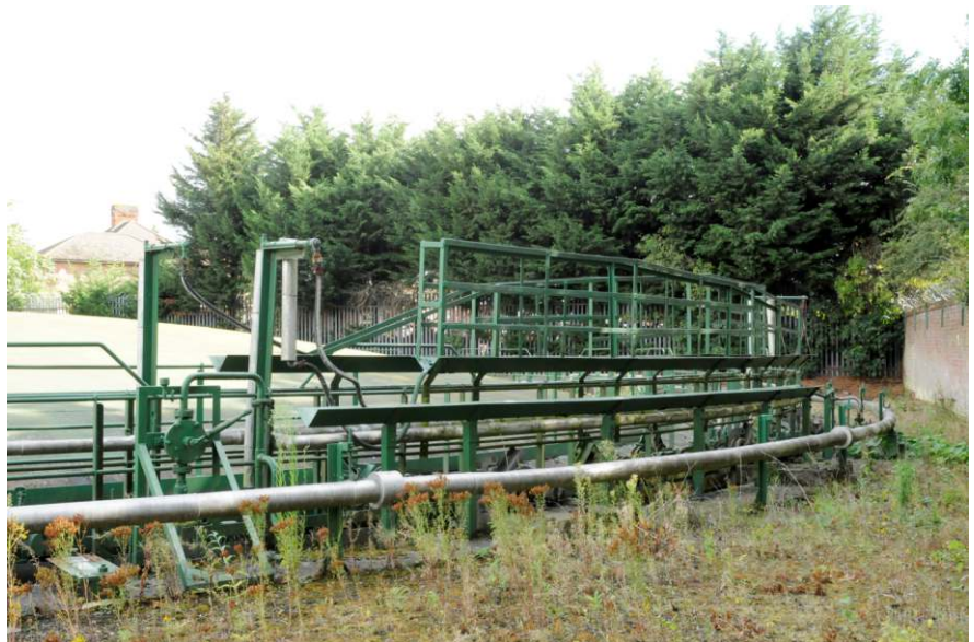
Pivoting steam pipe trays at the south side of the gasholder Fig 13
