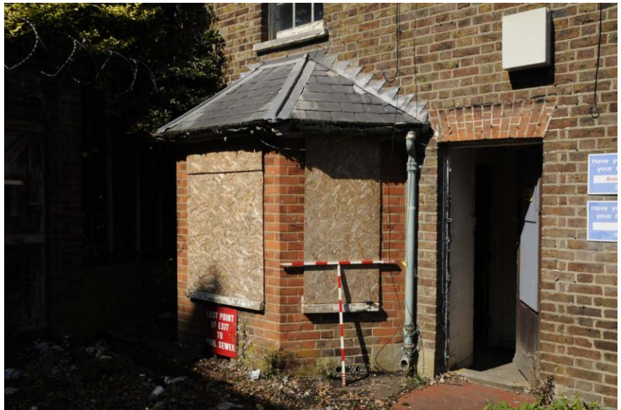
The main entrance with adjacent modern bay window Fig 45
