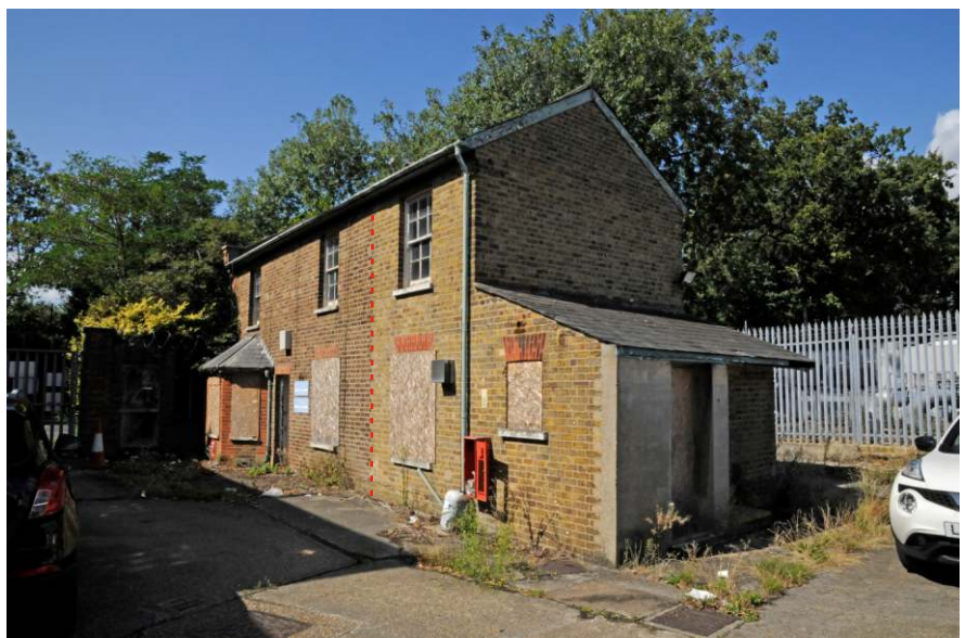
The south and east elevations of the Cottage; note vertical change in fabric Fig 44
