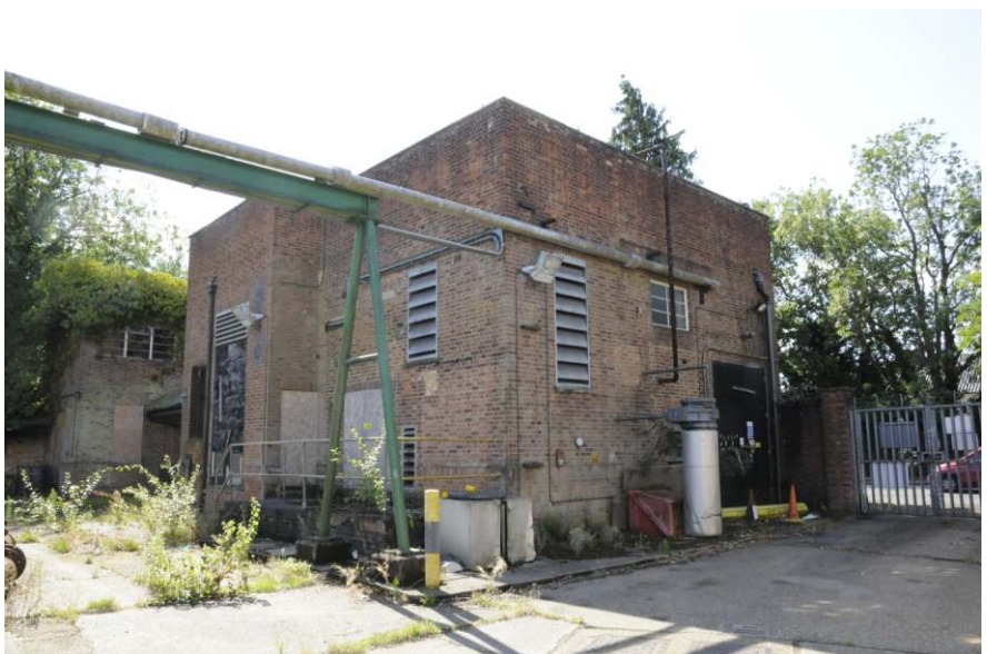
The Booster House, looking south, showing lagged pipe from Gasholder 2 Fig 41
