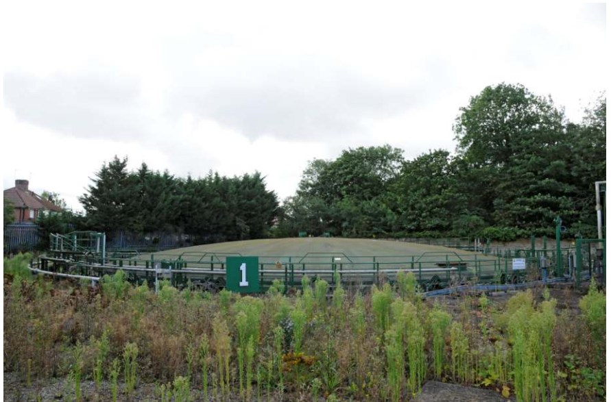
General view of Gasholder 1, looking south-east Fig 6
