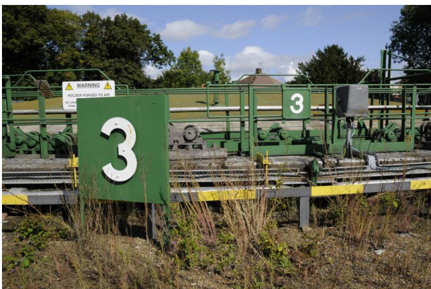
View of signage, crash barrier and tank handrails Fig 28
