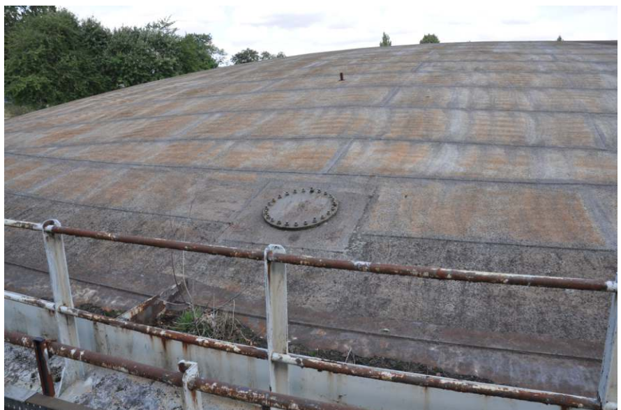
General view of the crown with circular manhole Fig 22
