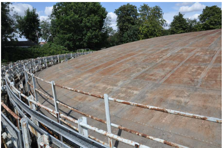
General view of the crown, looking north-west Fig 10
