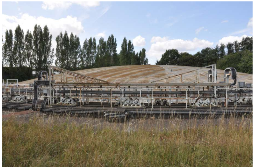
View of the gasholder, crown and cable trays, looking south-west Fig 18
