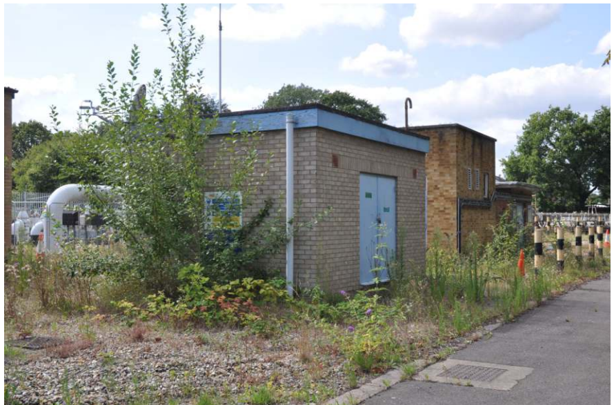
General view of electrical substation at site entrance Fig 30
