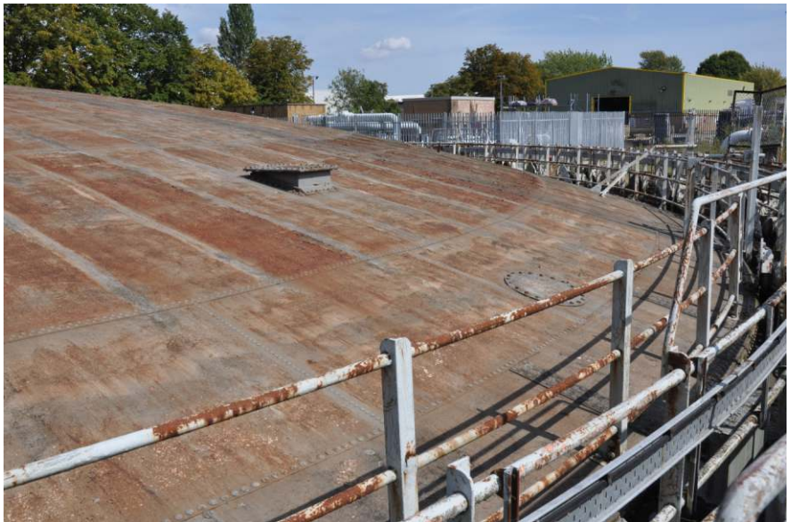
View of the crown with manholes, looking north-east Fig 11
