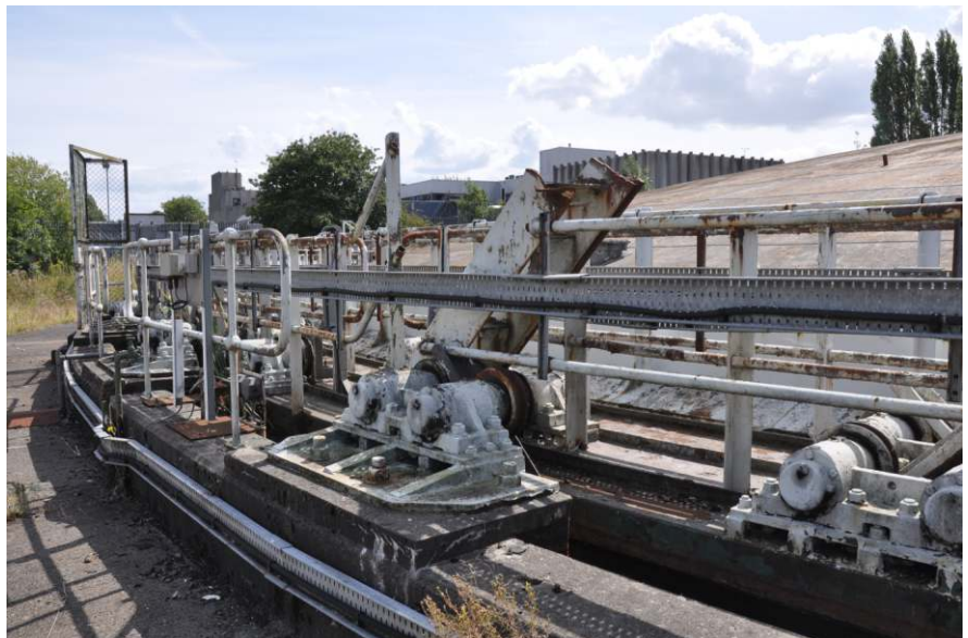
The roller carriages; also showing truncated spiral stair Fig 27
