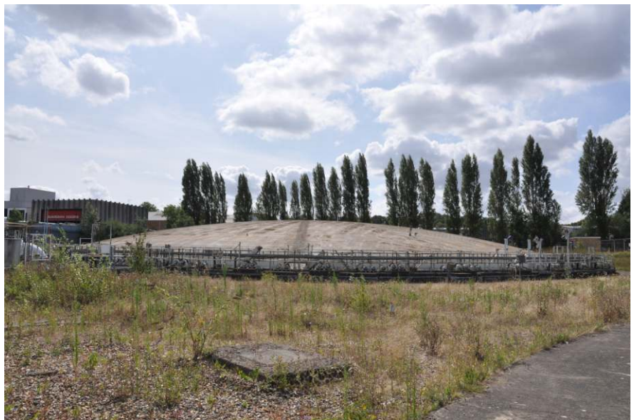
General view of Gasholder 2, looking south Fig 17
