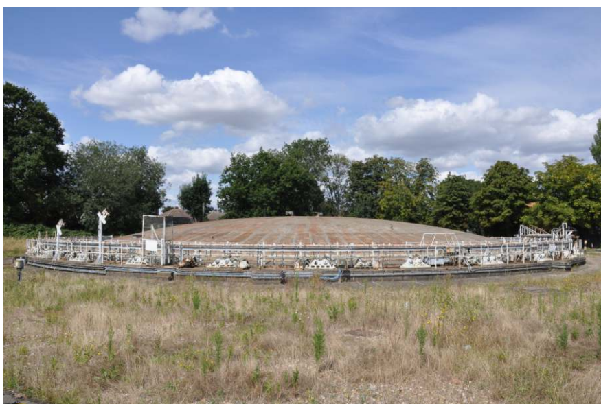
General view of Gasholder 1, looking north-west Fig 5
