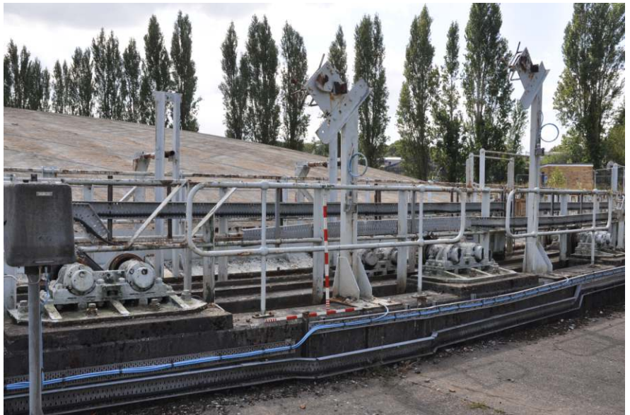
Elevated maglock / hammer switches and lift knock-off arms Fig 23
