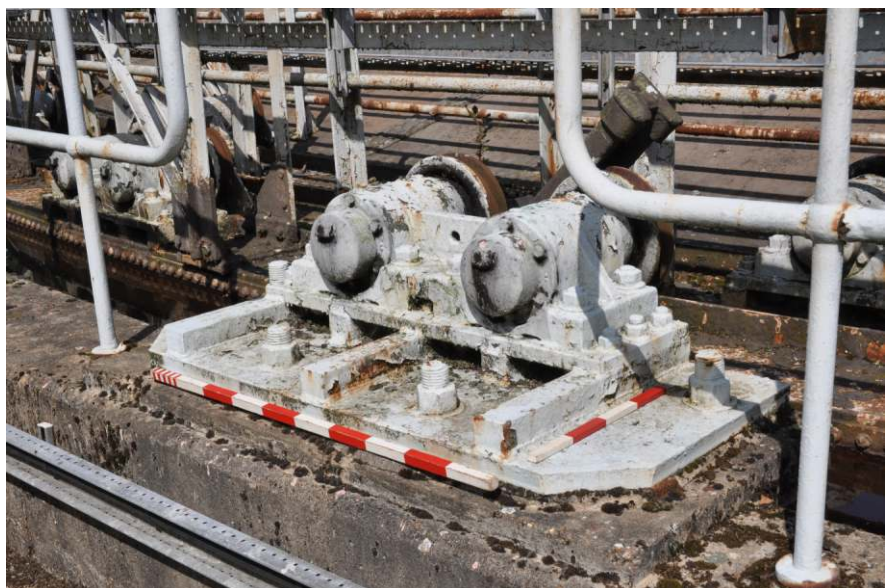
Example of the tank roller carriages Fig 16
