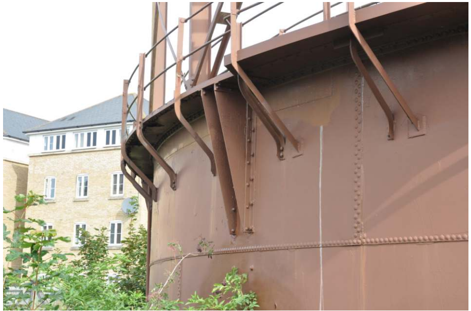
Detail of the tank construction Fig 8
