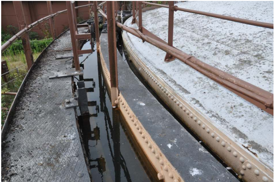
View of the walkway, lift and grips Fig 12
