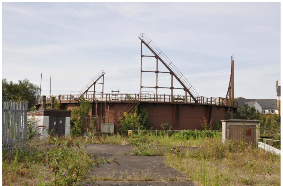
General view of the Gasholder 108, looking south-west Fig 18
