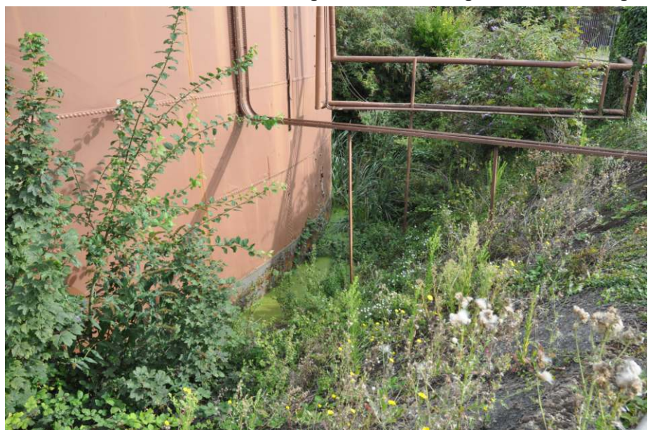
View of the gasholder moat Fig 7
