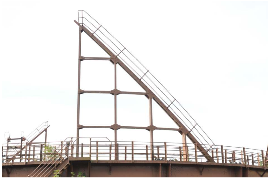
Example of the spiral stairs Fig 20
