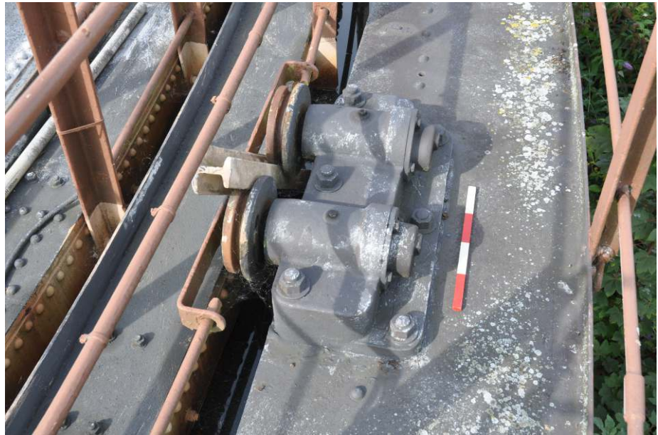
Example of the tank roller carriages Fig 27
