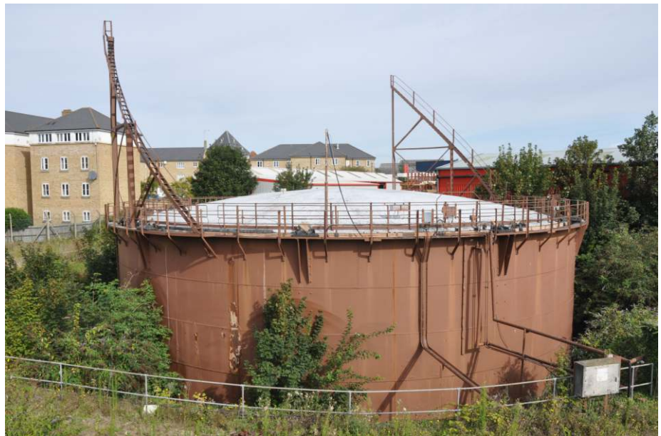
General view of Gasholder 107, looking north Fig 5
