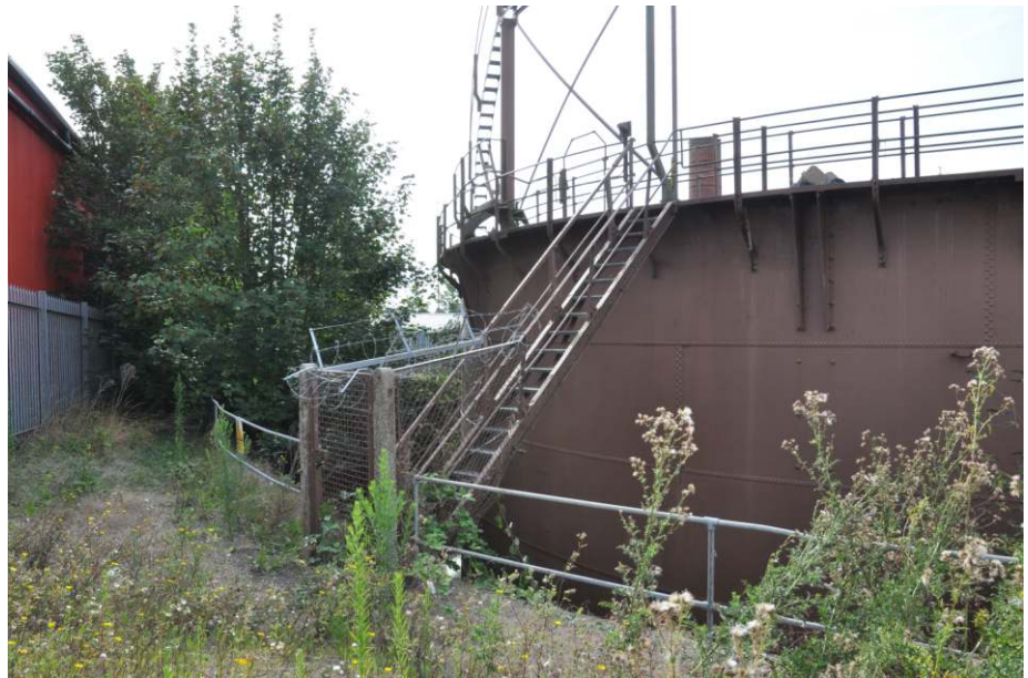
The stair to the tank walkway Fig 9
