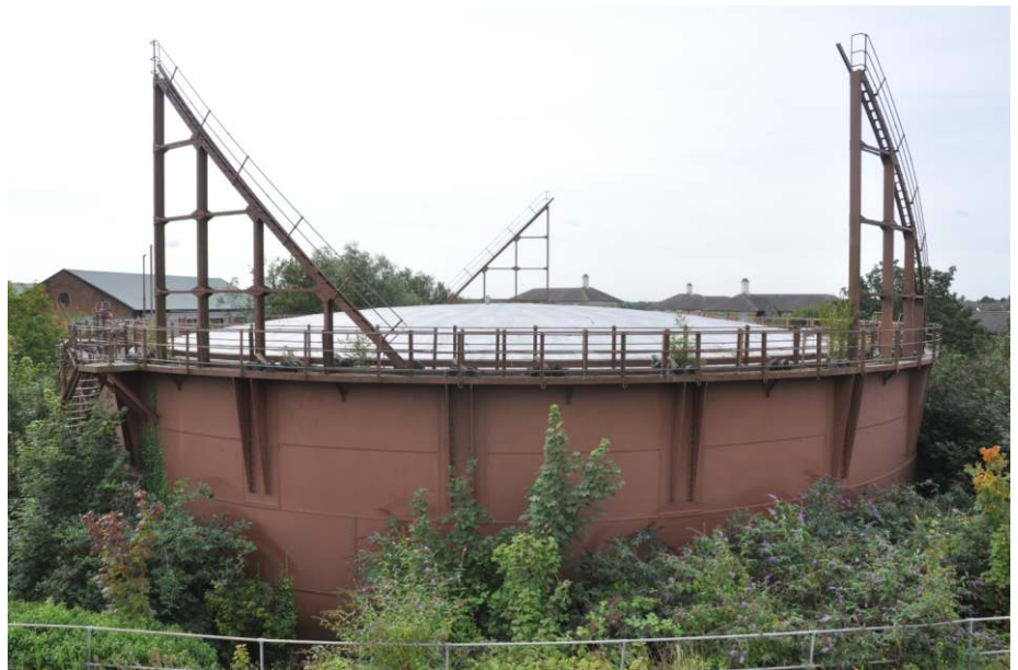
General view of Gasholder 108, looking south Fig 17
