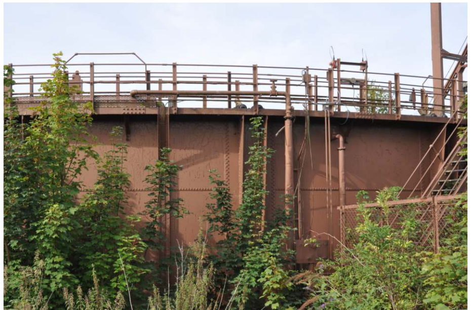
View of the tank walkway with handrails and overflow pipes Fig 21
