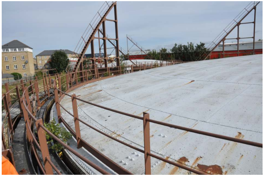
View of the crown, looking south Fig 23
