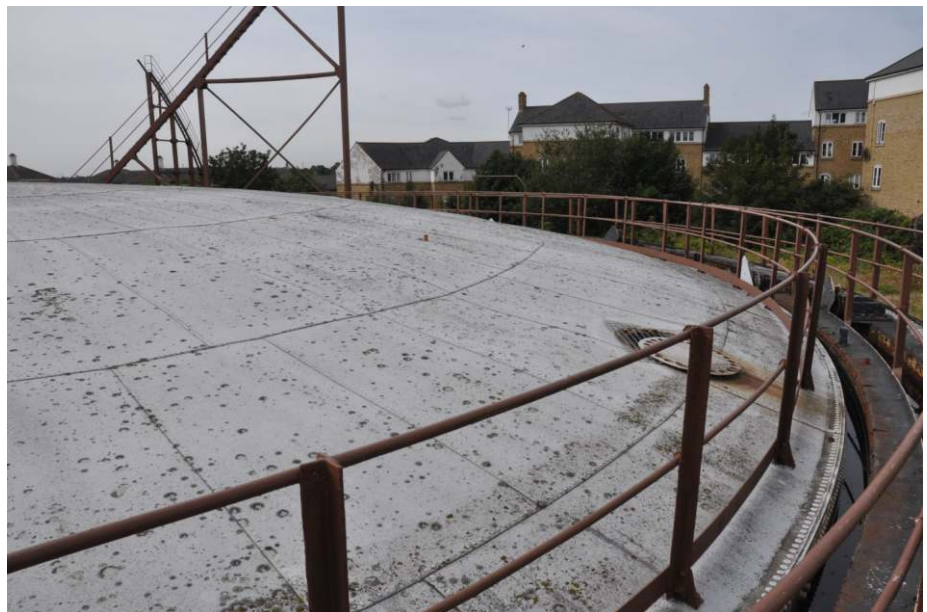
View of the crown, looking south-west Fig 10
