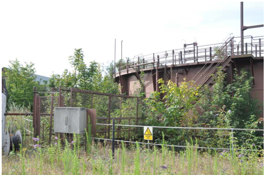
View of the tank stair Fig 22
