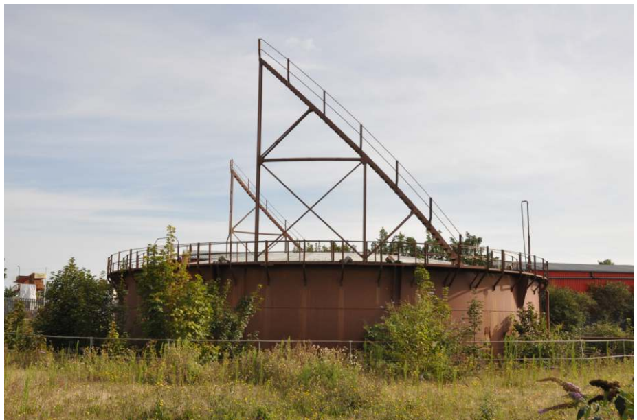
General view of the gasholder, looking north-east Fig 6
