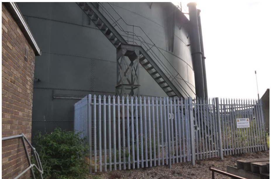
The tank stair Fig 10
