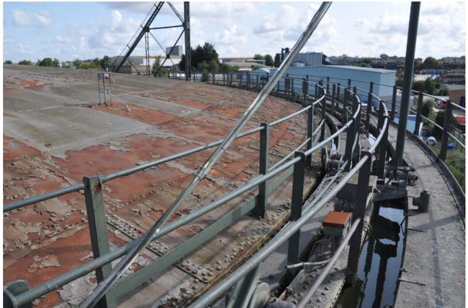
Detail of the tank walkway, lift grips and hand-rails Fig 12
