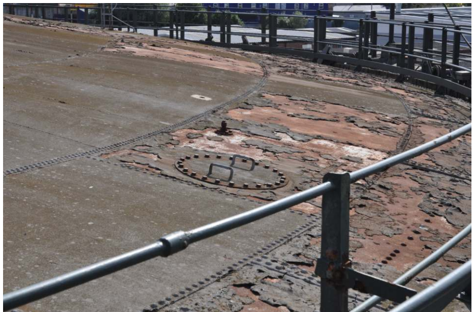
Detail of the crown with manhole Fig 13
