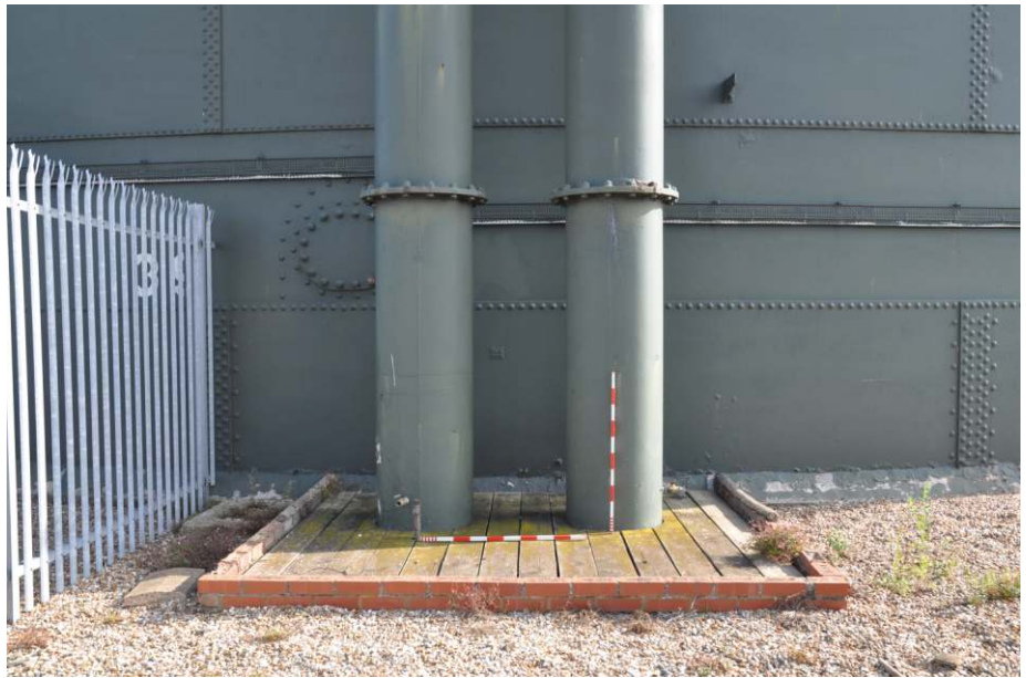
The inlet / outlet pipes and dry-well, with adjacent manhole Fig 8
