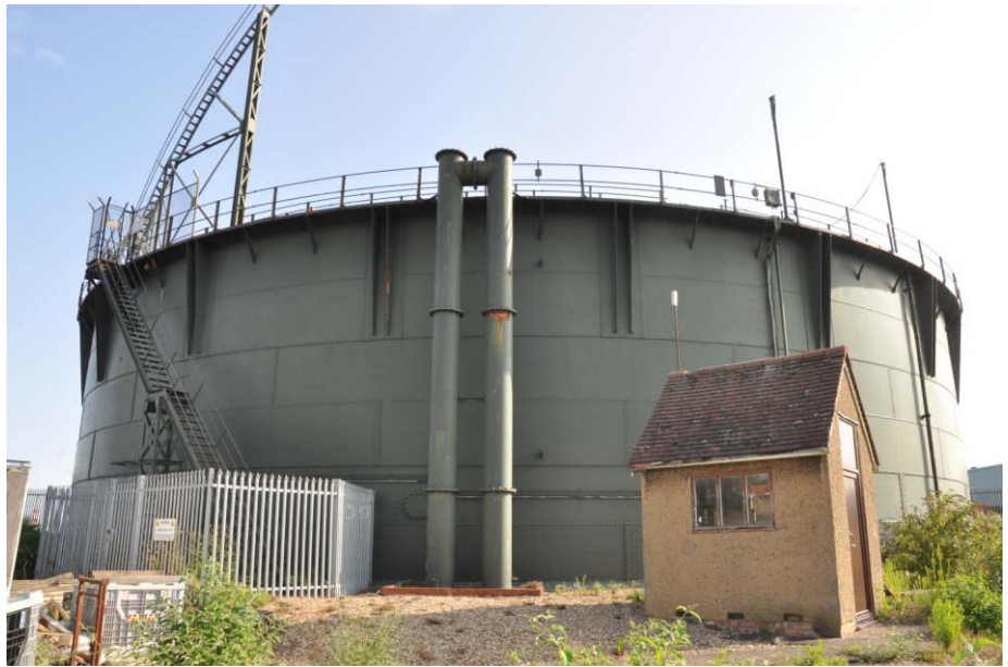
General view of the gasholder, looking north-west Fig 5
