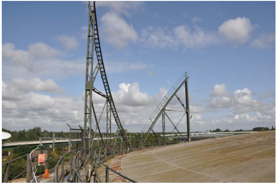
General view of the crown and spiral stairs, looking south-west Fig 11
