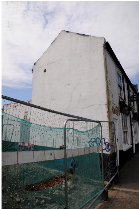
Figure 5 The east-facing gable elevation
