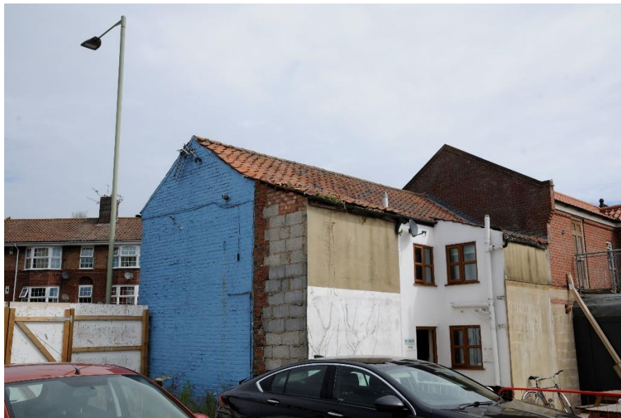
Figure 23 The west and south elevations, looking north-east
