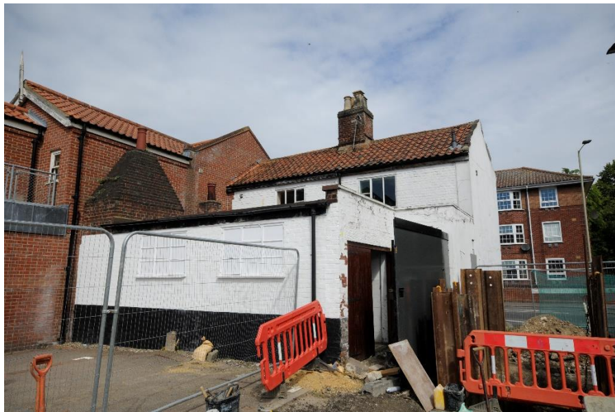
Figure 6 View of No. 77 and 79 from the south, showing the modern extensions
