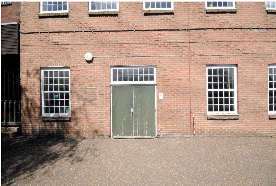
Figure 35 Detail of ground floor door and windows
