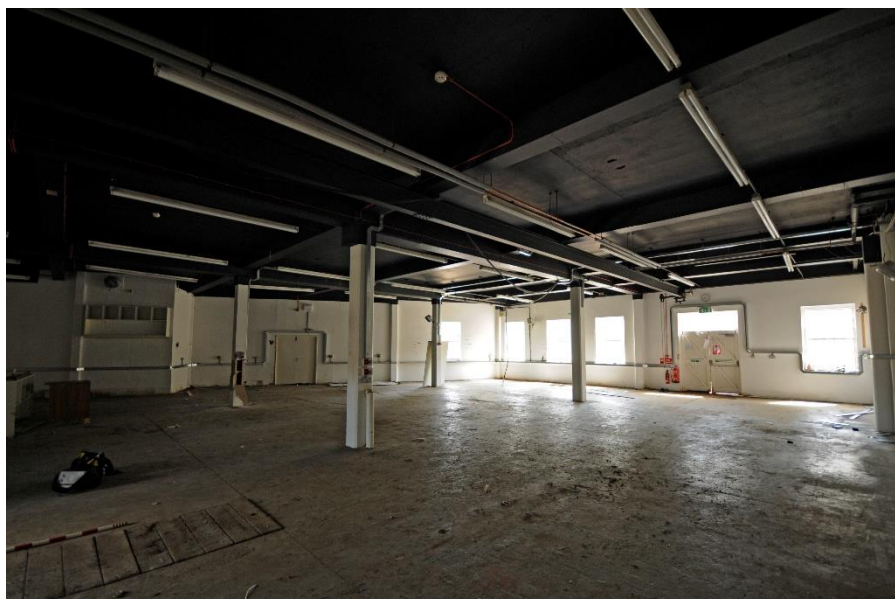
Figure 38 The ground floor space, looking south-east
