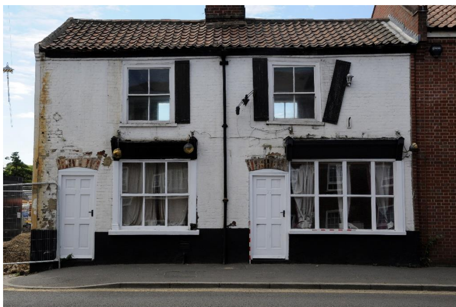
Figure 2 The north-facing elevation of No. 77 and 79
