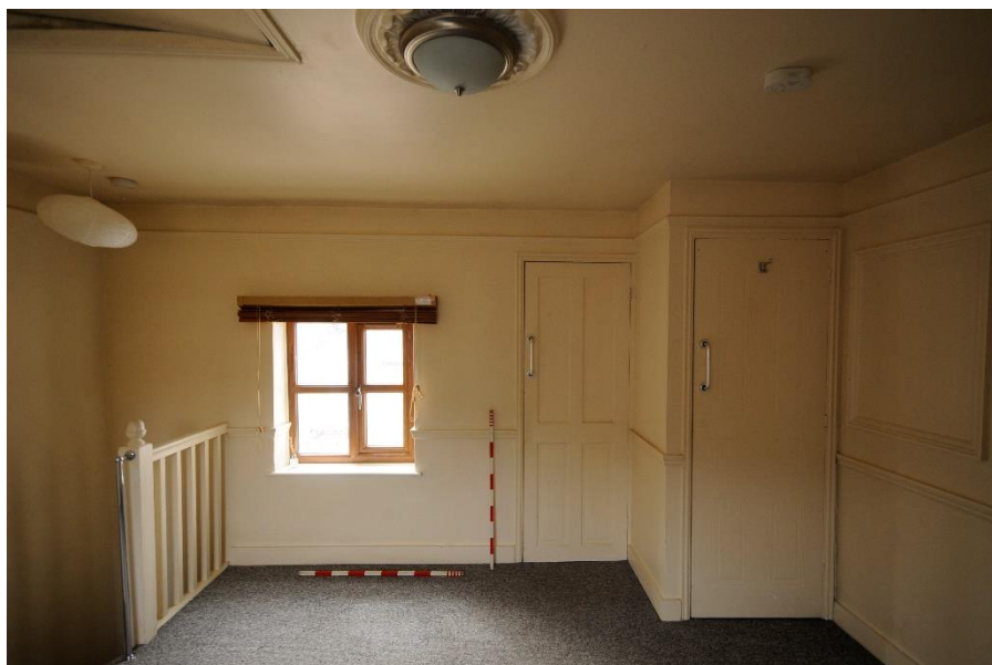
Figure 30 Room F1, looking south
