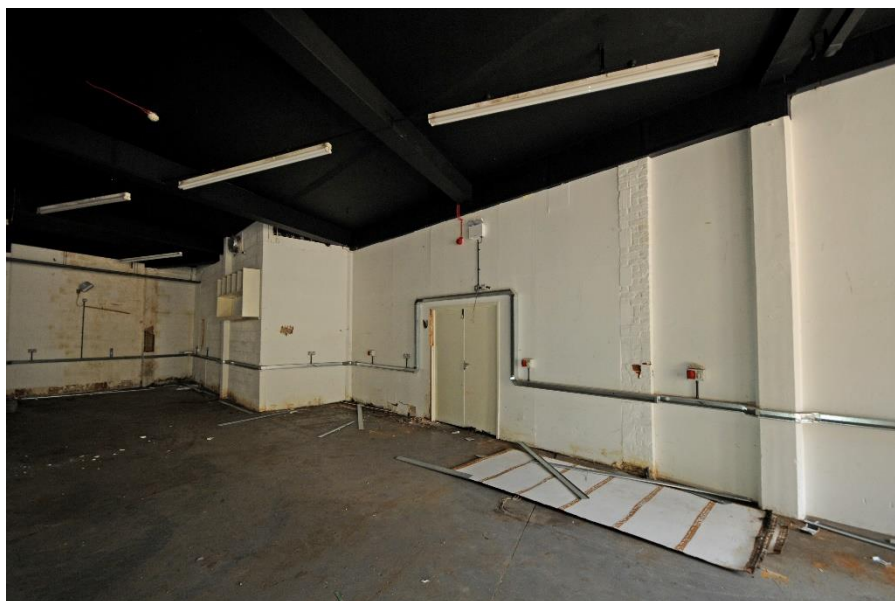
Figure 40 The eastern wall with truncated remains of a former return wall visible
