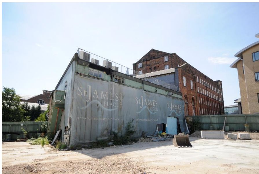
Figure 36 The southern side of the Annex
