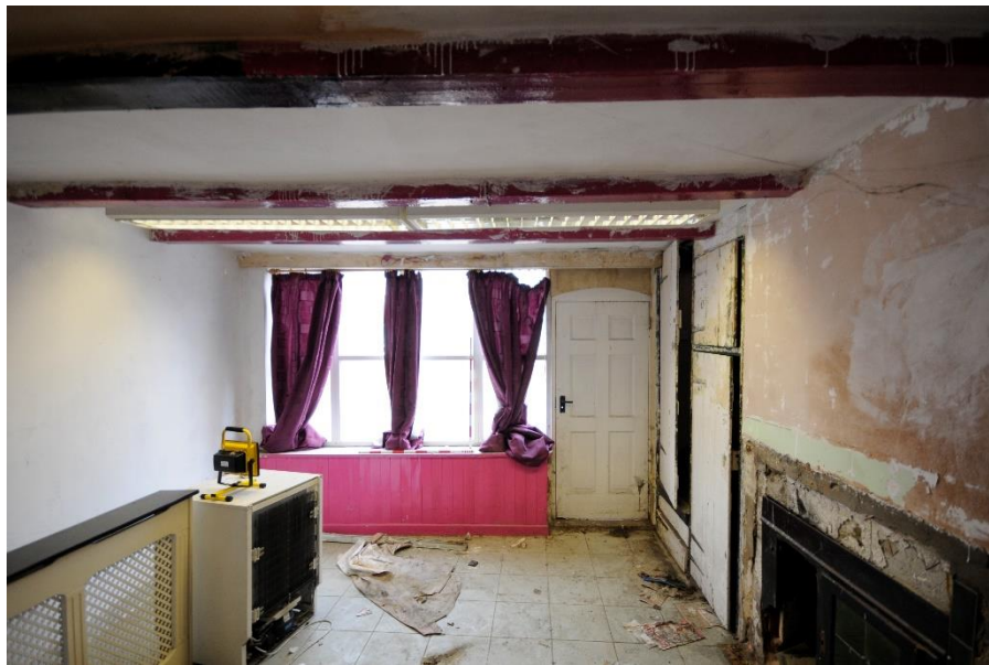
Figure 7 Room G1, looking north
