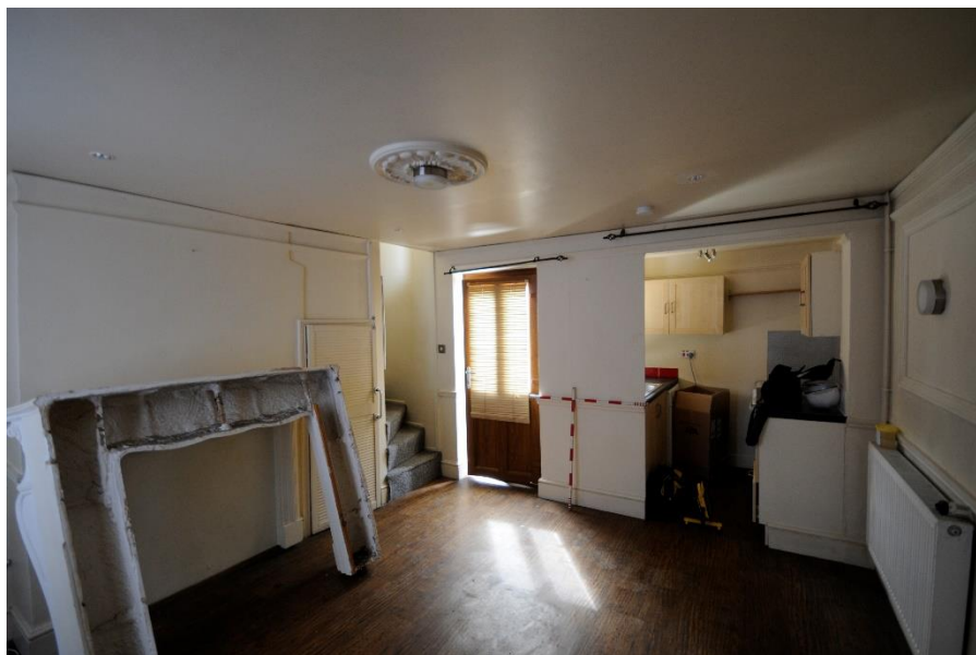
Figure 27 Room G1, looking south-east
