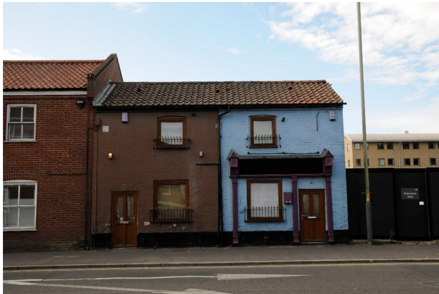
Figure 19 The north-facing elevation of No. 67 and 69
