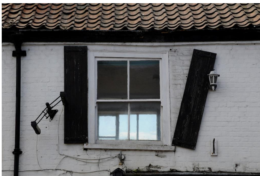
Figure 4 The first floor window to No. 77 with 'shutters'
