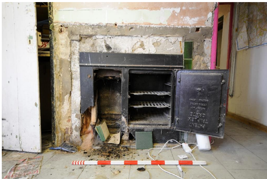
Figure 10 Detail of the fireplace
