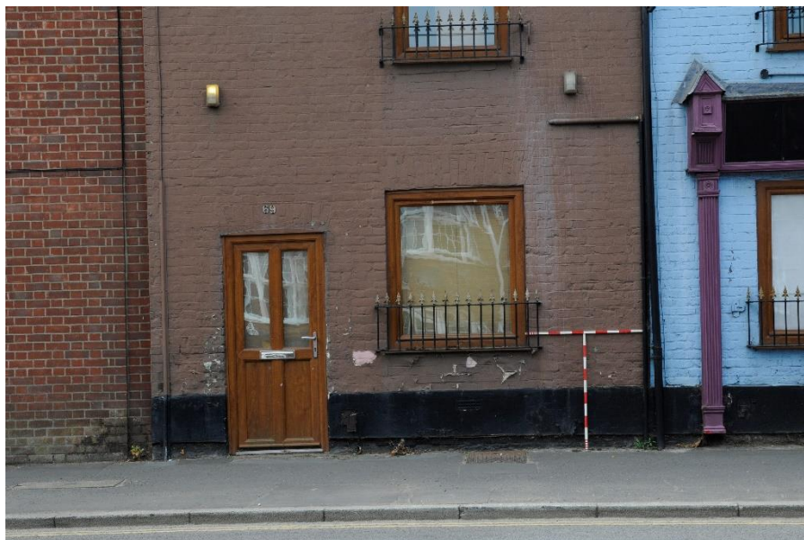
Figure 20 The ground floor level of No. 69
