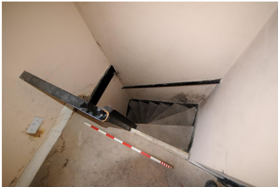
Figure 13 View of the winder stair from Room F1
