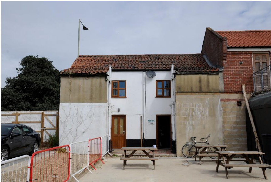
Figure 25 No. 67 and 69 viewed from the south and showing the rear extensions
