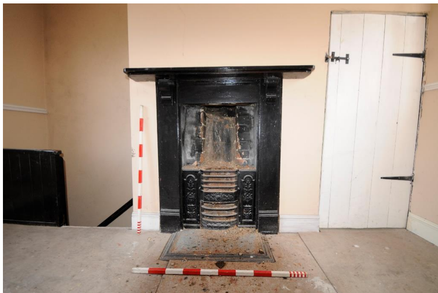
Figure 16 Detail of the cast iron fireplace
