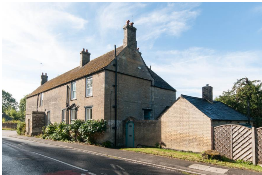
Figure 11 General view of Mill Cottages from Nene Way, looking south-east
