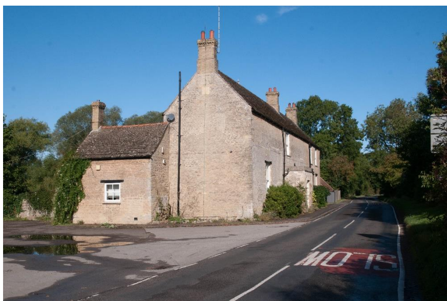
Figure 12 General view of Mill Cottages from Nene Way, looking north-west
