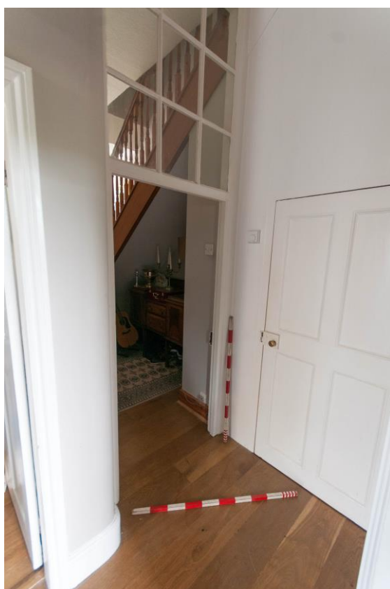
Figure 50 Transition between hall and staircase at south end of the hall
