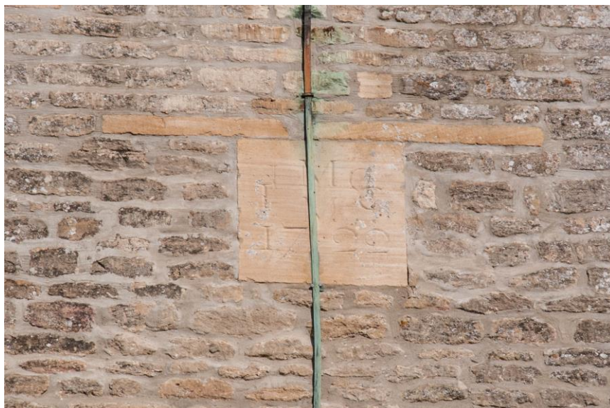
Figure 13 Detail of date stone with date of 1722 on south gable
