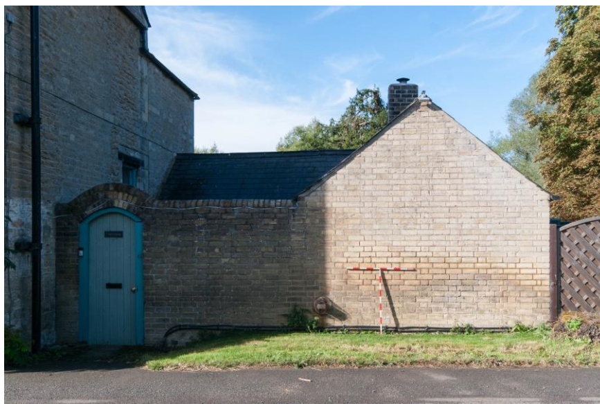
Figure 14 The eastern courtyard wall and gable end of outbuilding
