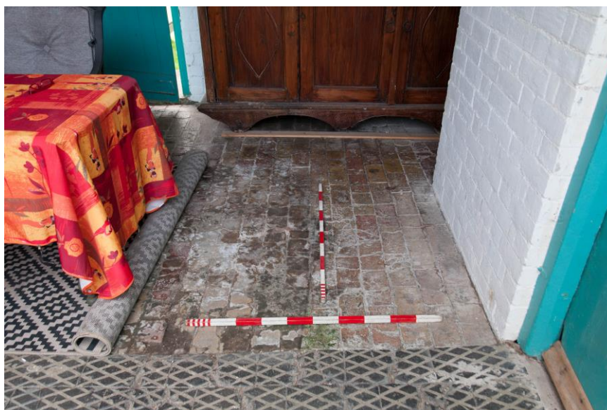
Figure 40 Detail of floor surface in the west range
