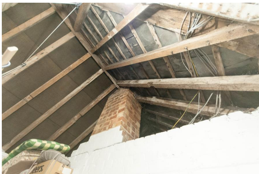
Figure 34 Chimney between the utility and storage rooms
