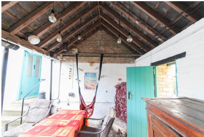
Figure 25 View within the west range, looking south
