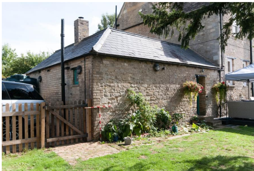
Figure 17 The join of the north and west ranges showing change between stone and brick walls
