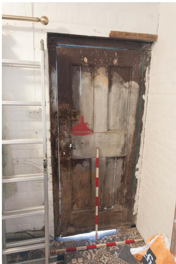
Figure 37 Detail of door to storage room
