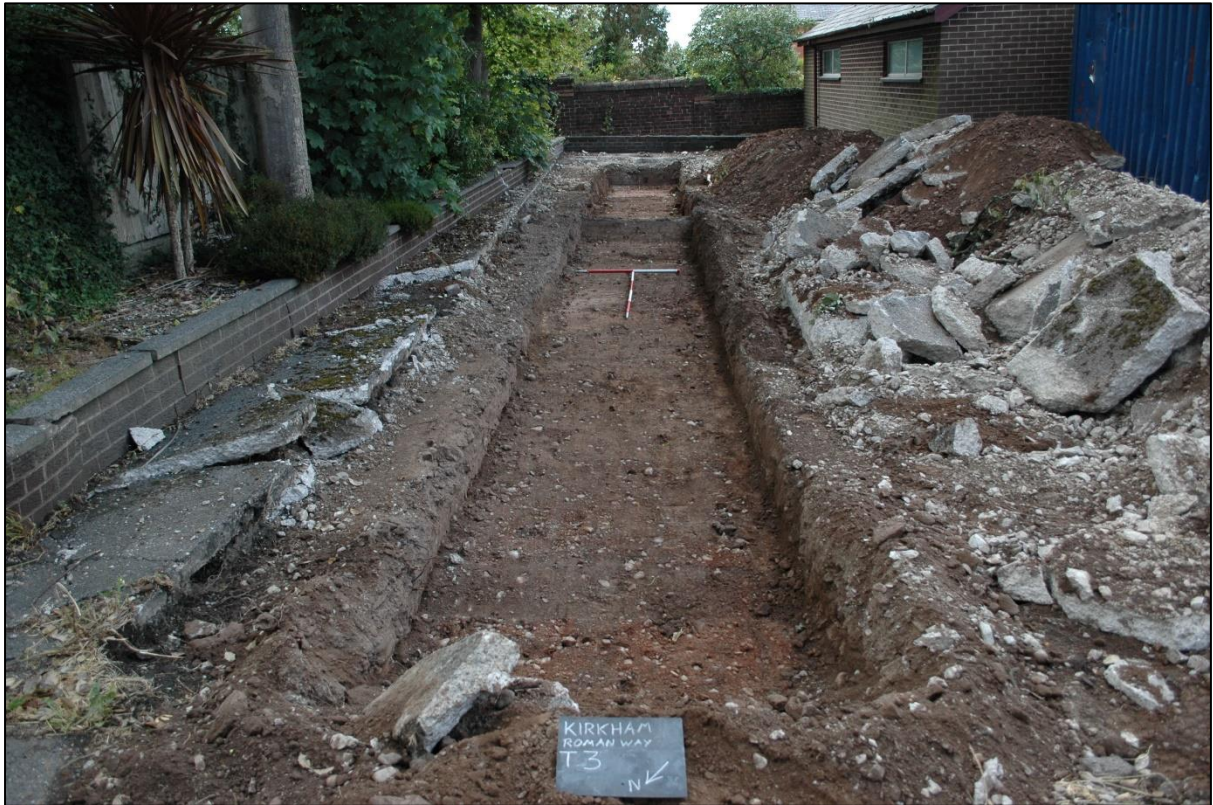
Plate 15: general shot of trench from the west
