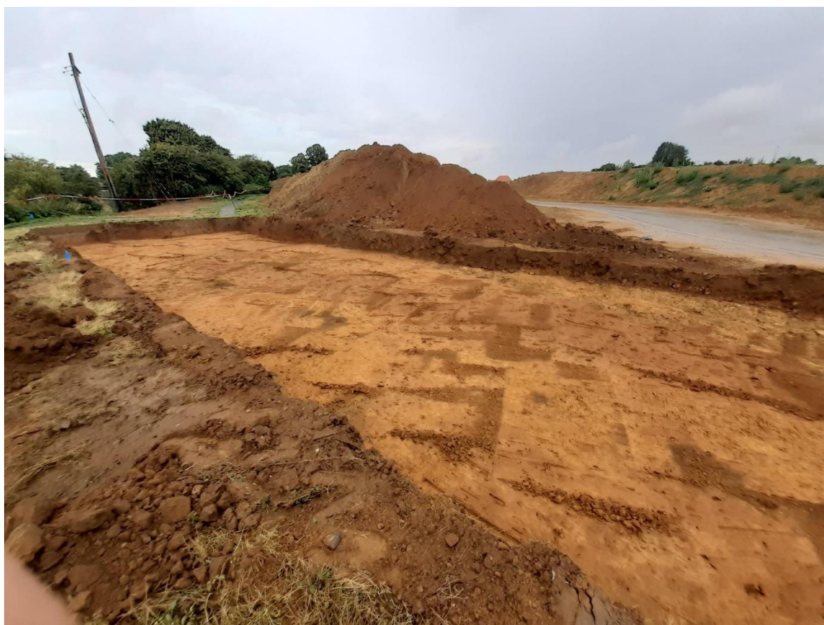
Plate 18: Stripped SW part of enclosure after removal of powerlines
