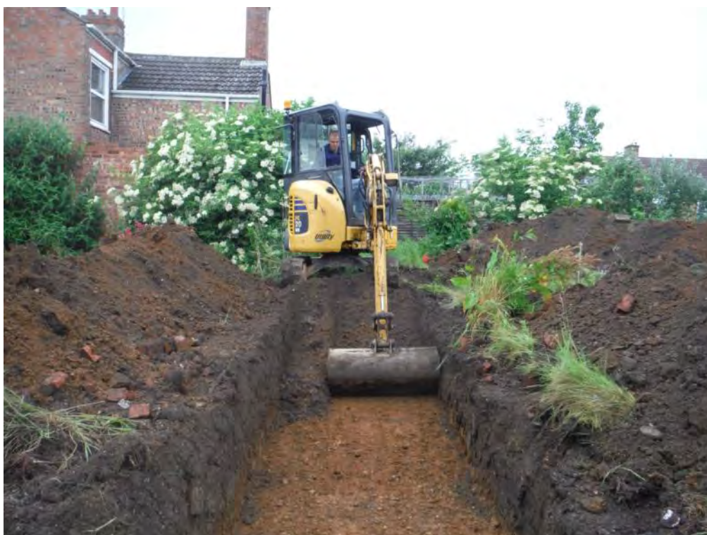
Plate 2: Machining of site, view west
