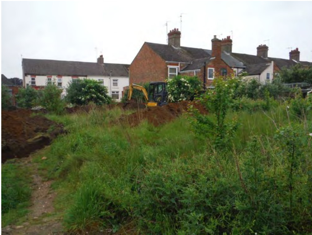
Plate 5: Site post-excavation, view southwest
