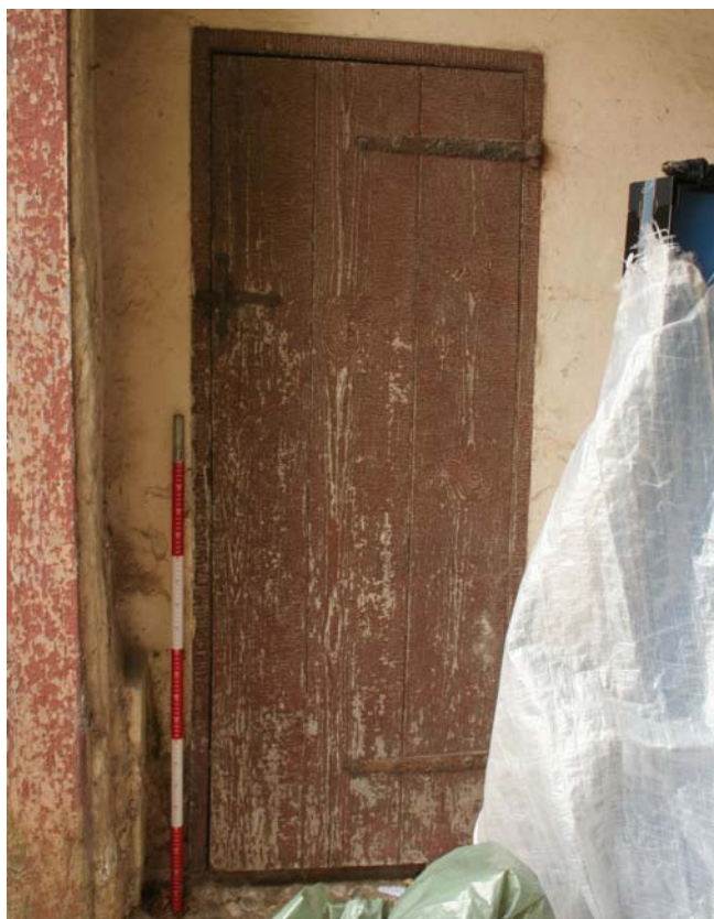
Plate 11: Ground floor interior, detail (Door to storage space under stairs)
