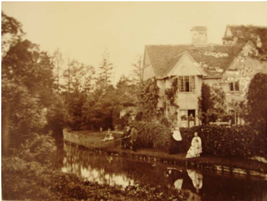
Pirton Grange undated photograph (HRO Gerish Box 61)
