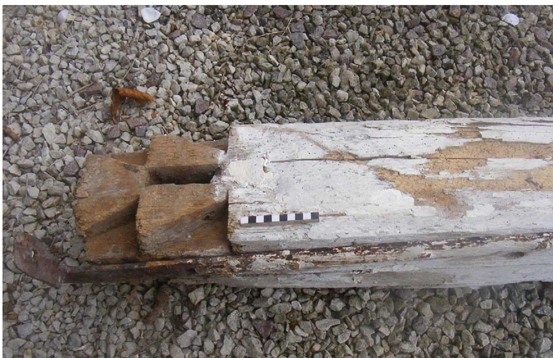
Plate 19: Central tie beam, detail
