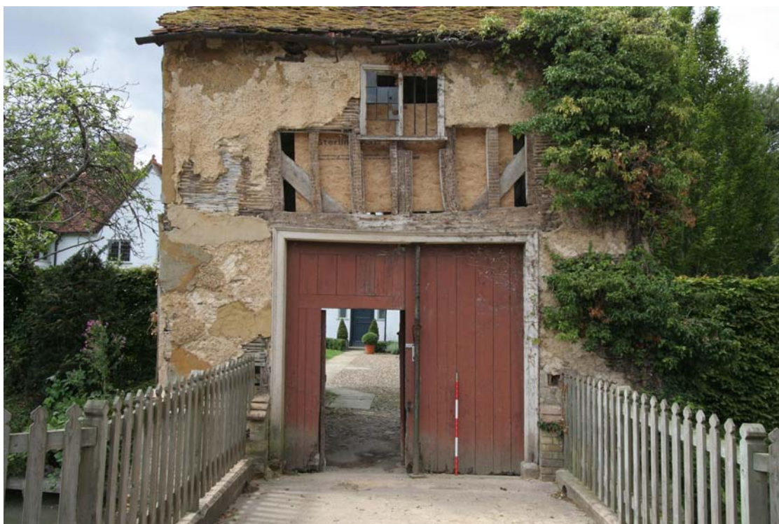
Plate 2: East elevation (After partial removal of plant growth and external render)
