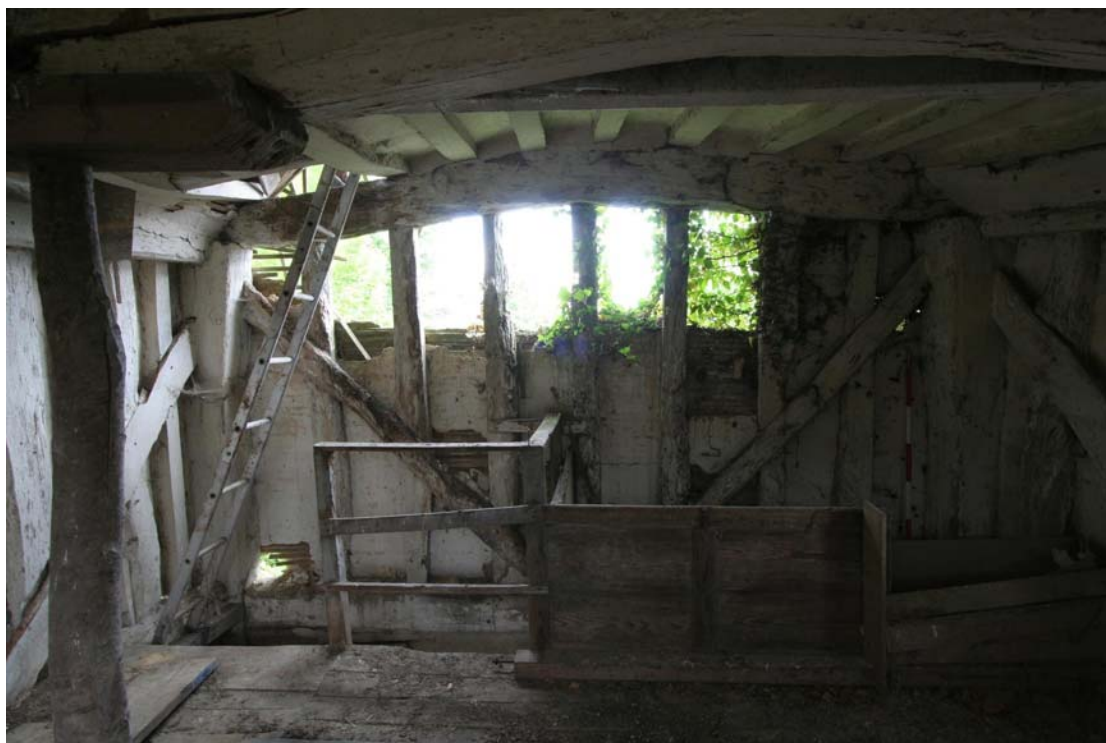
Plate 13: First floor interior, north wall
