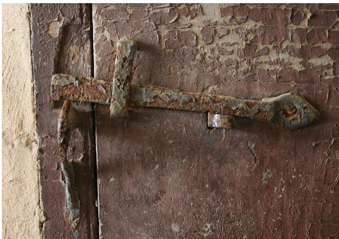
Plate 10: Ground floor interior, detail (Latch on door to stairs)
