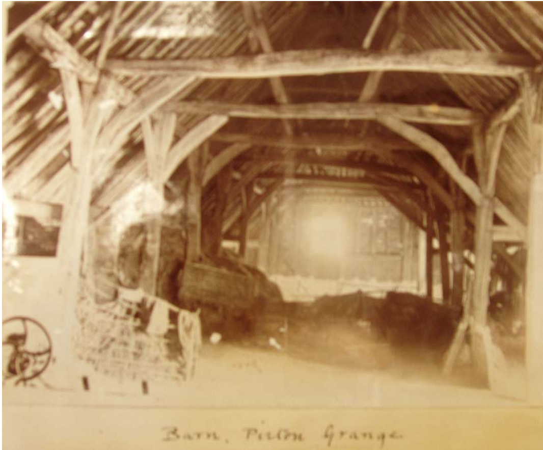
Barn at Pirton Grange, undated photograph (HRO Hine 4). This is probably the seven-bay Listed Grade II late 16 th century barn to the NE of the Gatehouse.
