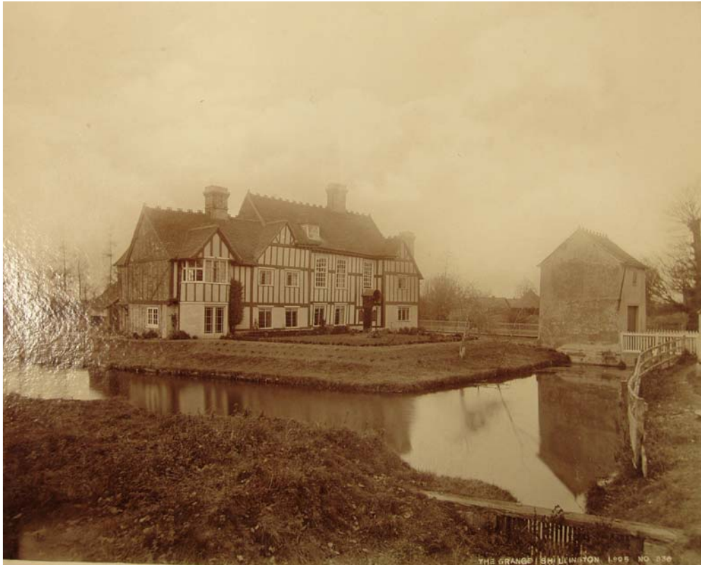
Pirton Grange 1895 (HRO Gerish Box 61) This shows the site after alterations to the Grange. The garden walls have gone and the sides of the moat cleared of vegetation.
