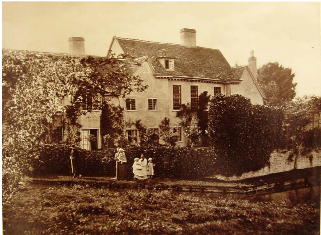
Pirton Grange undated photograph (HRO Gerish Box 61)
