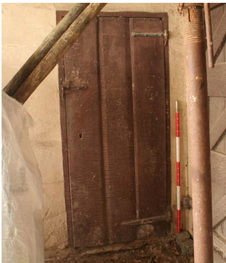
Plate 9: Ground floor interior, detail (Door to stairs)
