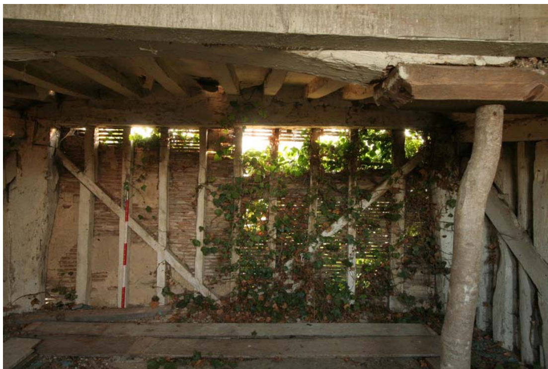
Plate 15: First floor interior, south wall
