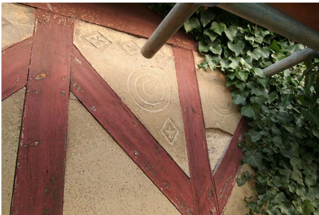
Plate 5: West elevation showing pargetting (Showing designs impressed in the cement render inside the top row of chevrons)
