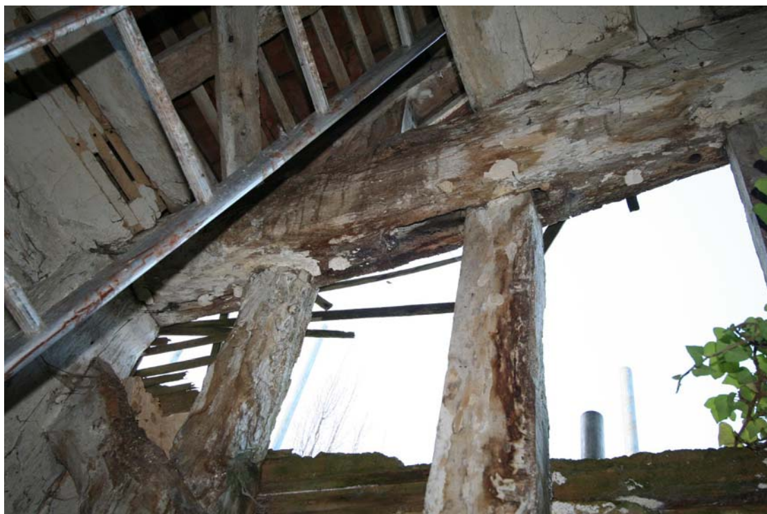
Plate 17: First floor interior, detail (Showing stave holes and empty mortise at west end of north tie beam)
