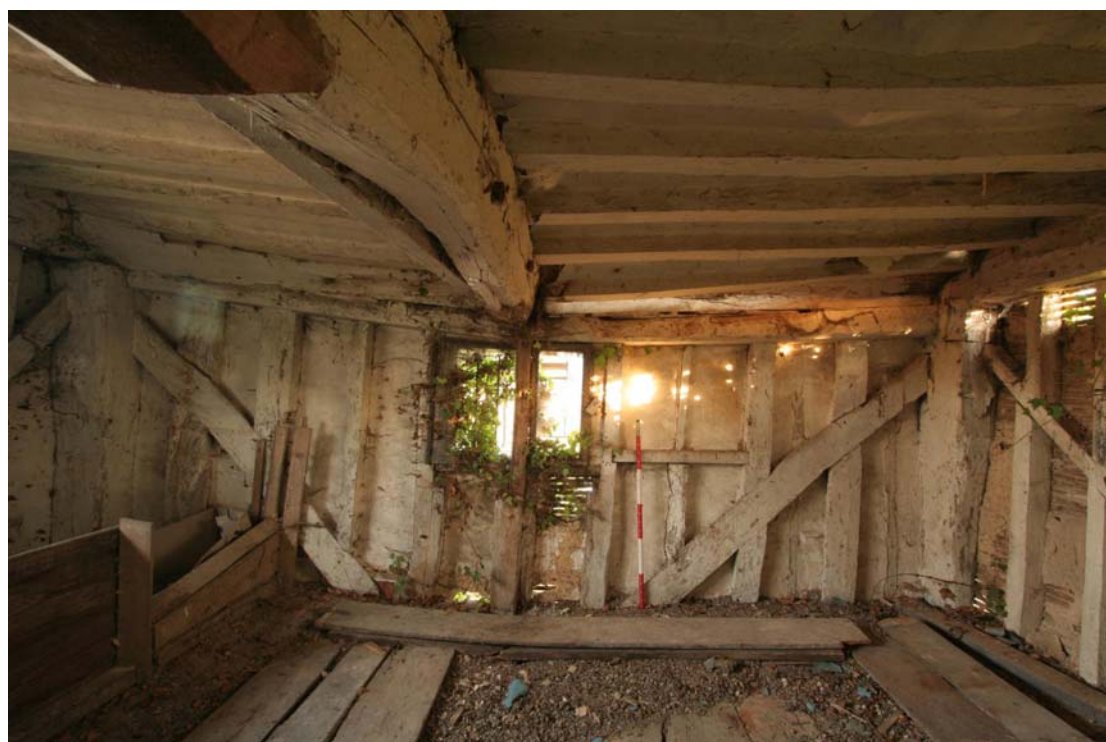
Plate 14: First floor interior, east wall
