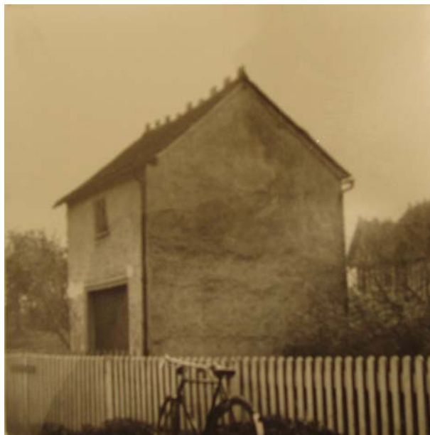
Pirton Grange Gatehouse c.1930-50, (HRO PIR/1) photograph by H Hallar, N & E elevations
