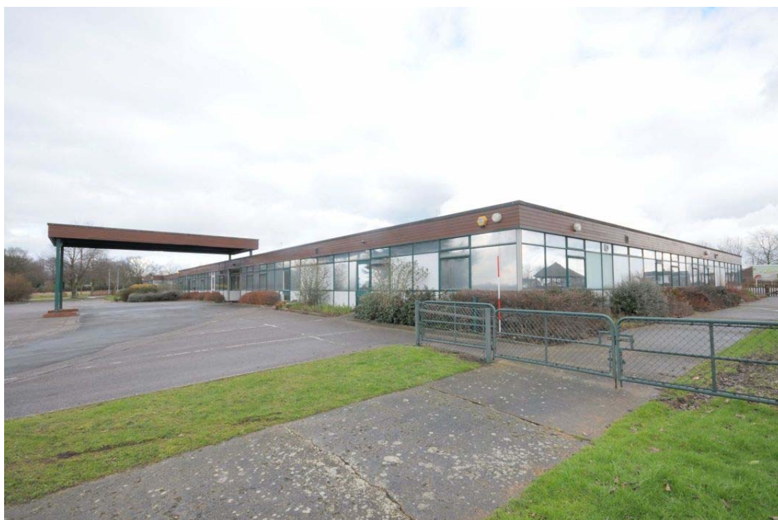
Figure 7: Main western façade, south-western corner
