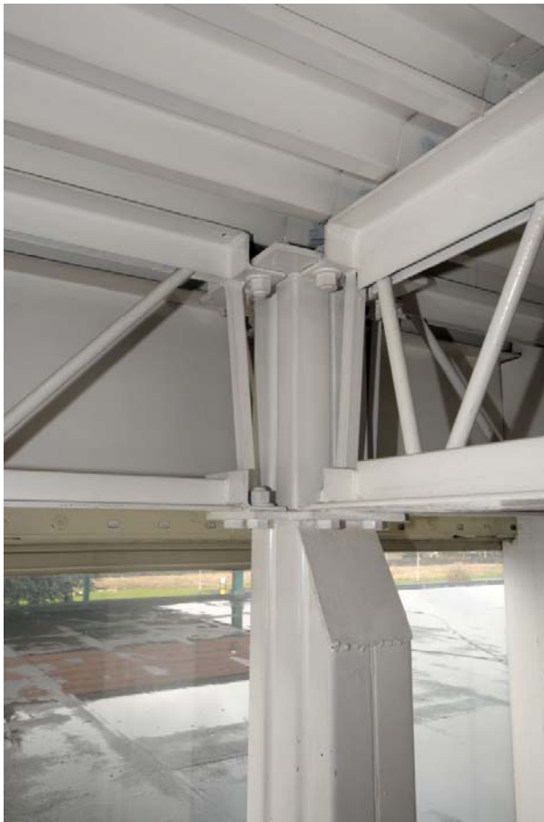
Figure 30: Physiotherapy hall, ceiling with lattice girders
