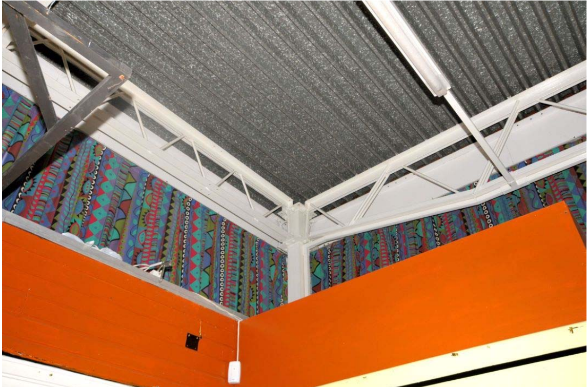
Figure 25: Main hall ceiling, lattice girder detail
