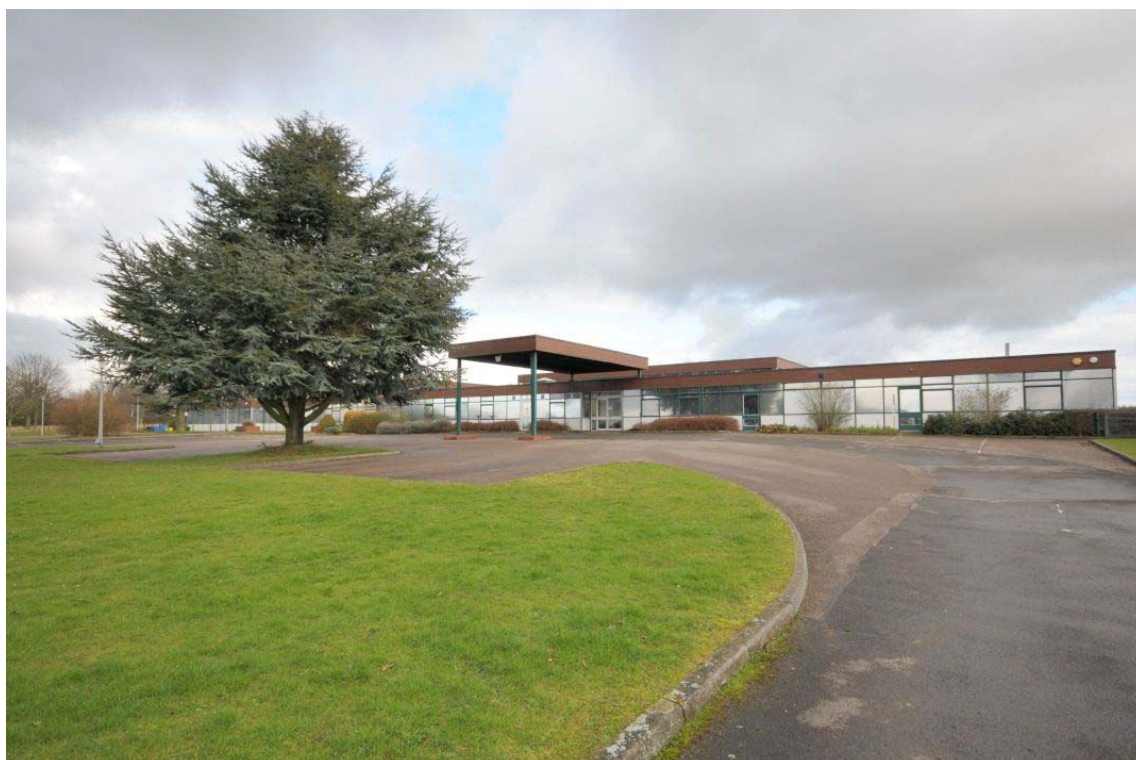
Figure 6: Main western façade
