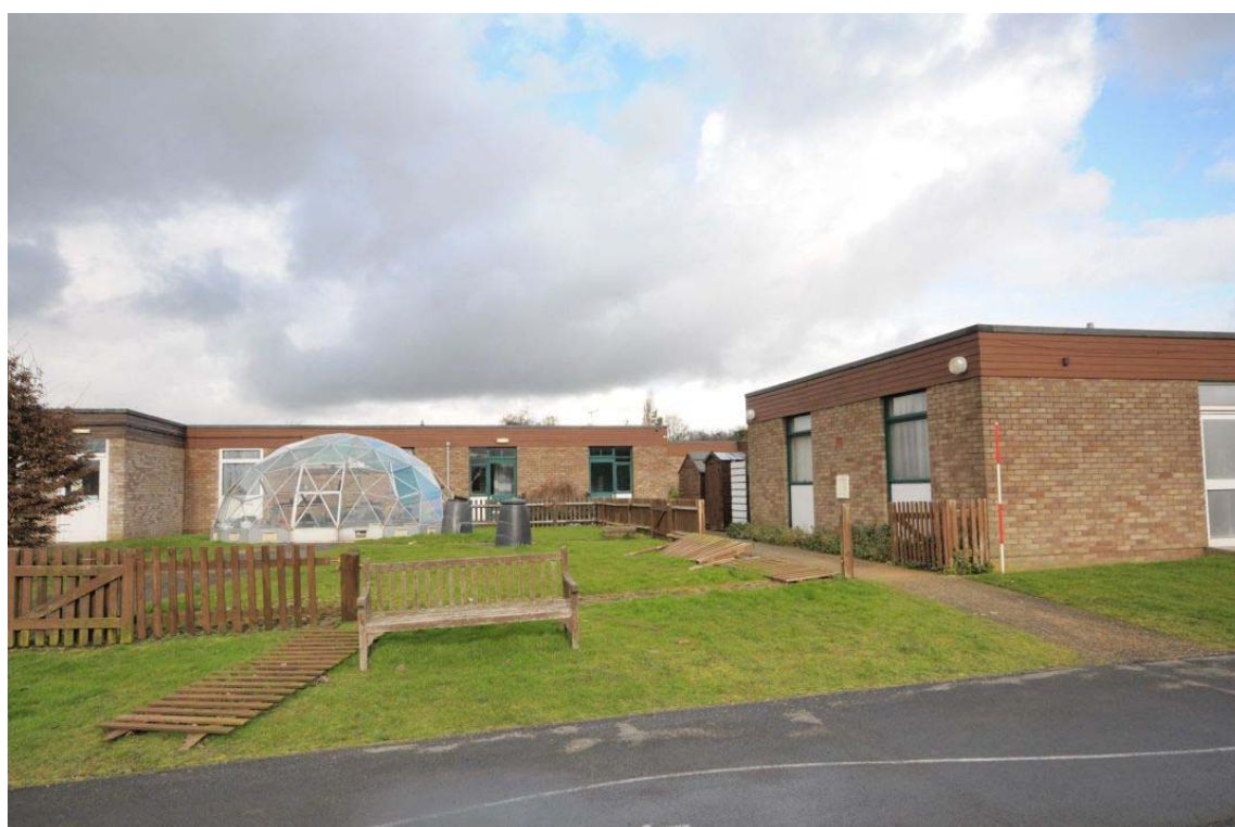
Figure 13: Residential block, southern side
