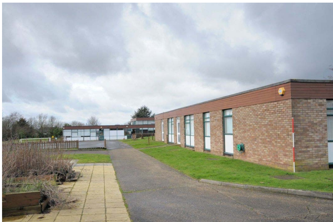
Figure 12: North-eastern corner of residential block (now classrooms), looking west towards teaching block
