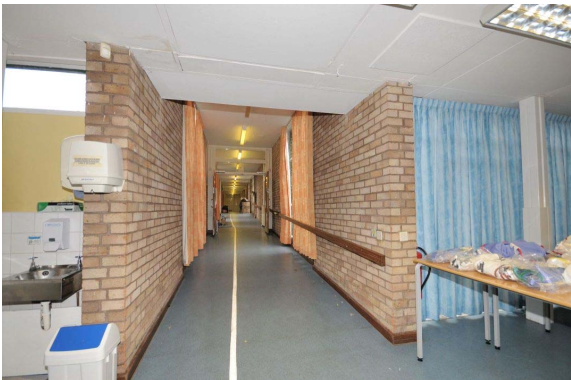
Figure 33: Central corridor, wooden handrail along inclined section towards residential block
