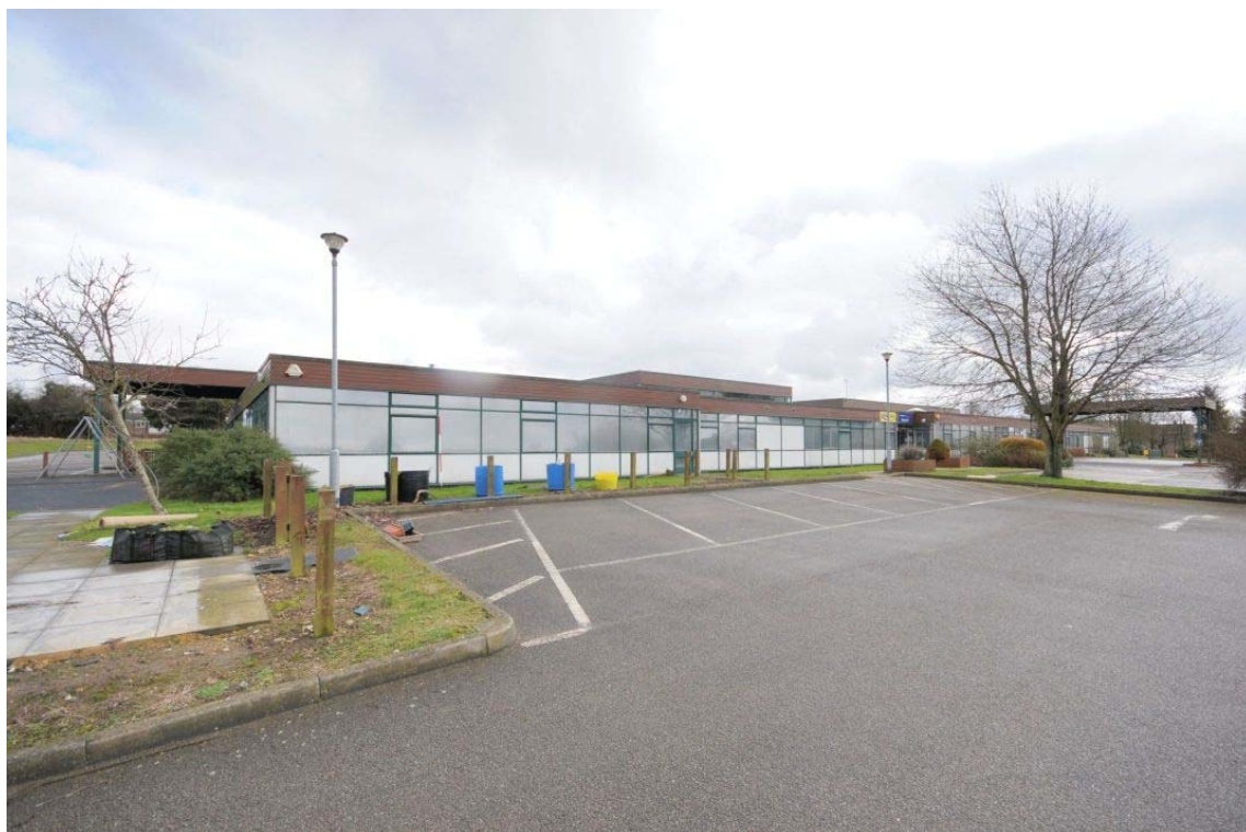
Figure 8: Main western façade, north-western corner
