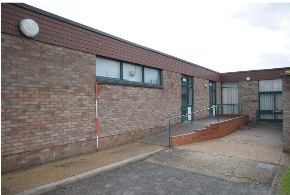
Figure 10: Chiltern residential unit, western side with wheelchair ramp
