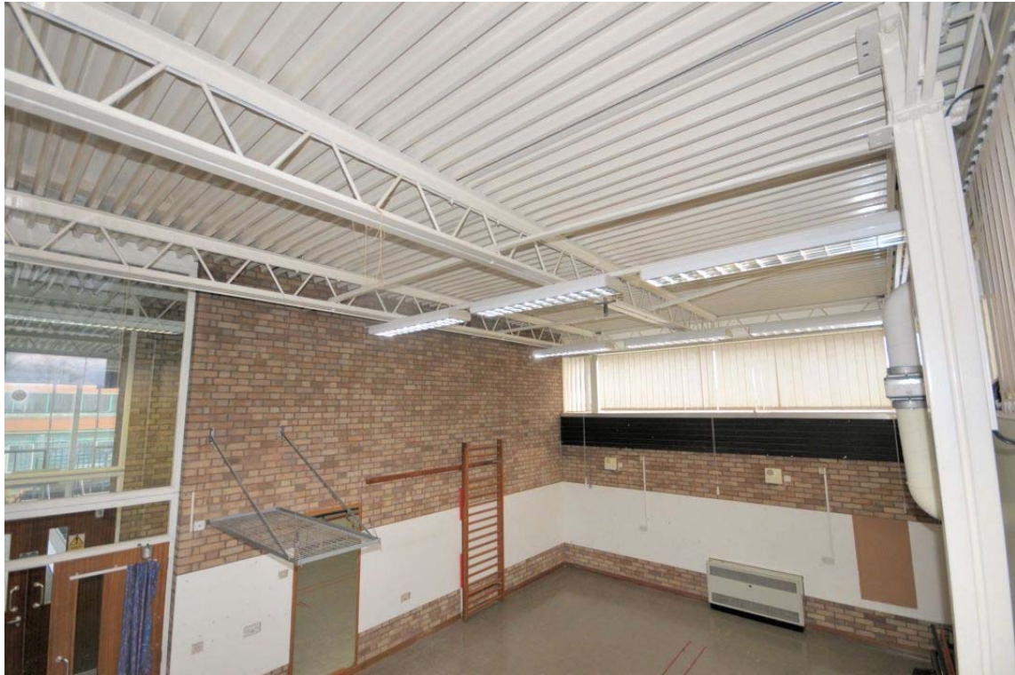
Figure 30: Physiotherapy hall, ceiling with lattice girders
