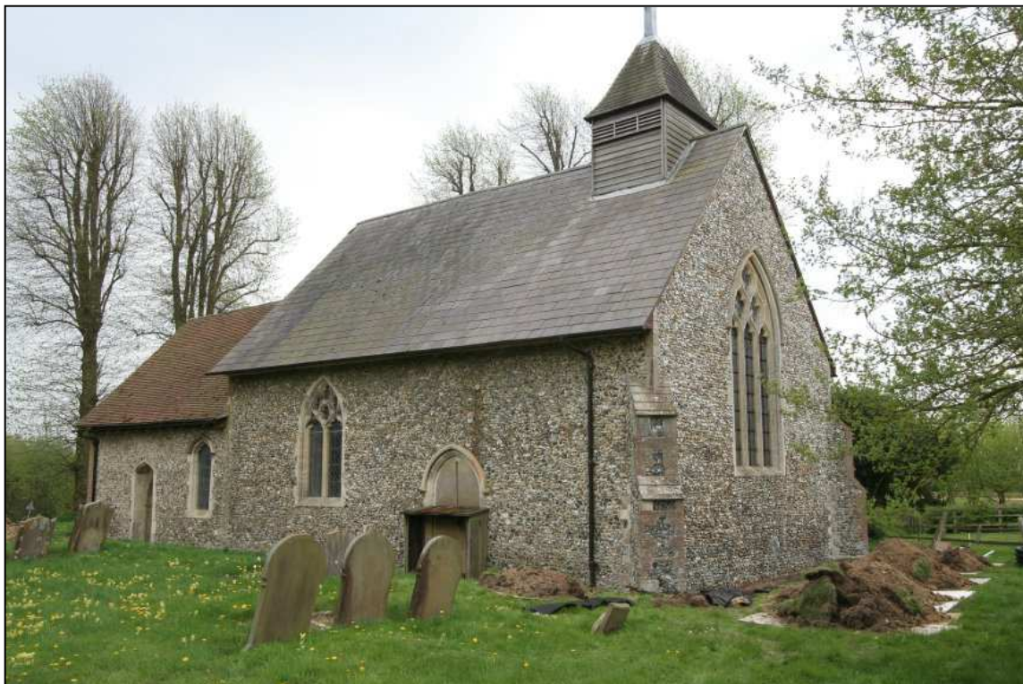
Image 2: View of north side and west end of church, showing location of trench at west end
