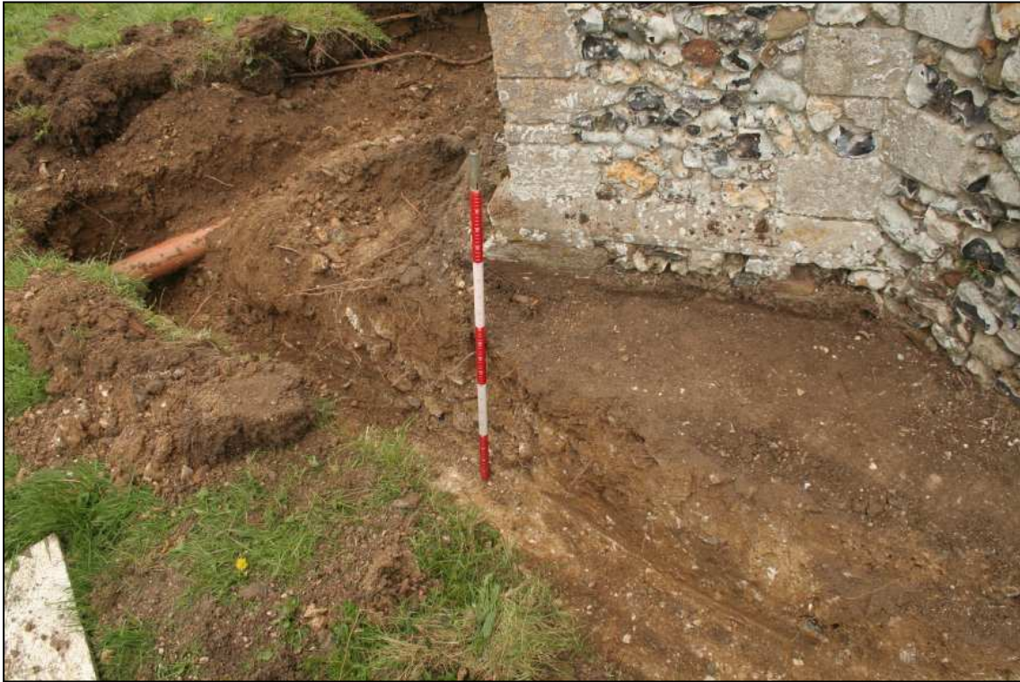
Image 5: Trench at west end of church showing area next to the north-west buttress, showing flint and mortar of foundation visible in section (scale 1m)
