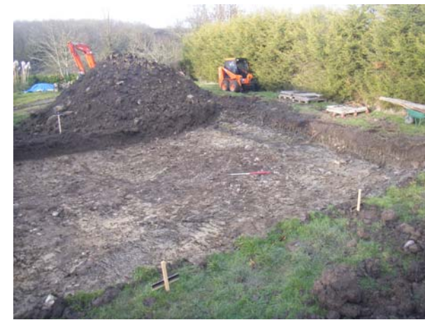
Trench within footprint of new house, looking north. Scale 1m
