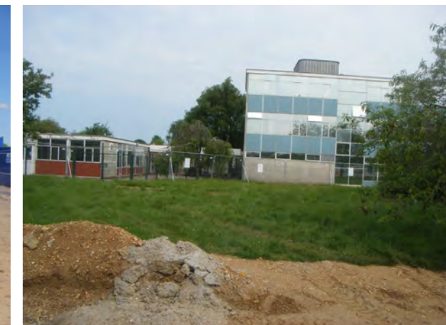
View of location of Trench 5 Facing NW
