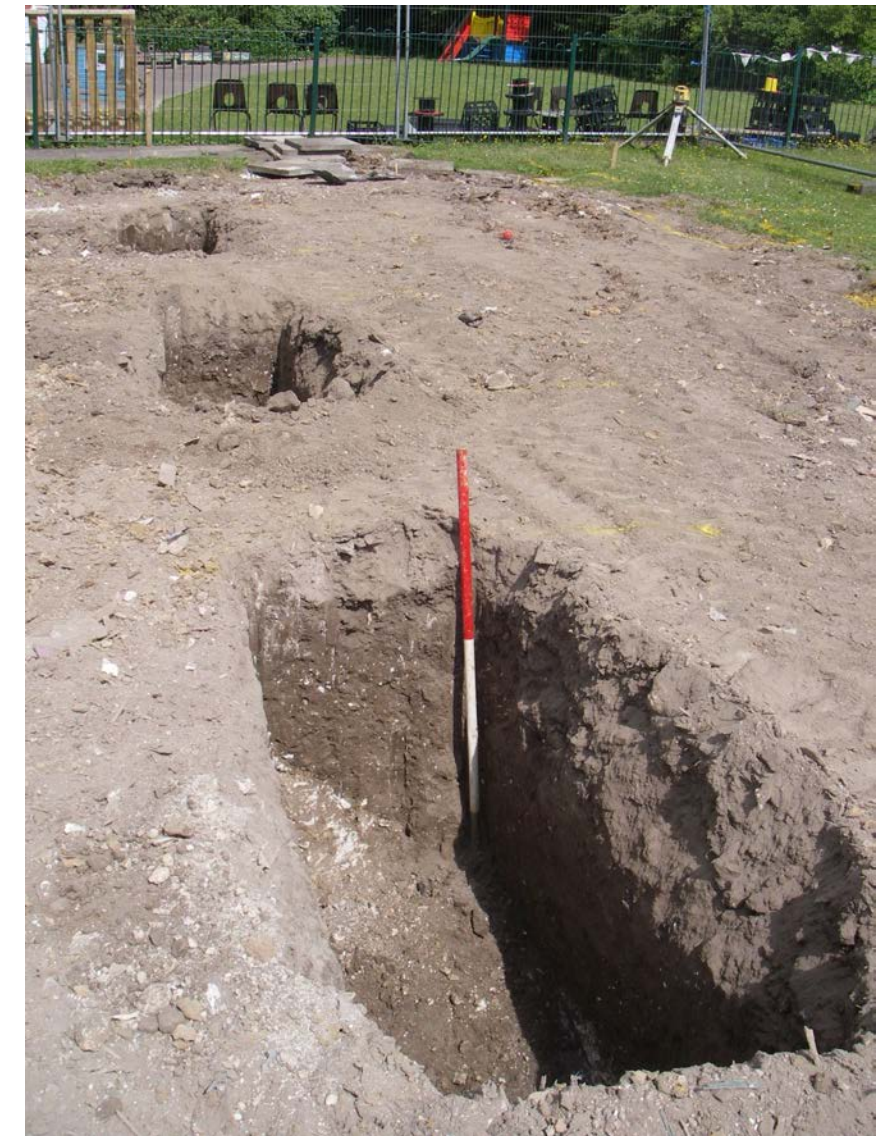
Foundation pads 1-4, looking east (Pit [019] visible in foreground section)
