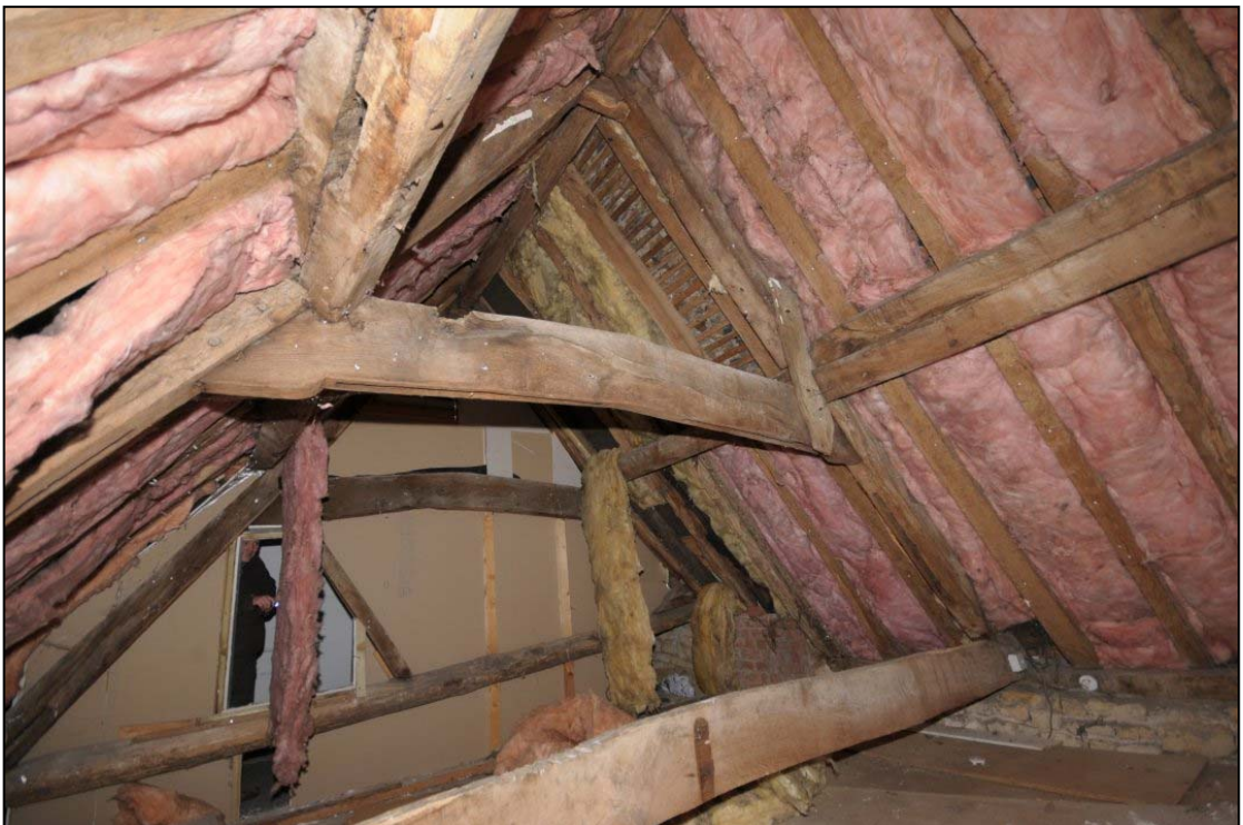
Figure 54: Attic S1, facing north-west
