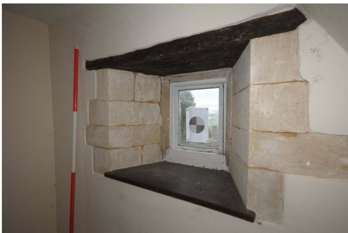
Figure 64: Room S4, detail of window in east wall
