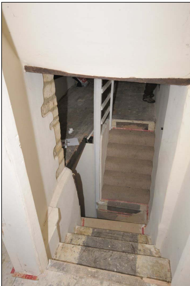
Figure 61: Stairs between rooms S3 and S4
