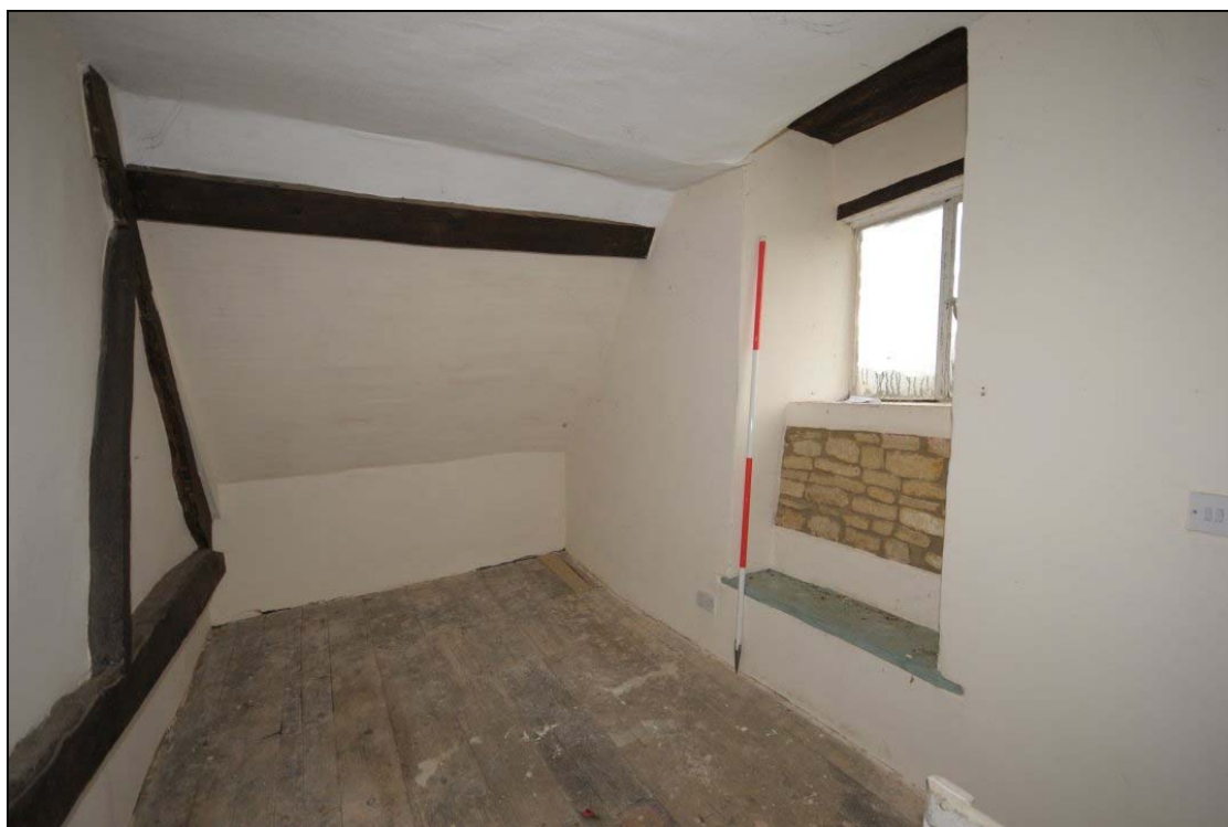
Figure 59: Attic room S3, facing south-west
