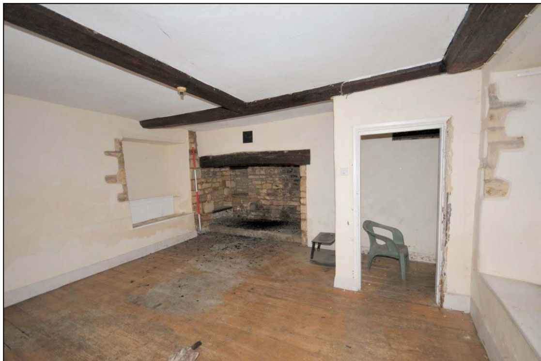
Figure 26: Room G4 facing north-east
