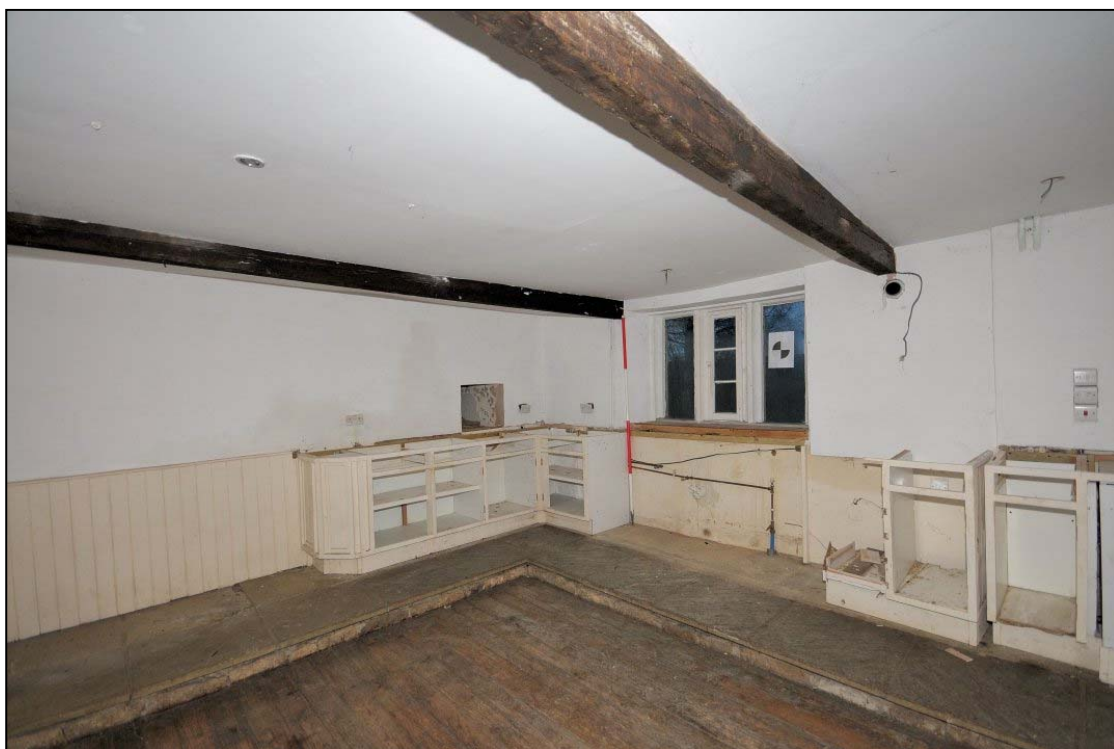
Figure 29: Room G5 facing north-west
