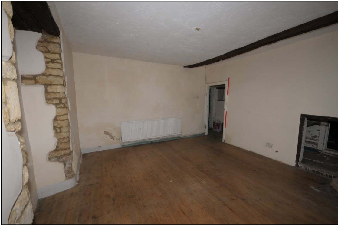
Figure 25: Room G3 facing north-east
