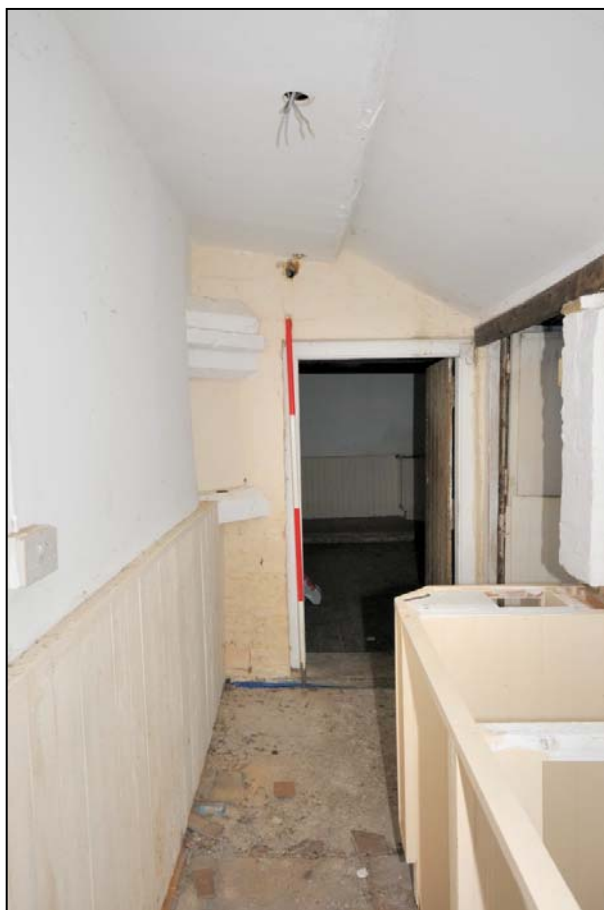
Figure 33: Ground floor lean-to extension, facing west
