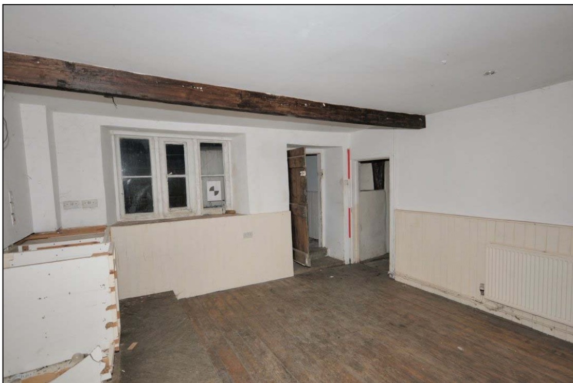
Figure 30: Room G5 facing south-east
