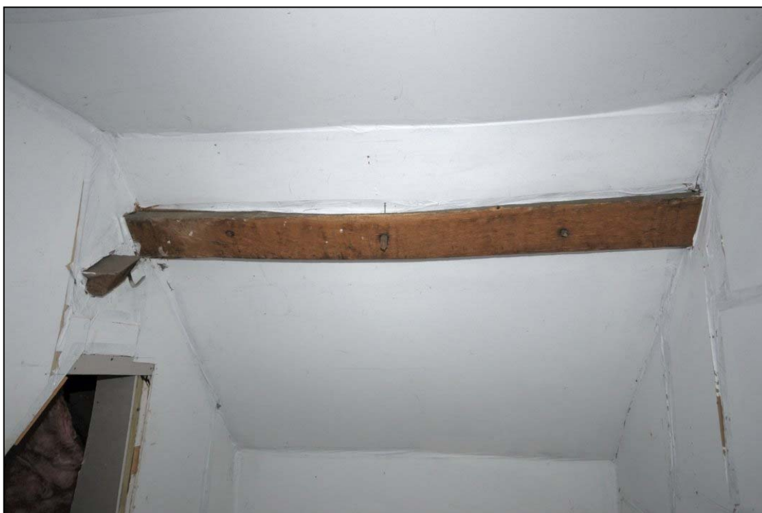
Figure 58: Attic S2, facing south
