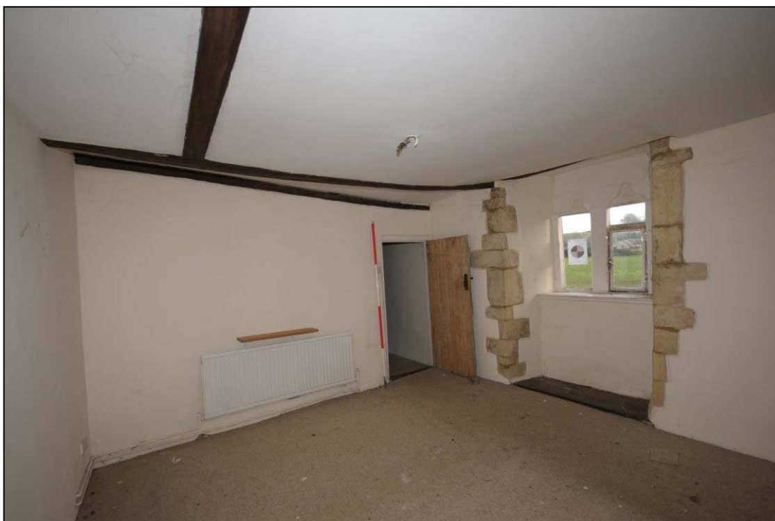
Figure 47: Room F4, facing south-east
