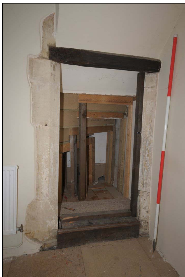
Figure 50: Room F5, detail of former door way
