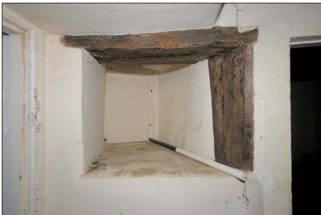
Figure 32: Detail of squint facing north-east
