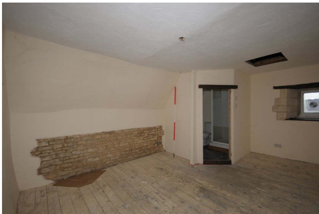
Figure 63: Room S4, facing north-east
