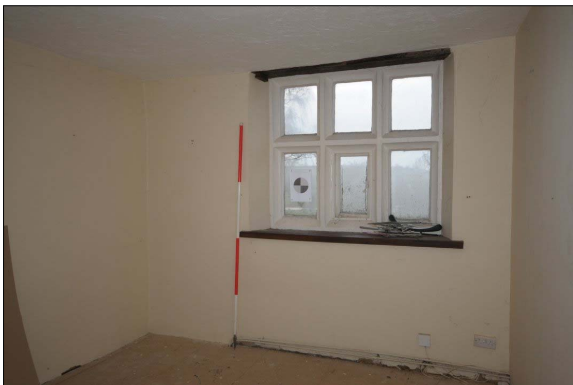
Figure 48: Room F5, facing north-west
