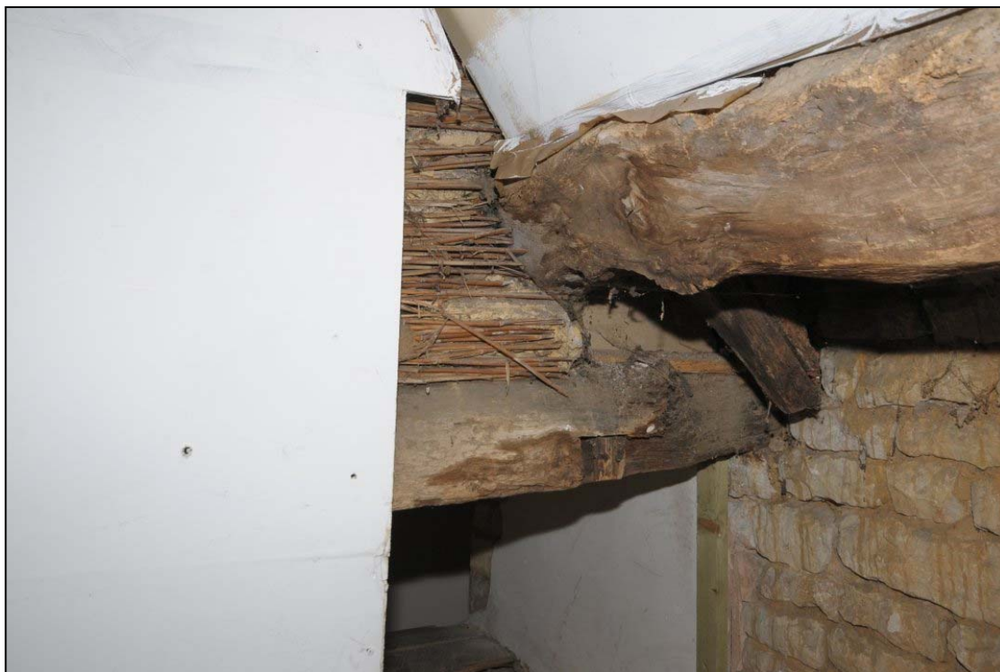
Figure 57: Attic S2, detail of reed and daub/plaster infill
