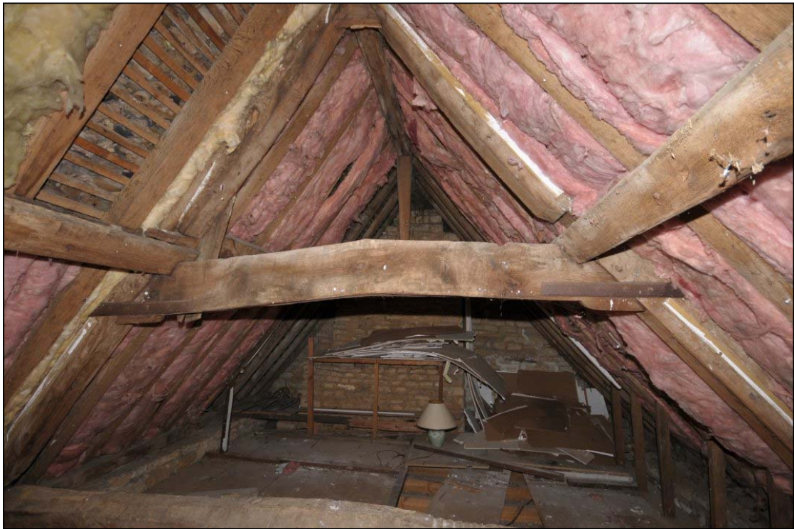
Figure 53: Attic S1, facing east
