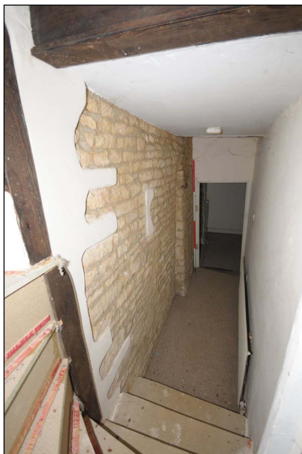
Figure 52: First floor corridor, facing east
