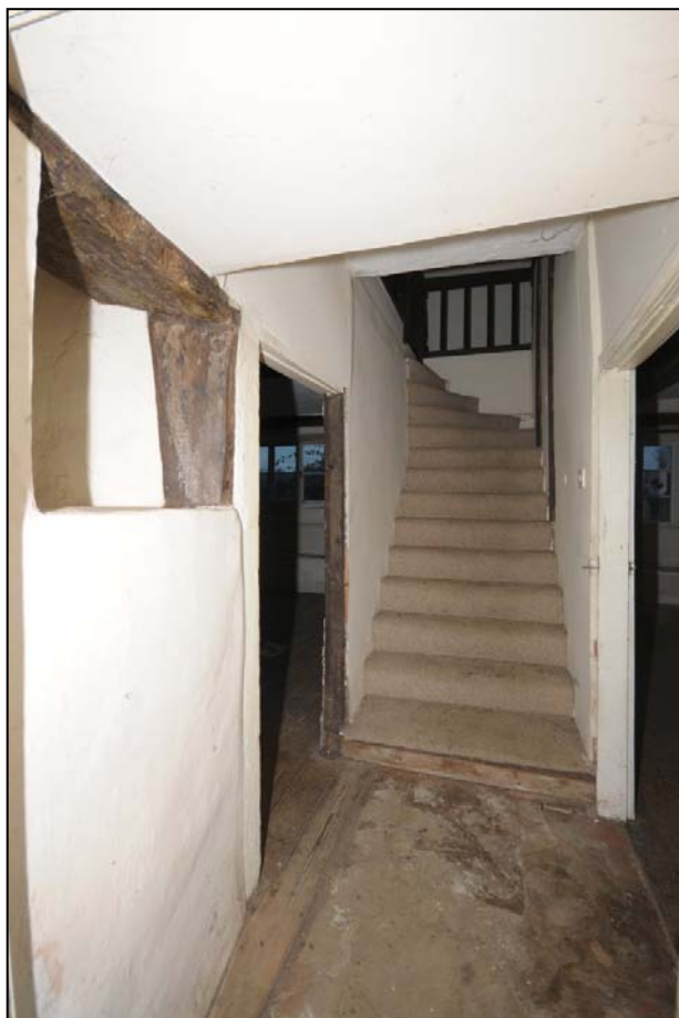
Figure 31: Hall between G3 and G4
