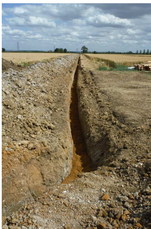
Image 6: General view along the cable trench looking towards the south-east.
