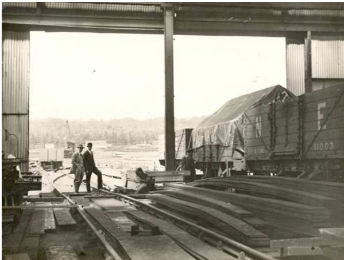
Dawney & Sons factory interior and railway siding 1928 ( LDA Chartered Architects )
