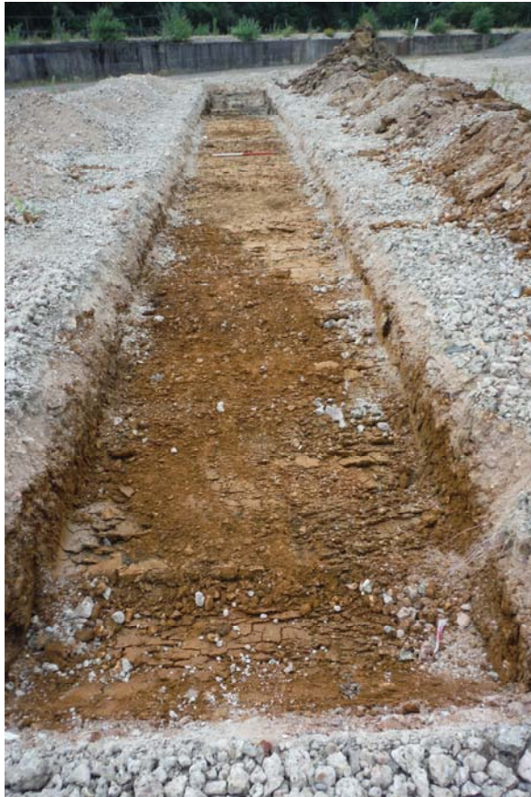
Trench 9 facing south-west
