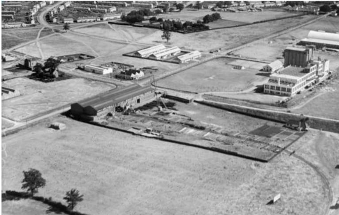
Aerial view of the application site occupied by Dawney & Sons 1928 ( LDA Chartered Architects )
