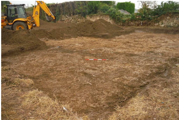
Machining of house footprint, looking south
