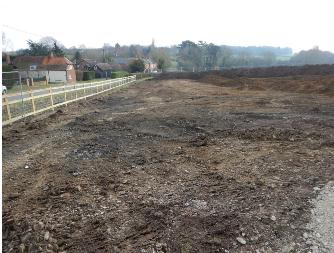
Image 8: Topsoil strip in the area to the south of Plot 2, adjacent to access road
