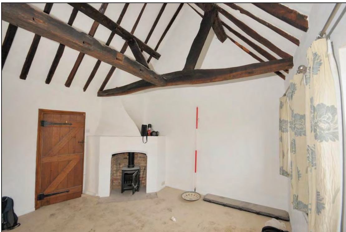
Image 17: Bedroom 2, looking south-east Showing corner fireplace and roof truss (Scale 2m).
