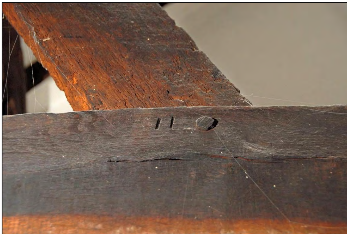
Image 20: Bedroom 2, detail of assembly mark
