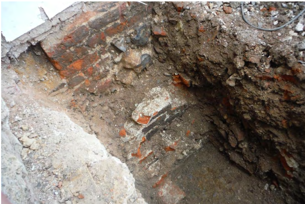
Image 29: Detail of the narrow gap between the cottage wall footing [113] and the demolished building [116]. The foundation trench for the cottage wall appears to have been infilled with flint nodules (115). The two footings are separated by a thin band of material (118).
