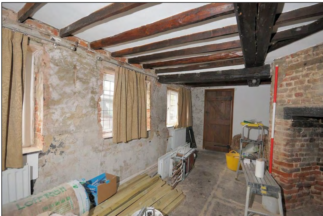
Image 10: Living area, general view looking north
