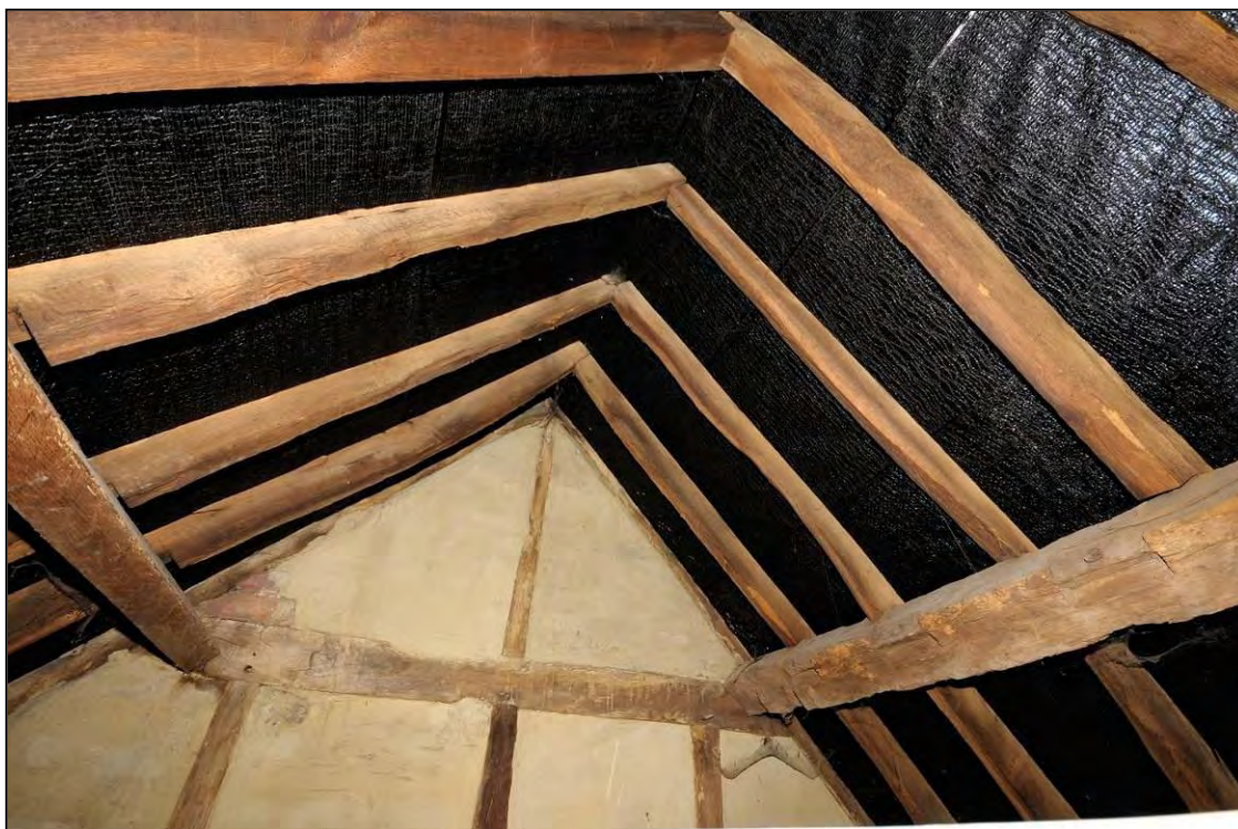
Image 25: Roof over northern part of rear range
