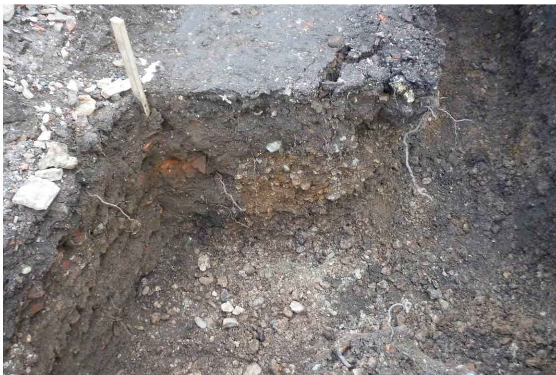
Image 33: West edge of pit [132], dug into the gravel geological strata. This would appear to be a continuation of pit [109] to the north, rather than wall footing (207) to the south.
