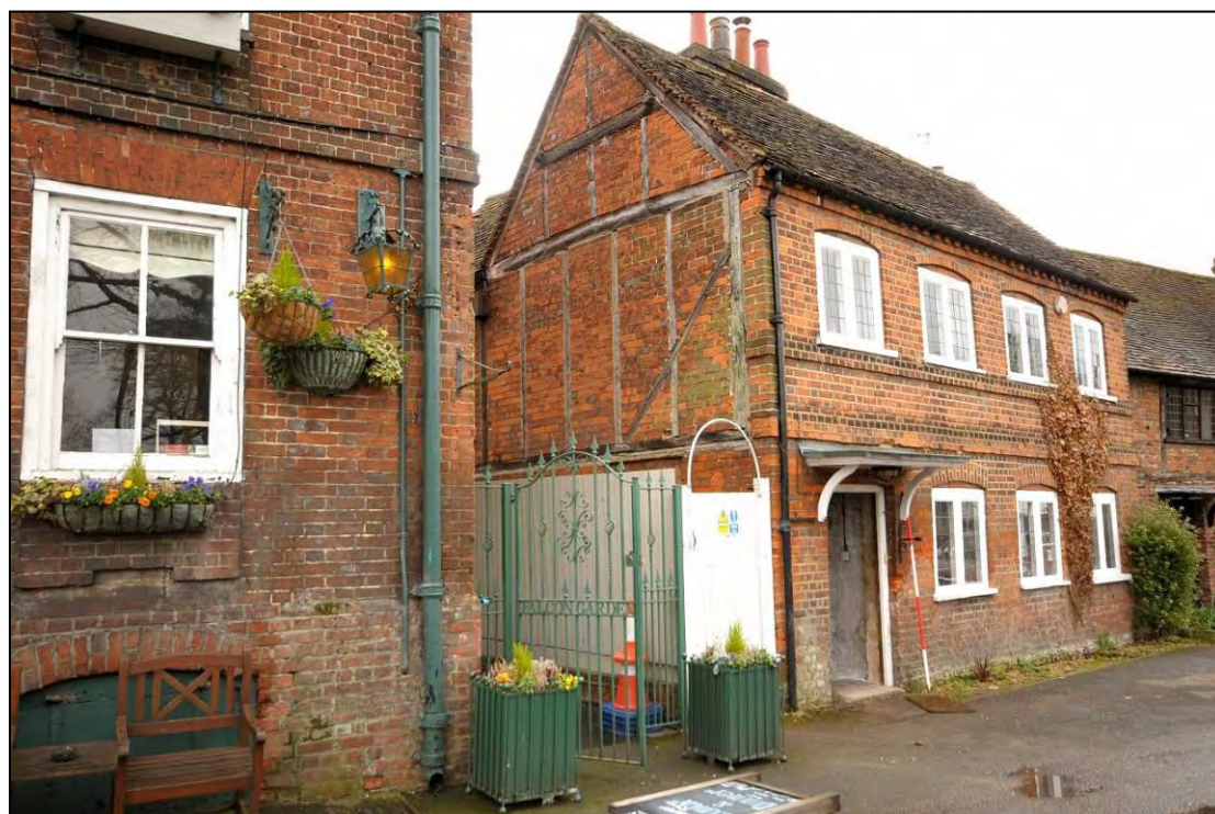
Image 2: Building viewed from north-west
