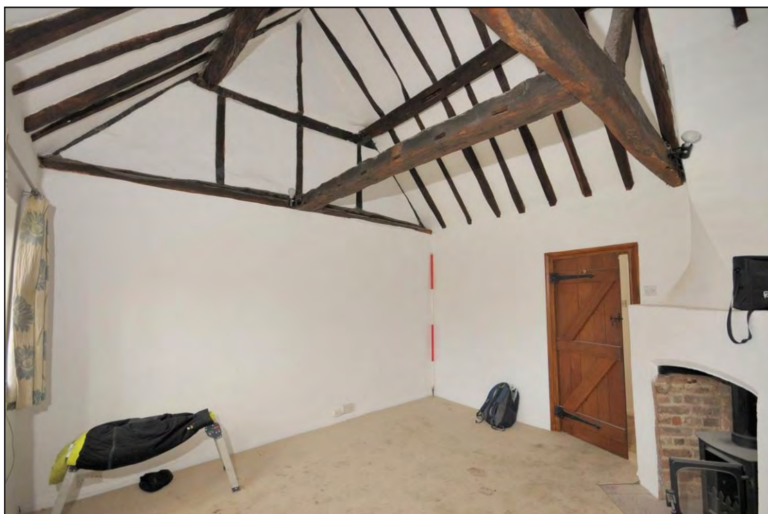
Image 18: Bedroom 2, looking north-east Showing timber frame in end wall and axial beam with empty mortise holes for ceiling/attic floor (Scale 2m).
