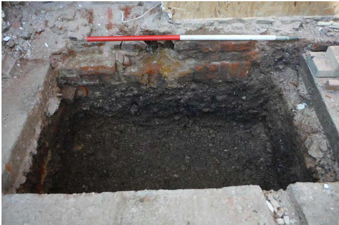
Image 30: Central pit exposing the footing for the cottage [119] / (120), with the underlying deposit (118). Scale 1m in 50cm divisions.
