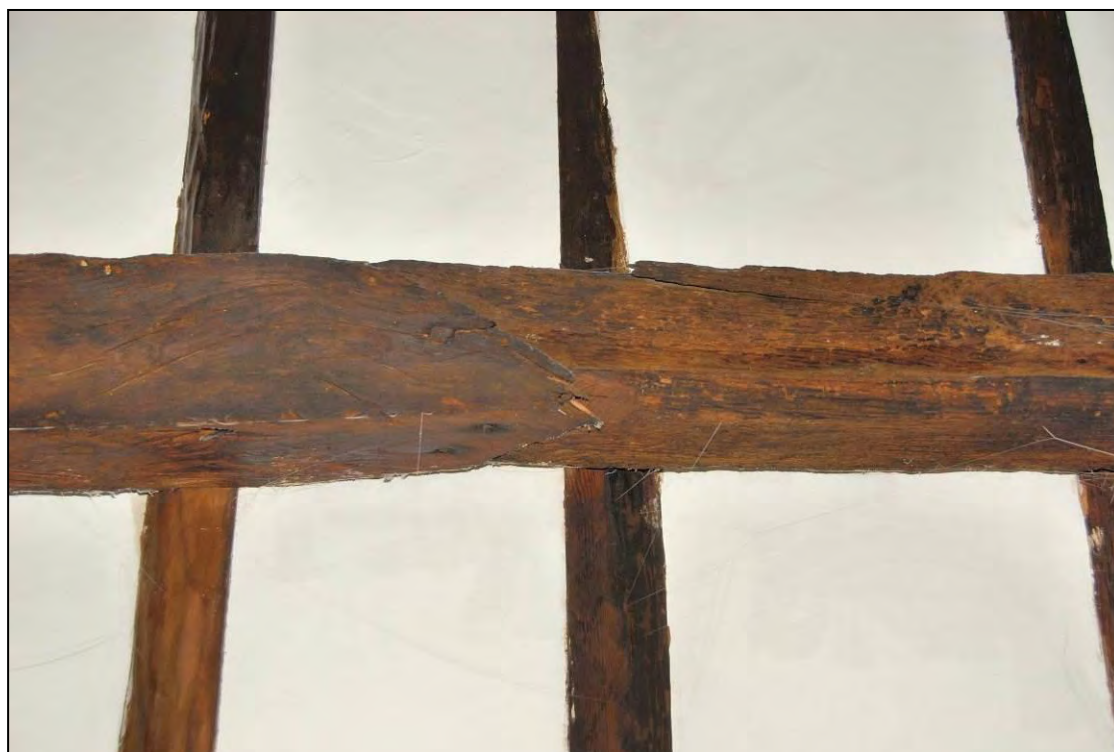
Image 19: Bedroom 2, scarf join in purlin
