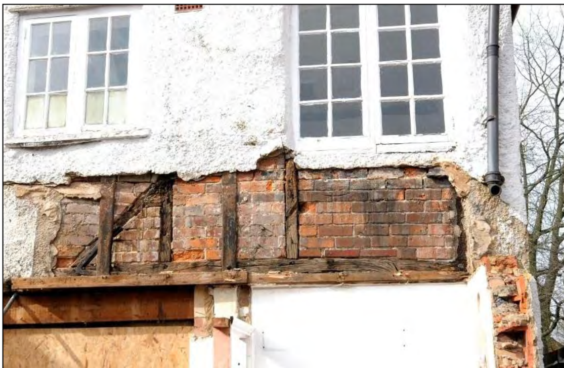
Image 5: Rear (east) elevation (detail)
