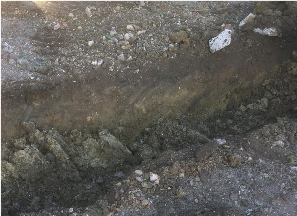
Image 1: Section through the disturbed soil profile following removal of the footings for the existing garage.
