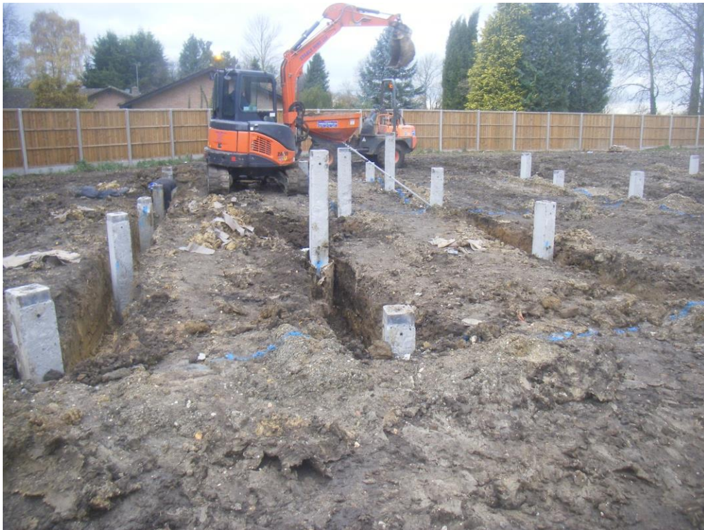
Image 3: Trenches under excavation to link the piles for the two buildings.
