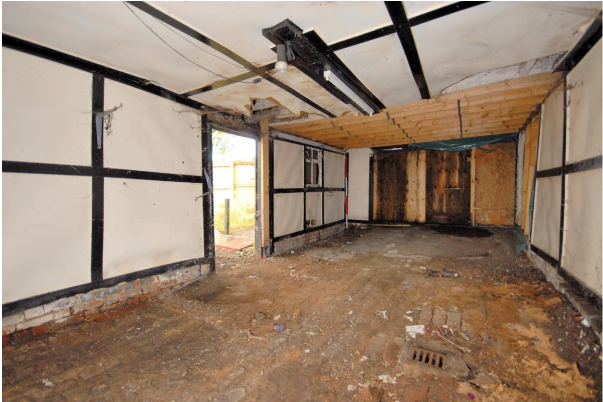
Figure 14: Northern room interior, looking NE
