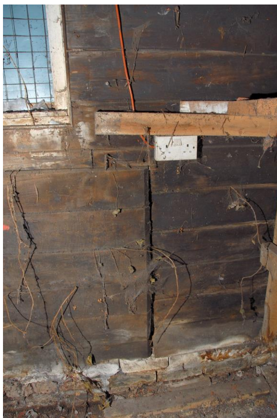
Figure 10: Reinforced lower wall panels (former horse boxes?) in south-central room
