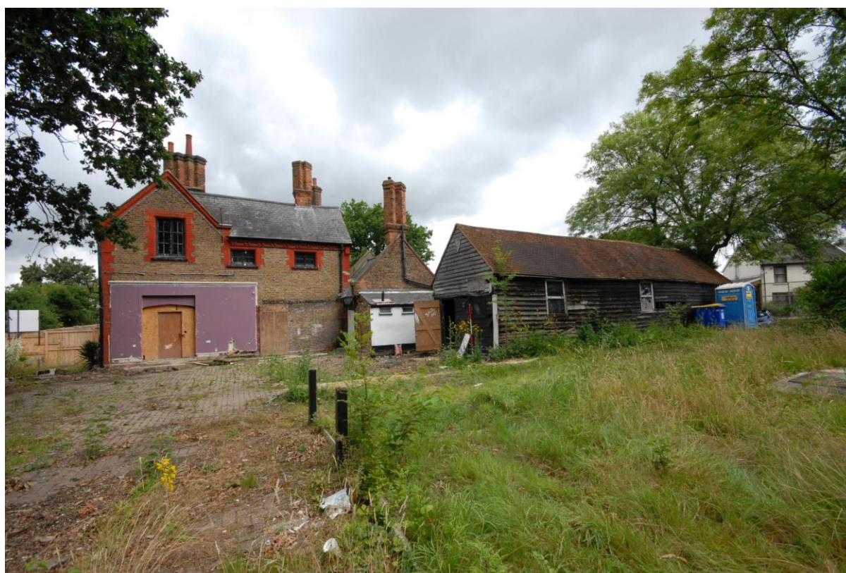
Figure 7: The Black Lion public house and former stable block, looking NNW
