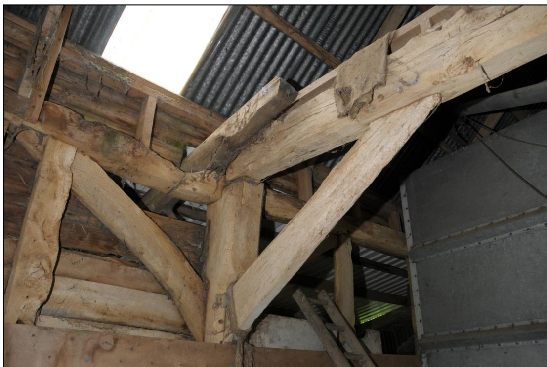
Image 10: Barn 1, interior south wall
