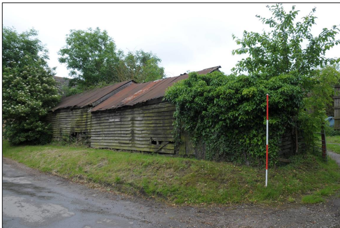
Image 31: Buildings 1 and 2, exterior
