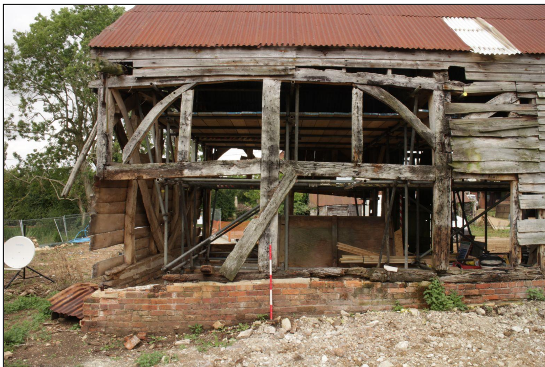
Image 7: Barn 1, exterior south side
