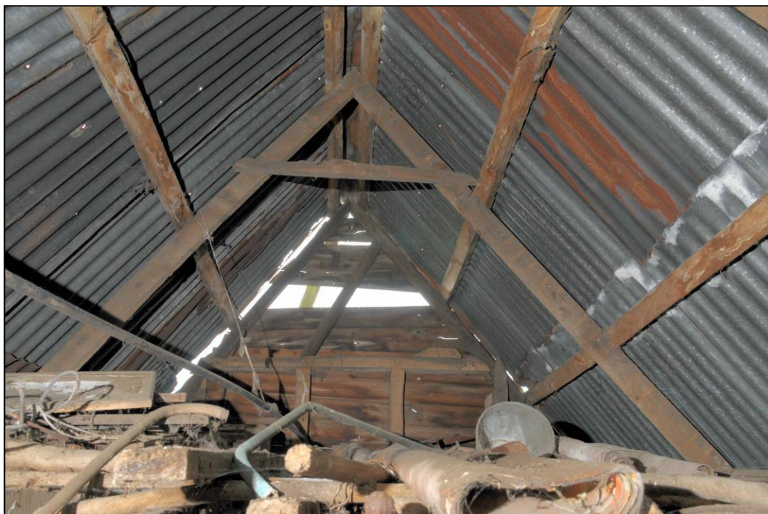
Image 30: Granary interior, roof
