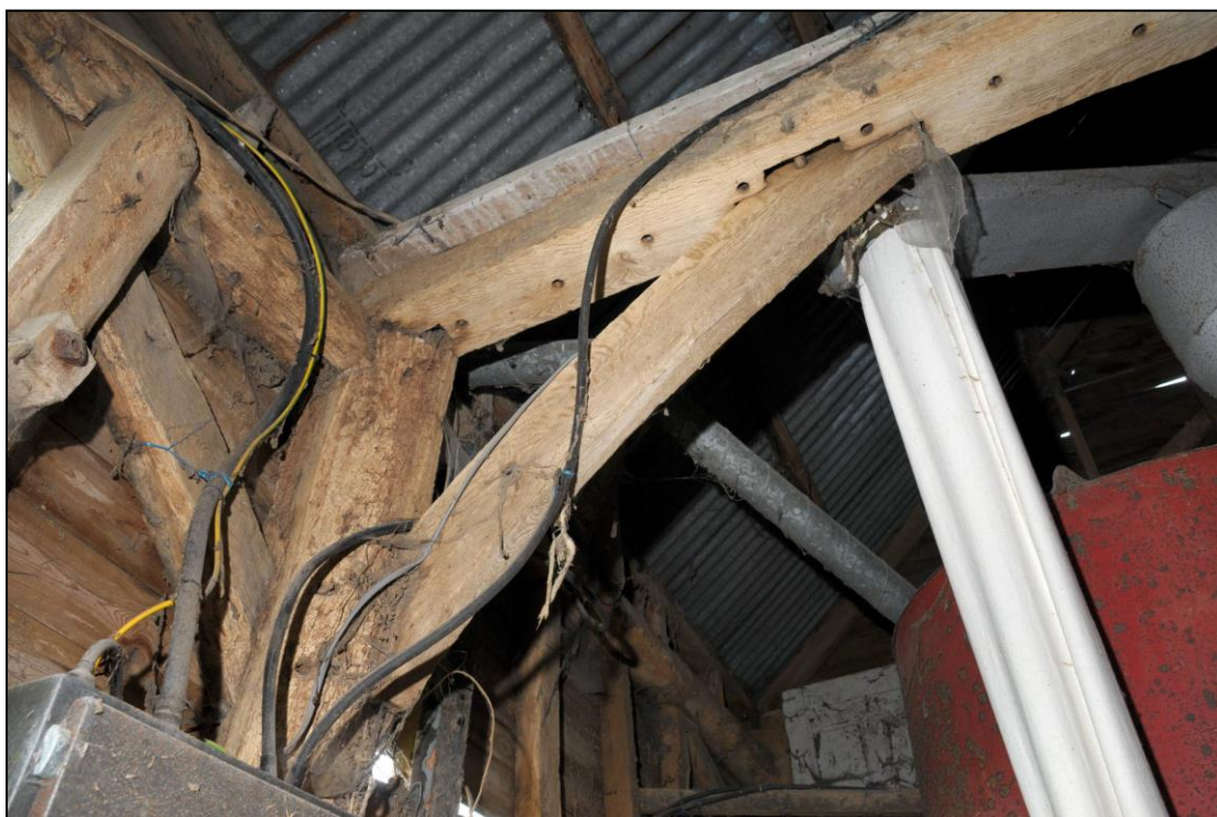
Image 12: Barn 1, interior north wall
