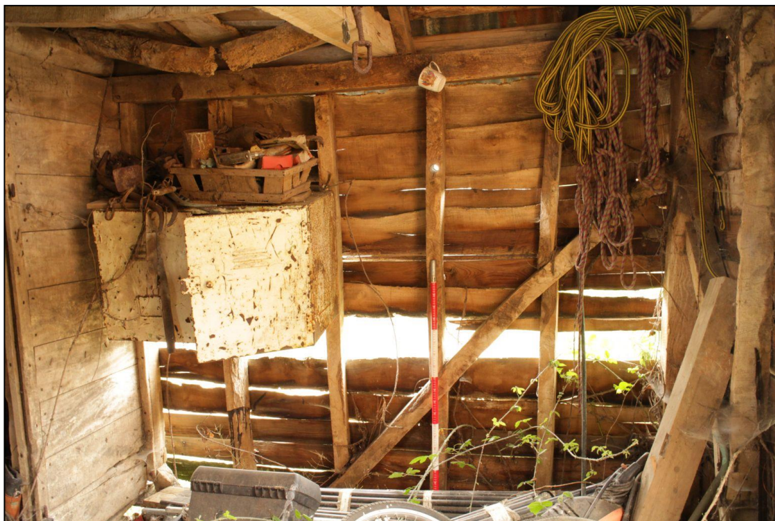
Image 27: Granary interior, west wall
