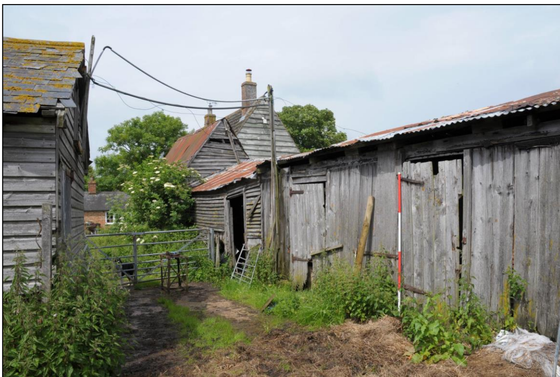
Image 34: Buildings 3 and 4, exterior
