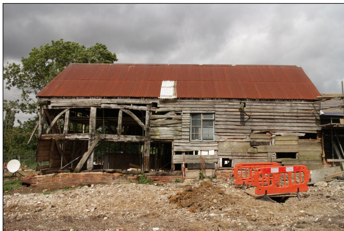
Image 6: Barn 1, exterior south side
