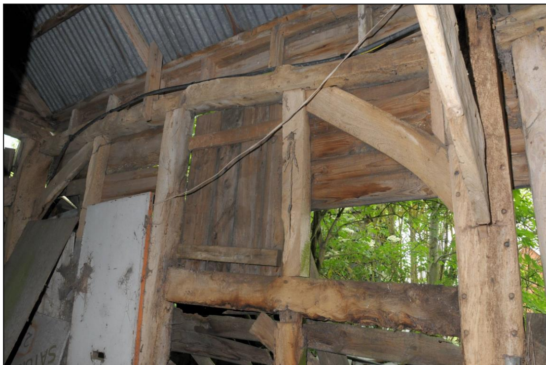
Image 9: Barn 1, interior north wall
