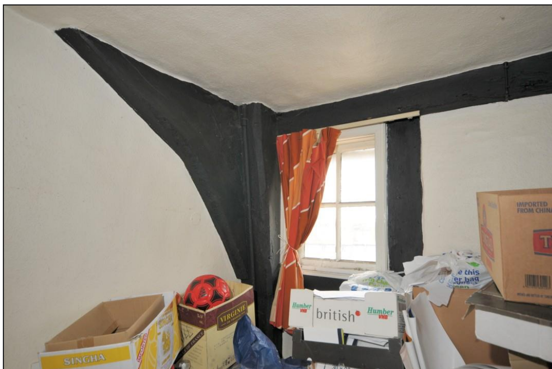
Image 9: No. 69 north-west cross-wing, first floor F2
