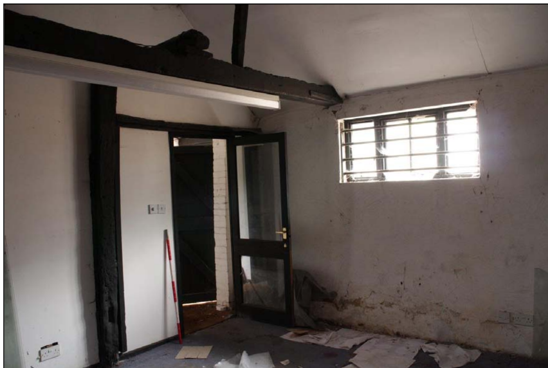
Image 44: Outbuilding, compartment C2
