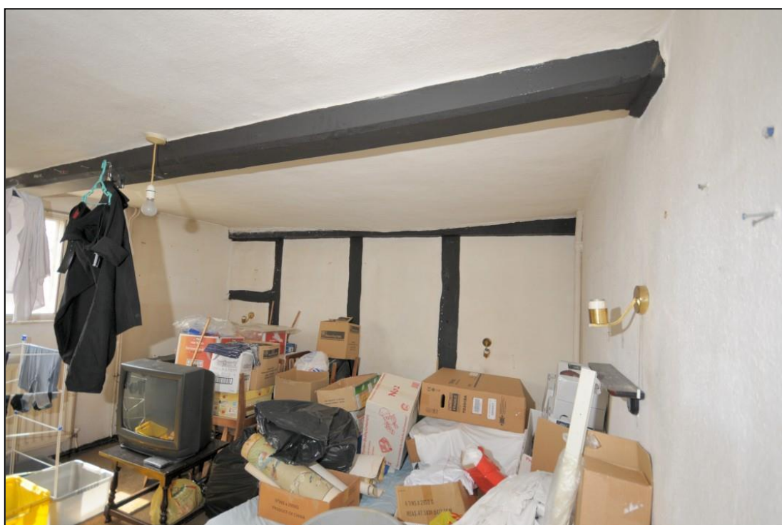
Image 10: No. 69 north-west cross-wing, first floor F1
