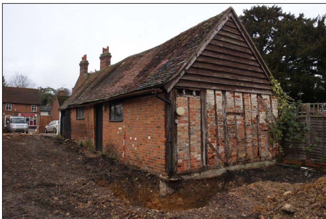
Image 38: Outbuilding, east end and south front
