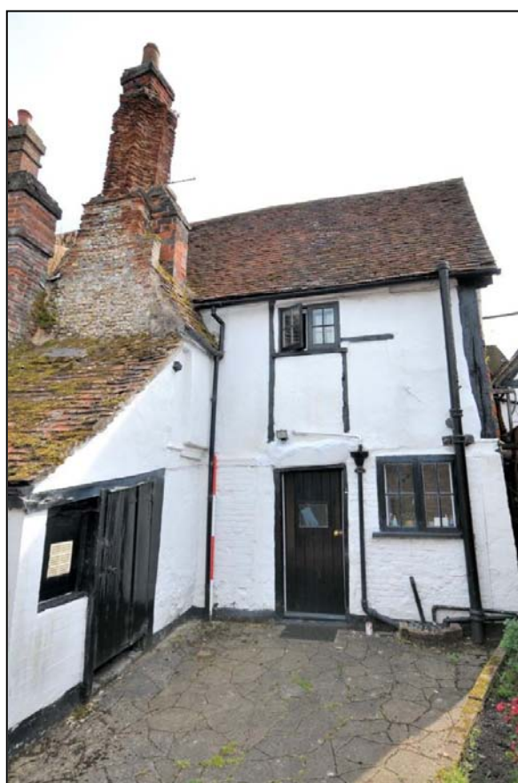
Image 6: Rear elevation of No. 71
