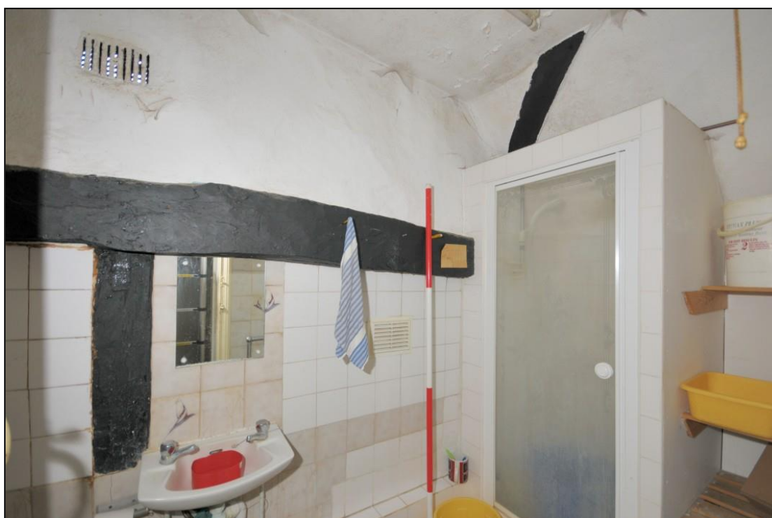
Image 24: No. 69 south-east cross-range, first floor F6
