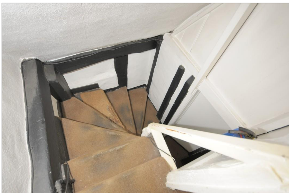
Image 14: No. 69 north-west cross-wing, second floor stairs
