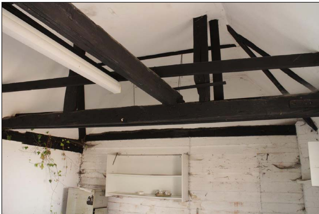
Image 45: Outbuilding, compartment C4
