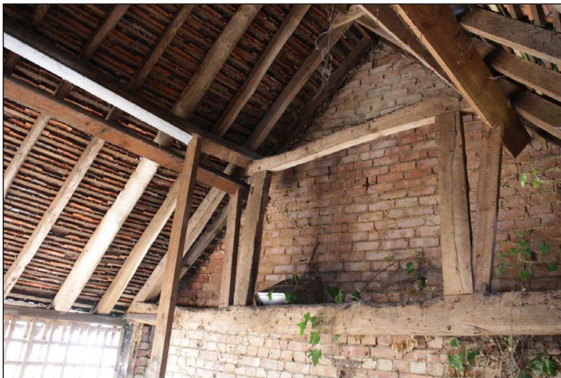
Image 43: Outbuilding, compartment C1 roof structure
