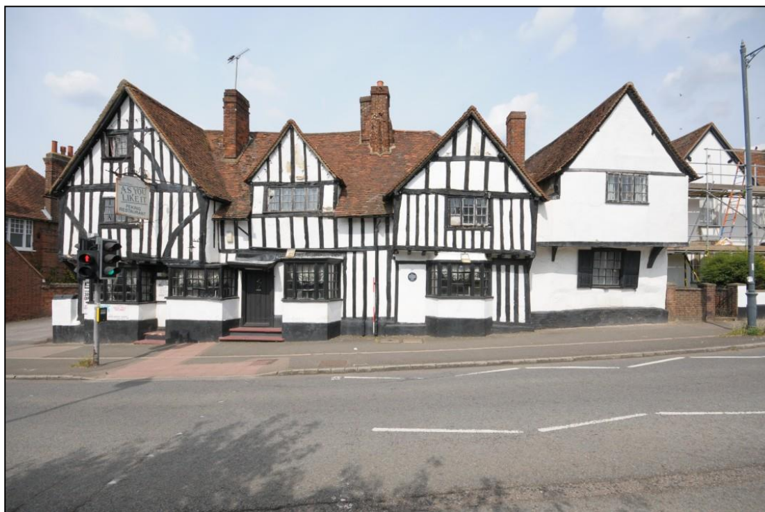
Image 1: South-west elevation of Nos. 69 and 71
