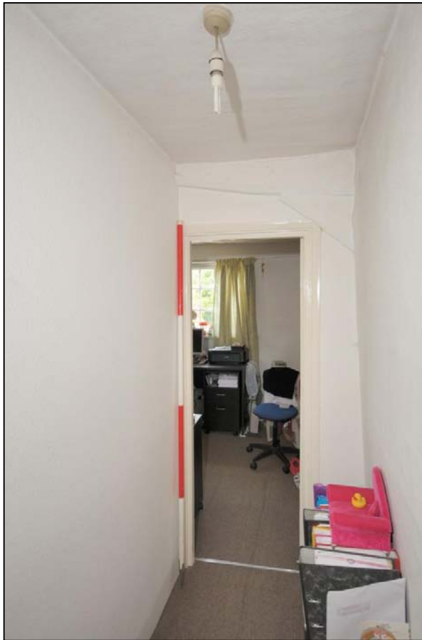
Image 31: No. 71 front-range, first floor landing
