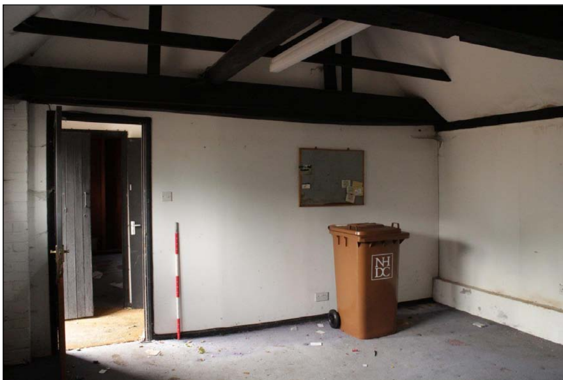
Image 46: Outbuilding, compartment C4
