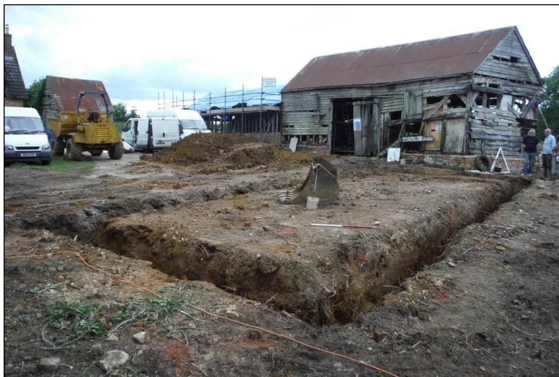
Image 1: Area 1, Pond Barn, Showing completed trenches
