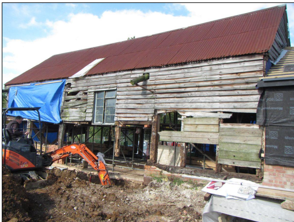
Image 7: Area 3, Dairy Barn, underpinning works
