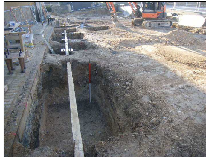
Overview of post-pads, looking south-east (scale 1m)
