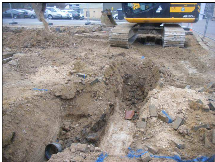
Overview of northern foundation, looking south-west
