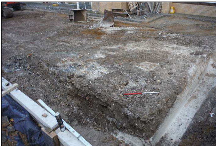
Overview of L-shaped foundation, looking north (scale 1m)
