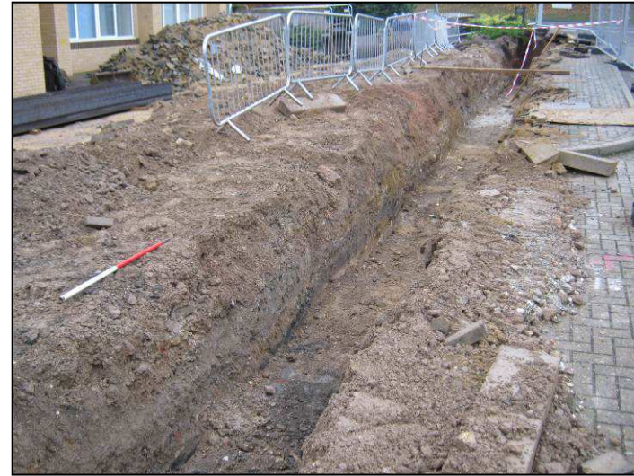
Overview of retaining wall foundation, looking east (scale 1m)
