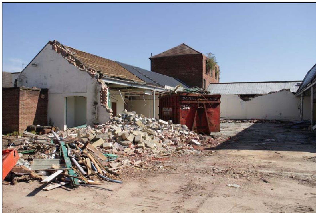
Image 5: Exterior view from yard
