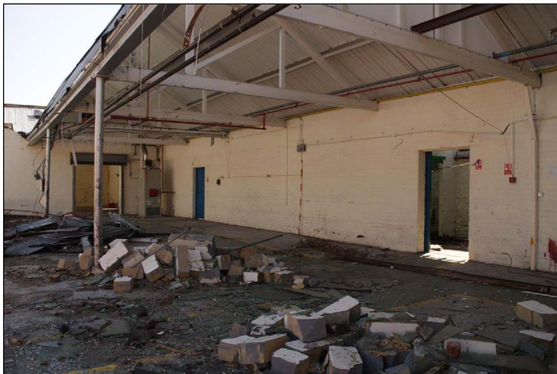
Image 13: Workshop 4, Area 4c Looking south-east (scale 2m)
