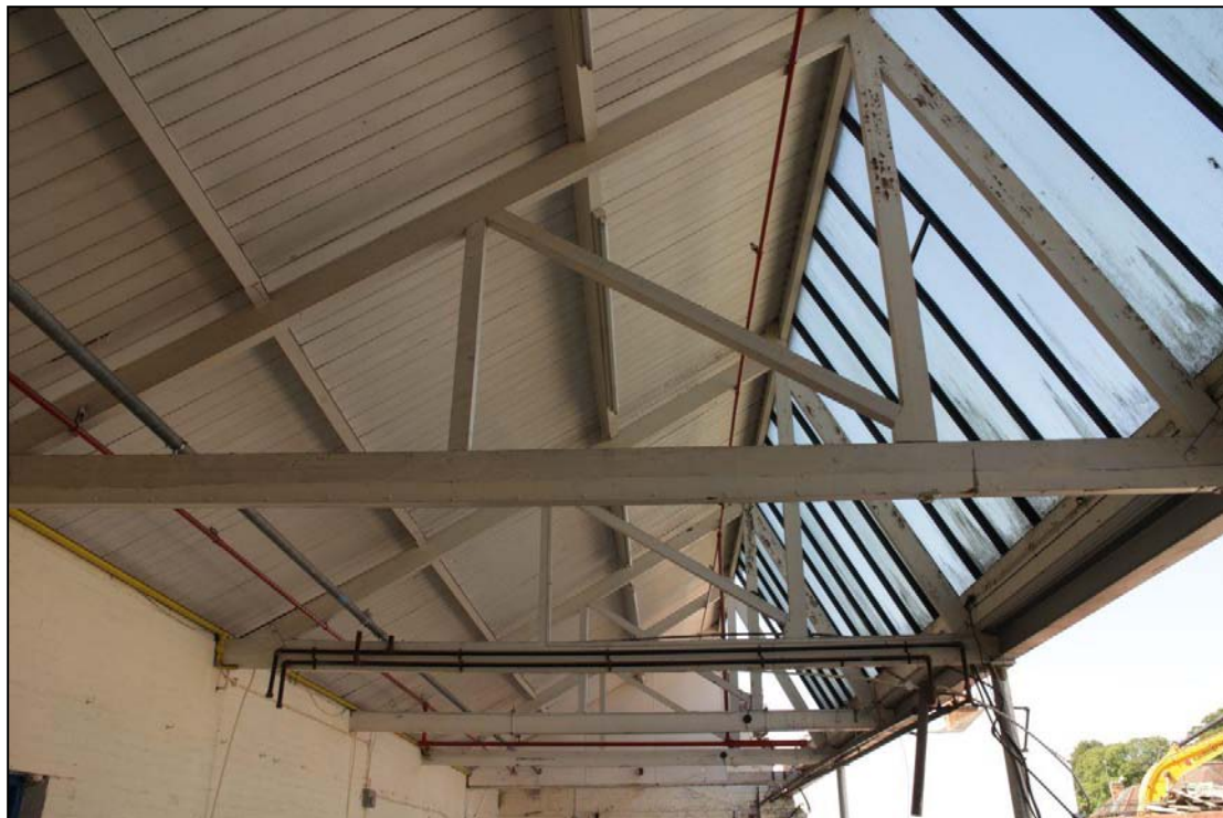
Image 14: Workshop 4, Area 4c Looking west showing roof structure
