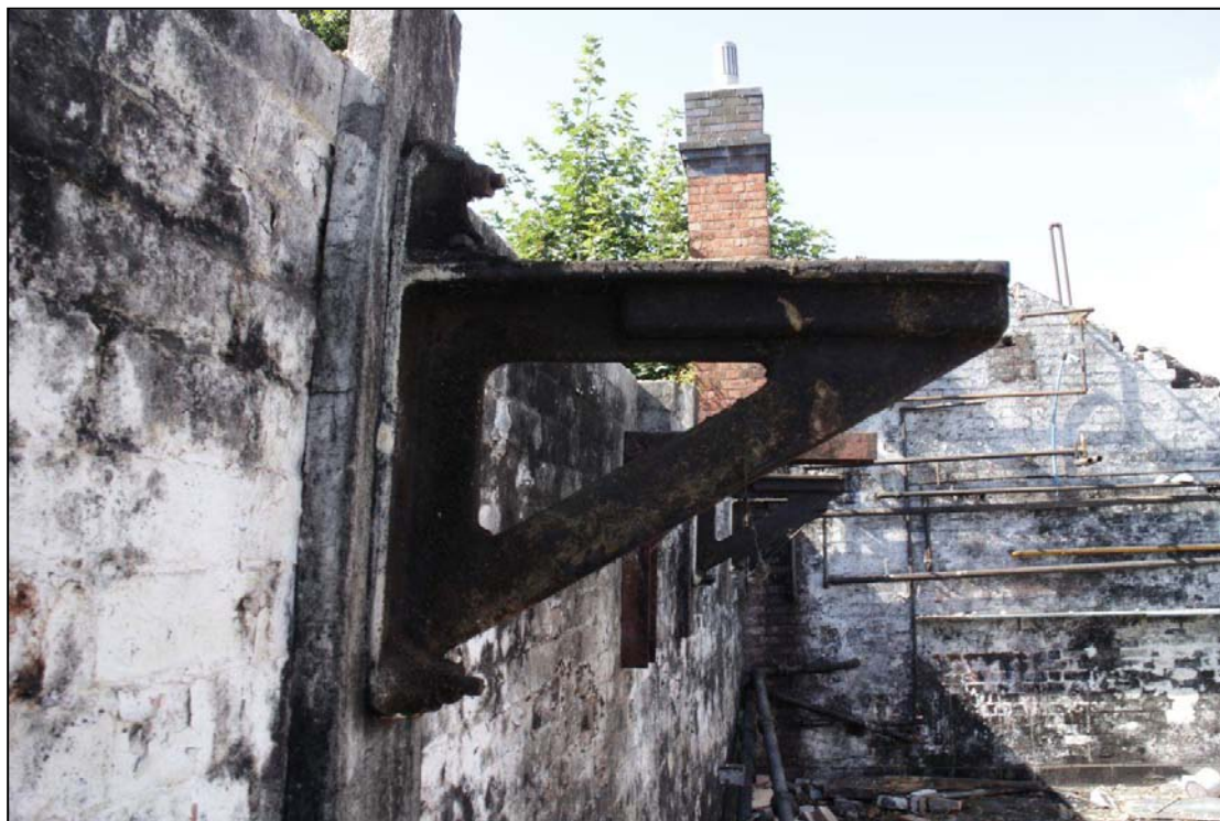
Image 30: Detached workshop 12, Detail of line shaft bracket Looking west showing cast iron line shaft bracket bolted to north wall
