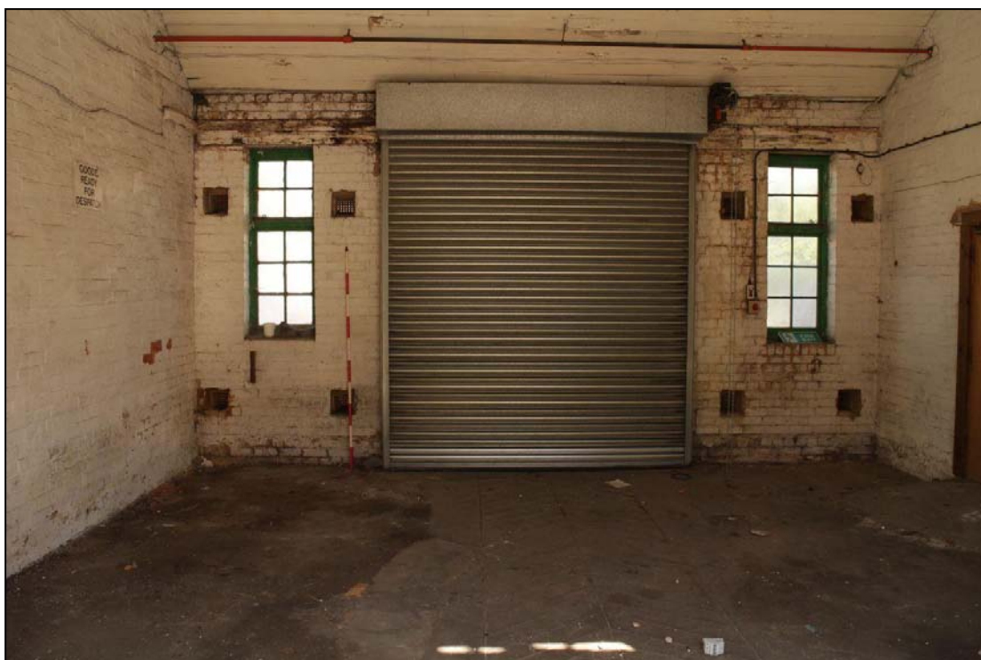
Image 12: Goods loading bay 3
