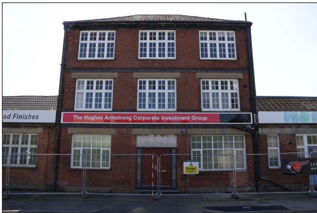
Image 3: Front elevation, three-storey block
