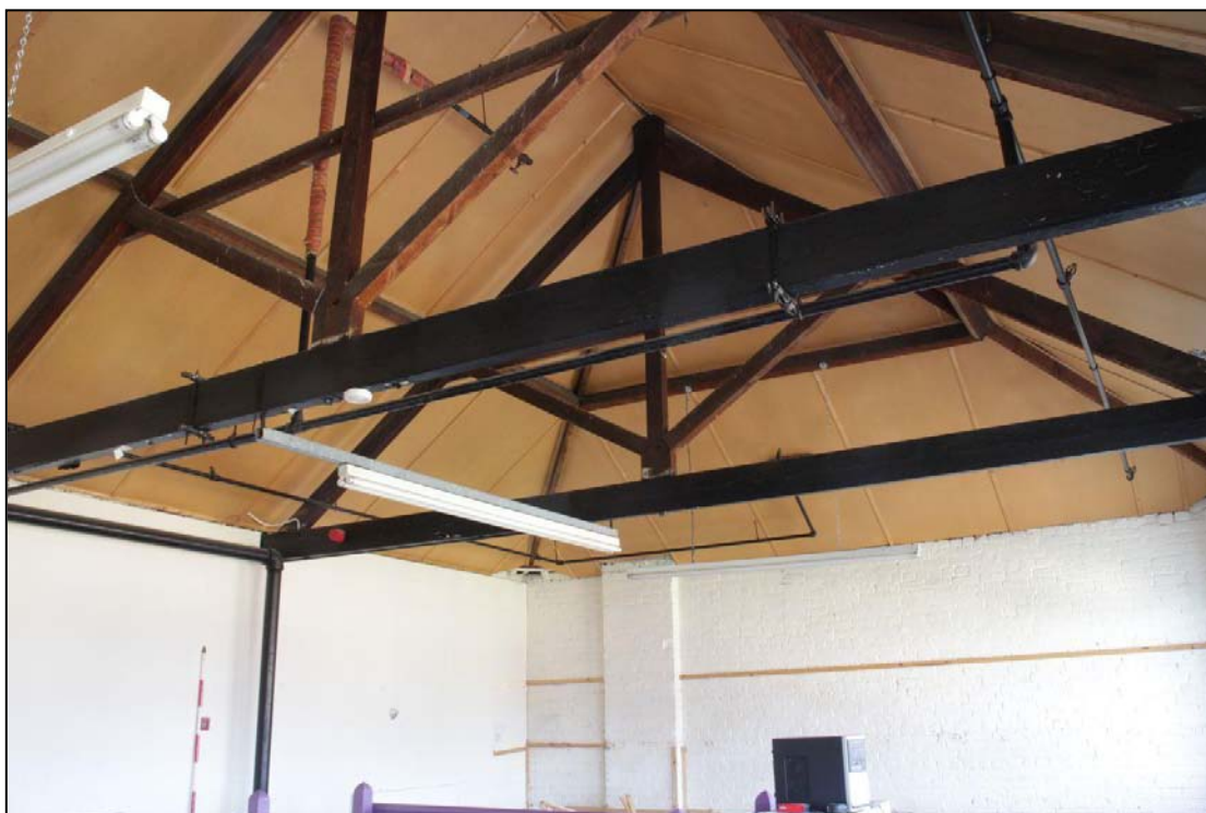
Image 11: Second floor of three-storey block 1
