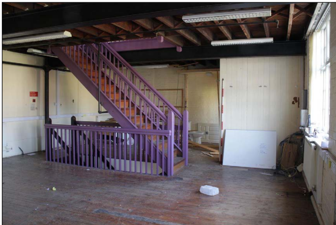
Image 9: First floor of three-storey block 1 Looking south-west (scale 2m)
