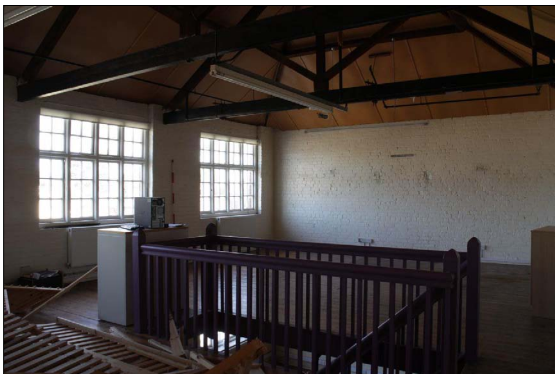
Image 10: Second floor of three-storey block 1 Looking north-east
