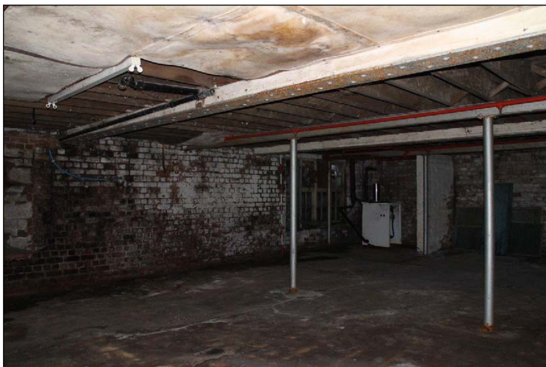
Image 6: Basement, east compartment
