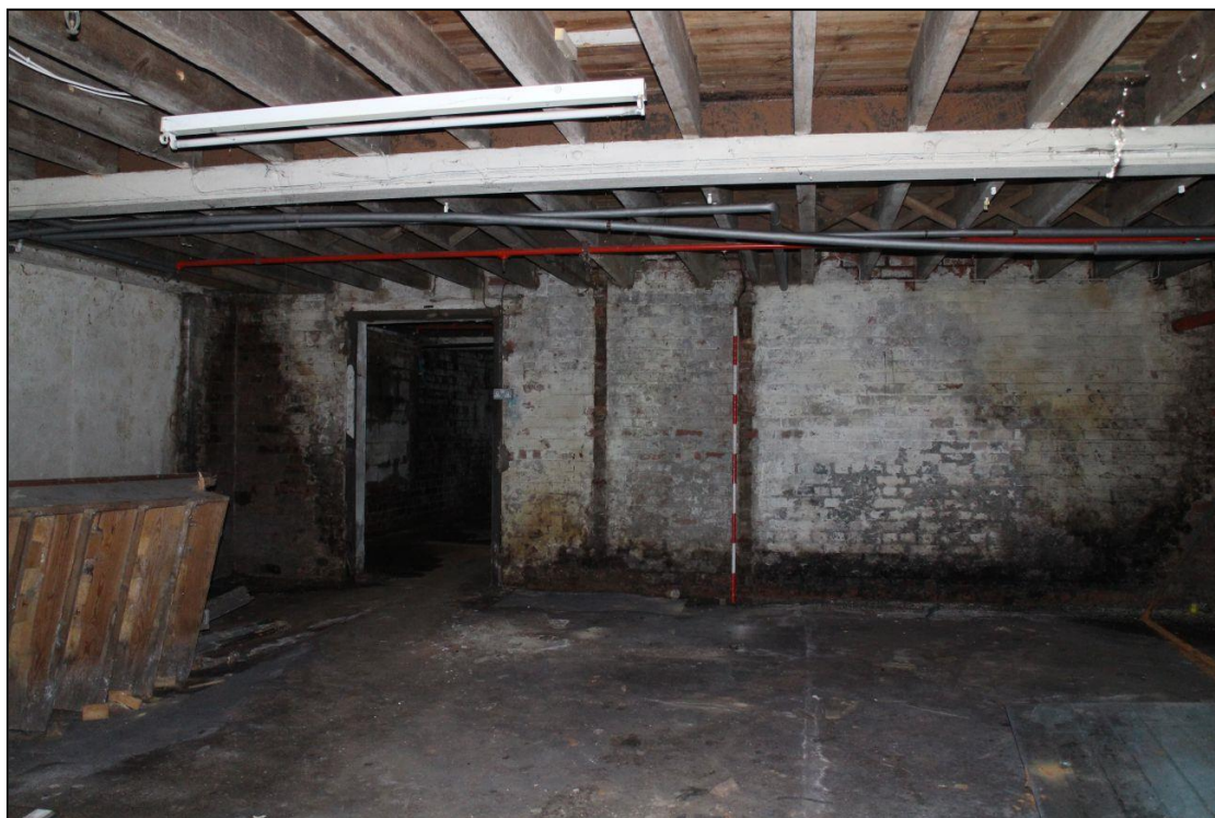
Image 7: Basement, west compartment
