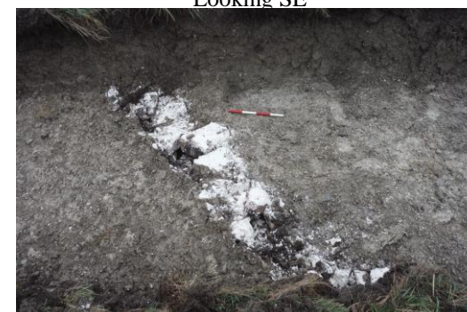
Tr 10. French land drain, Scale 40cm. Looking S.
