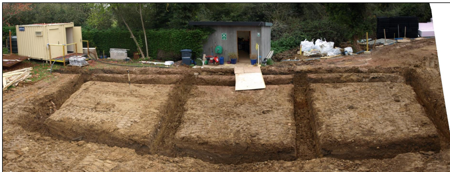
Plate 2: Panorama of non-basement area strip, looking north-west (created using AutoStitch)
