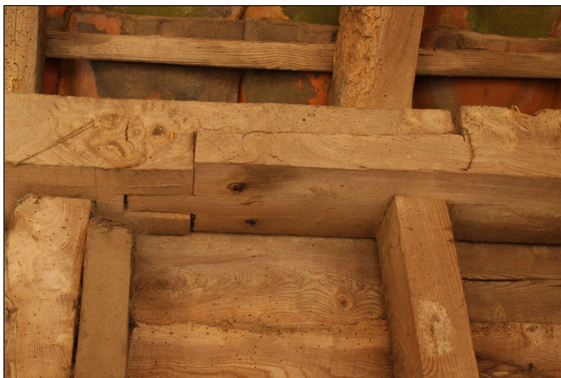
Image 12: Shelter shed, scarf joint in wall plate in north wall
