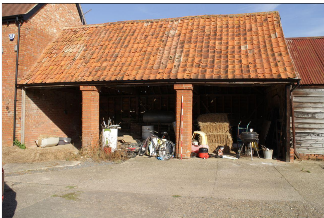
Image 4: Shelter shed, south elevation
