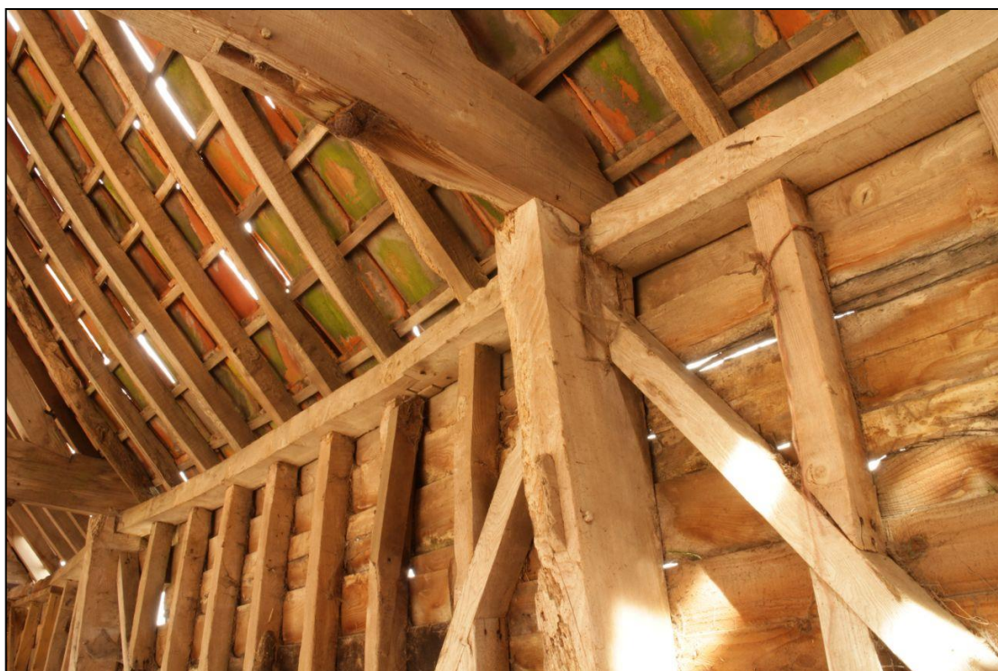
Image 13: Shelter shed, frame detail
