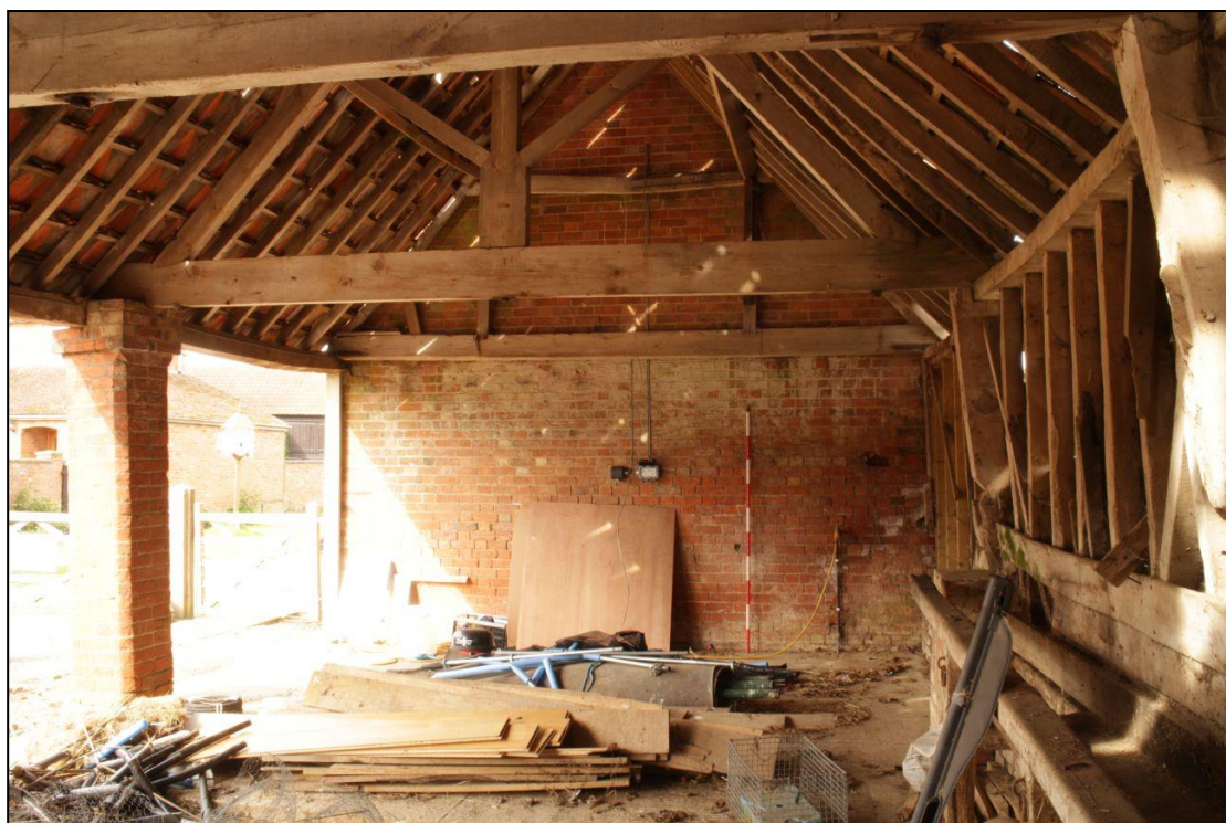
Image 8: Shelter shed, interior looking west
