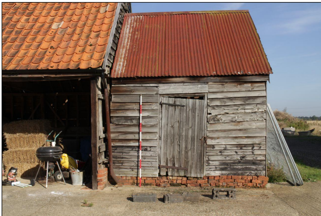
Image 19: Storage shed, south elevation
