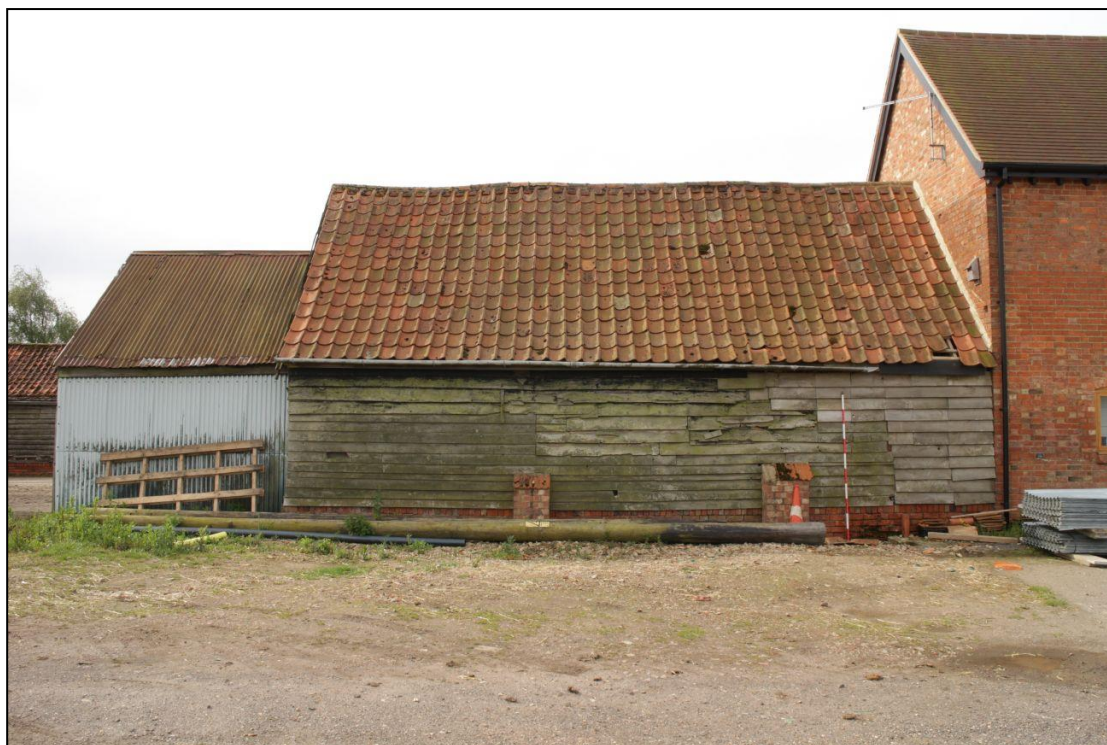
Image 5: Shelter shed and storage shed, north elevation
