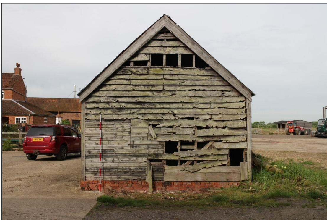
Image 20: Storage shed, east elevation
