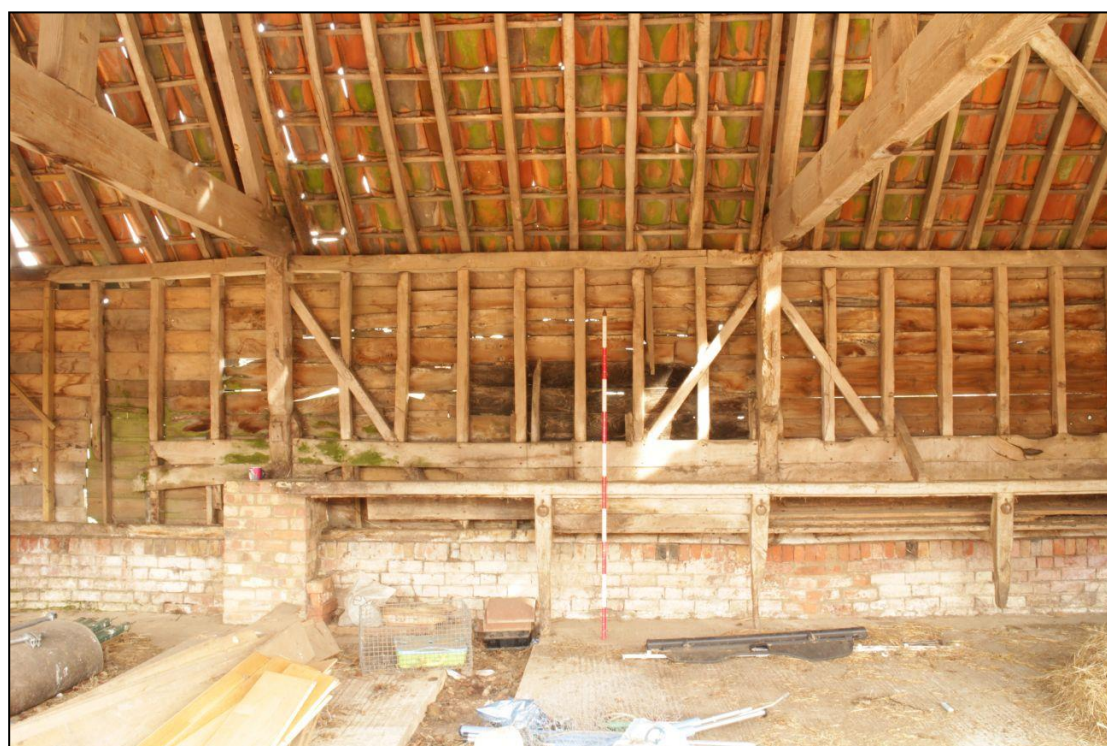
Image 10: Shelter shed, north wall, central bay
