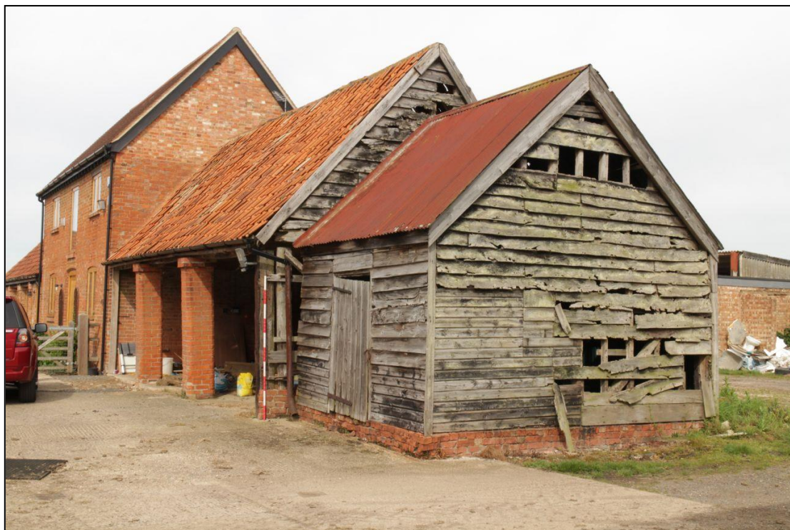
Image 3: General view looking north-west
