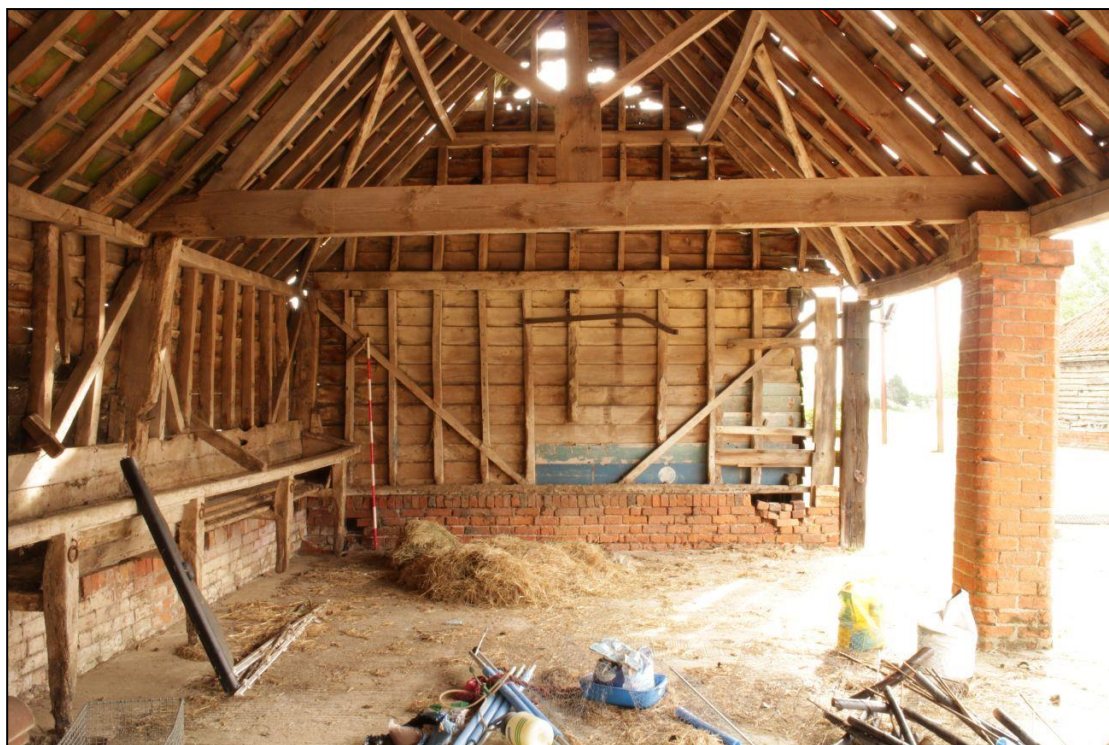
Image 7: Shelter shed, interior looking east
