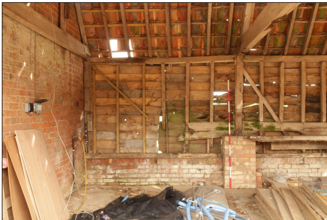
Image 9: Shelter shed, north wall, west bay
