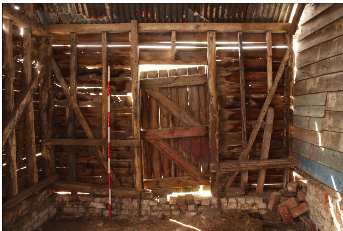
Image 21: Storage shed, south wall
