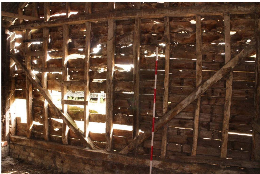
Image 23: Storage shed, east wall
