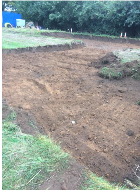
Image 1: General view of house footprint, showing soil profile and undisturbed geological strata
