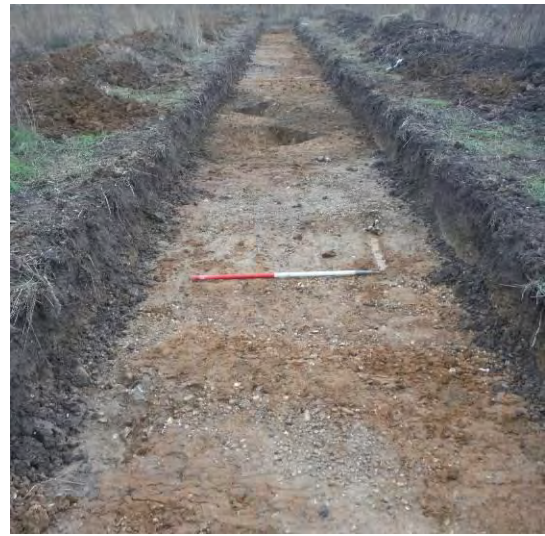
View of Trench 6 looking south-west
