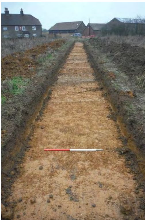
View of Trench 31 looking south-west
