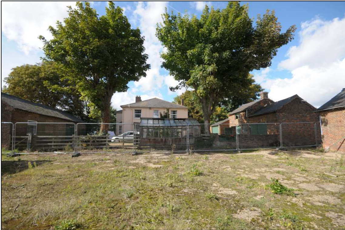
Image 1: General view across farmyard, looking towards farmhouse Temporary fencing marks extent of buildings not subject to demolition
