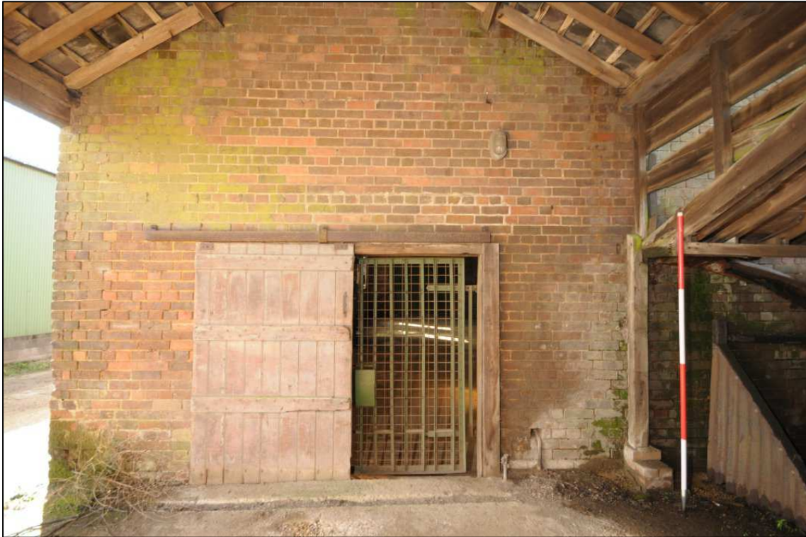
Image 27: East range: north end wall
