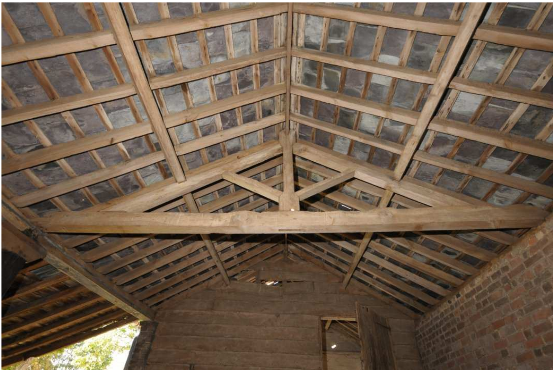
Image 16: North range: compartment C3, roof structure
