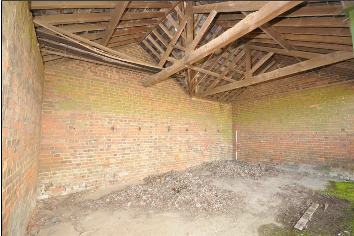
Image 21: North range: compartment C5, interior looking south-west
