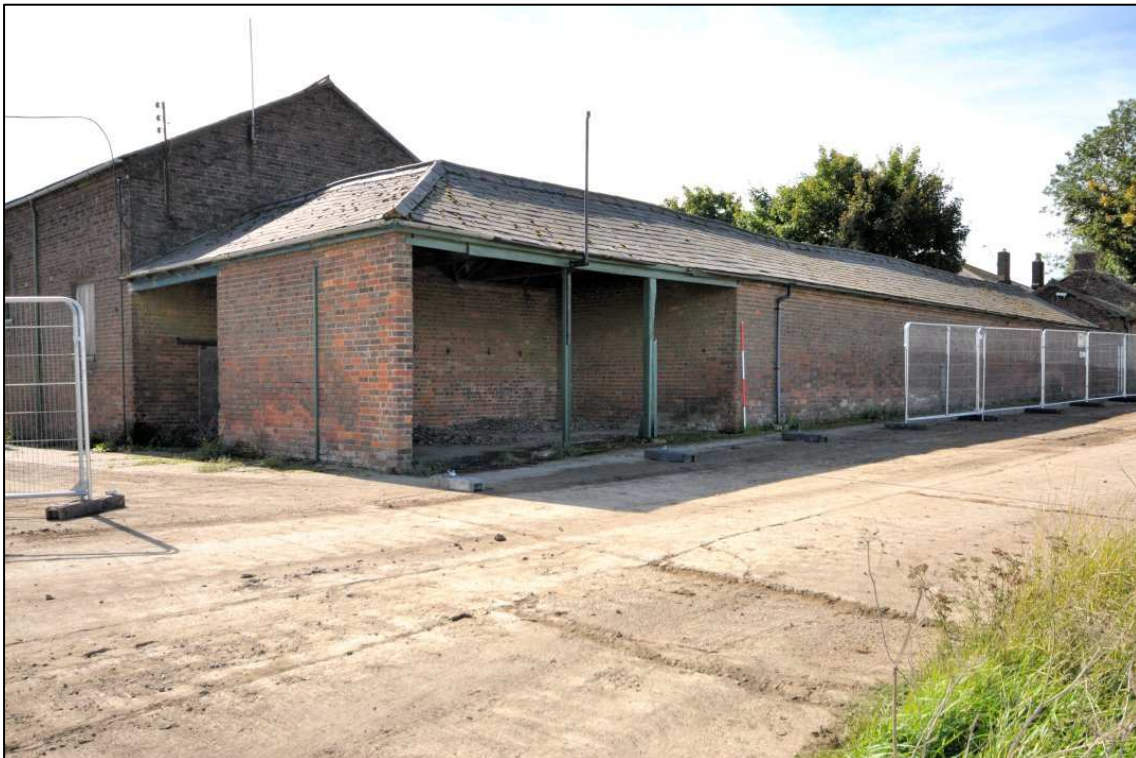
Image 20: North range: compartment C5 exterior, looking south-west
