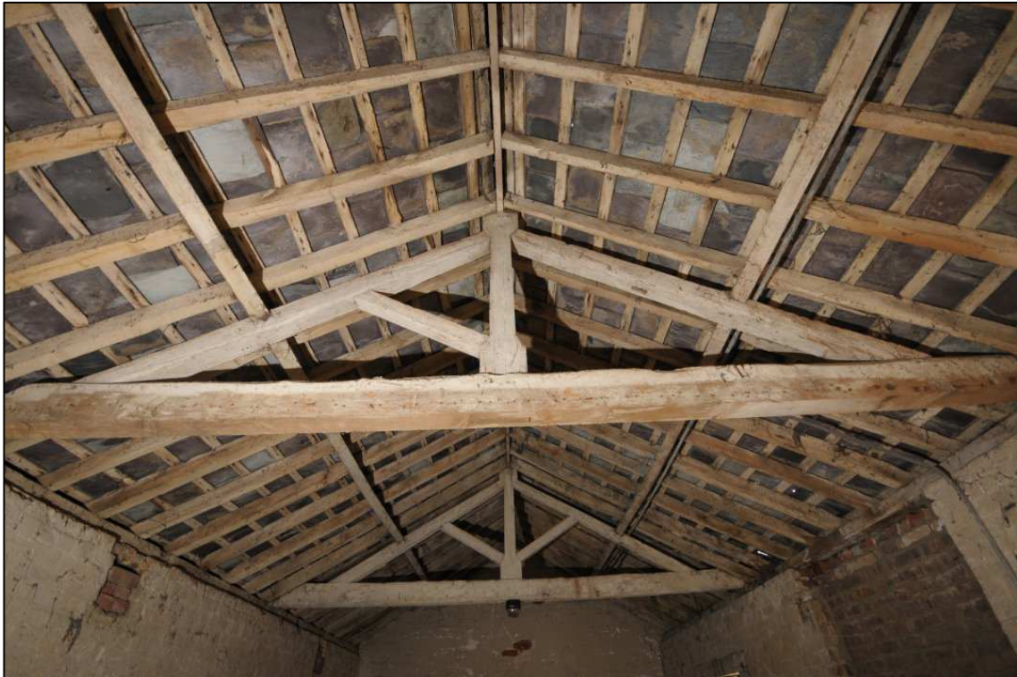
Image 9: North range: compartment C1, roof structure
