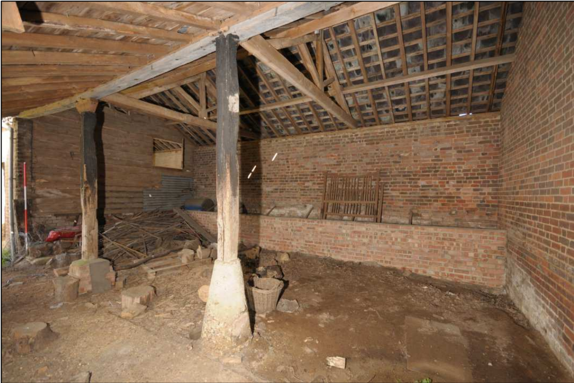
Image 15: North range: compartment C3, looking north-west
