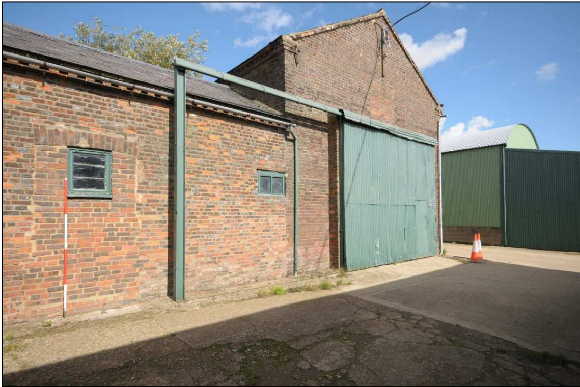
Image 23: East range: exterior of south end
