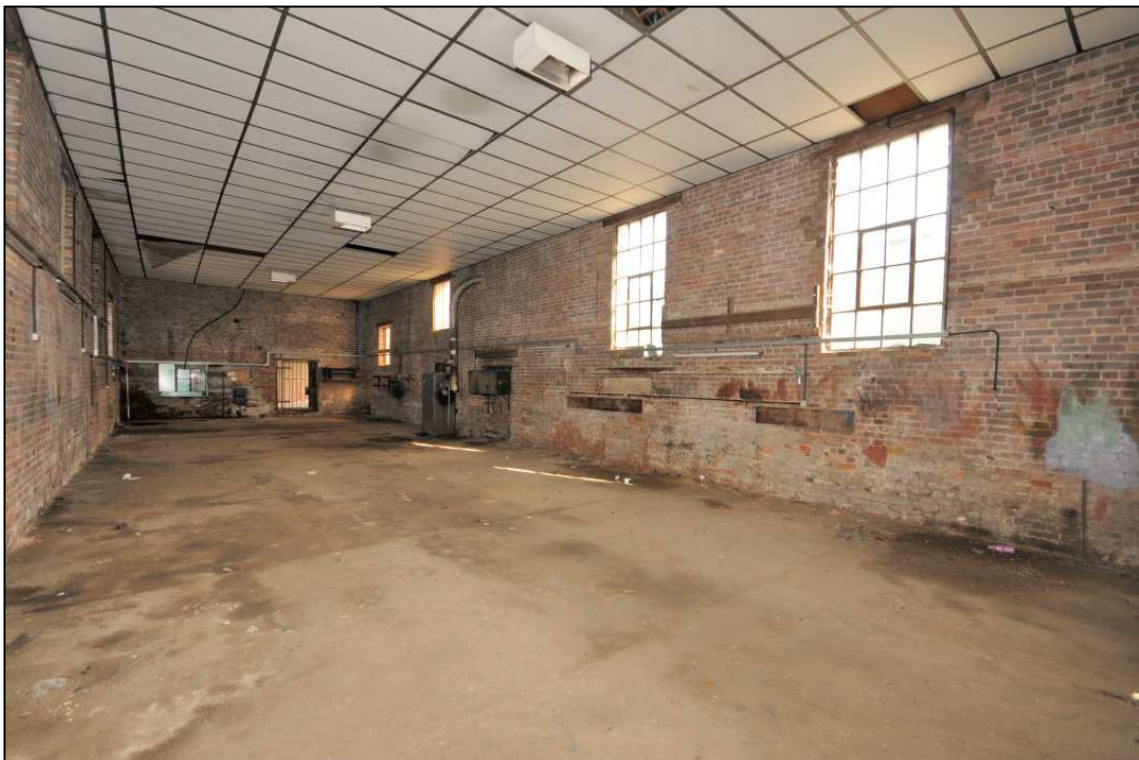
Image 30: East range: interior looking north-east
