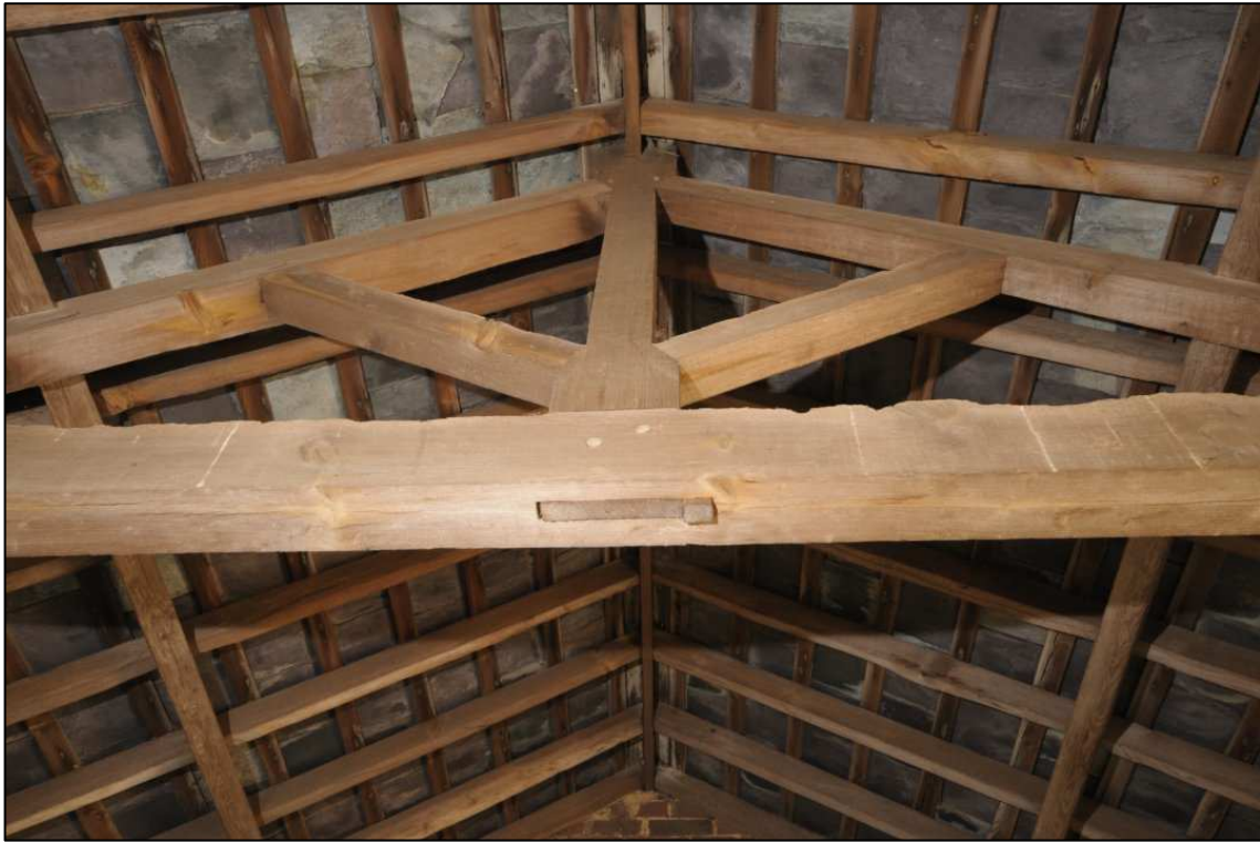
Image 45: Detail of kingpost roof truss in north range
