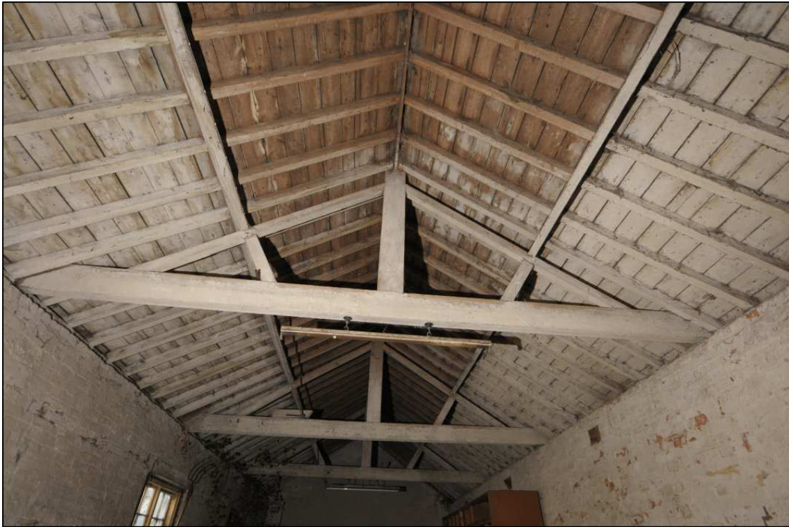
Image 39: South range: compartment C8, roof structure
