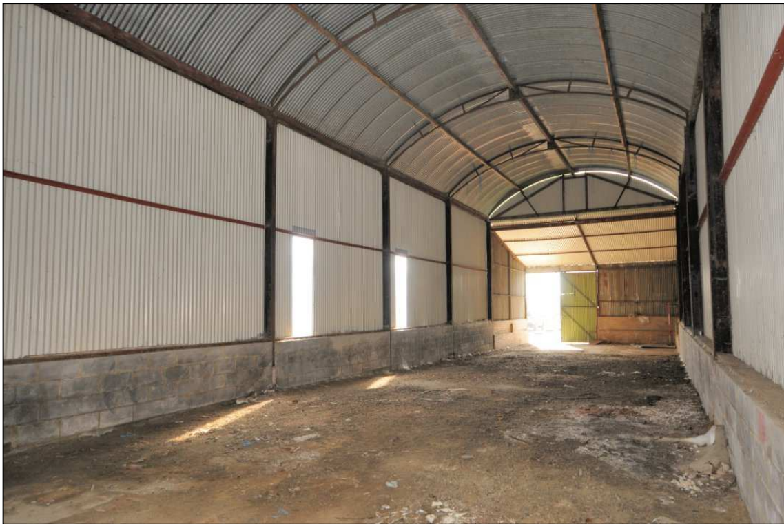
Image 41: Dutch barn to east of farmyard (DB1), interior Looking south
