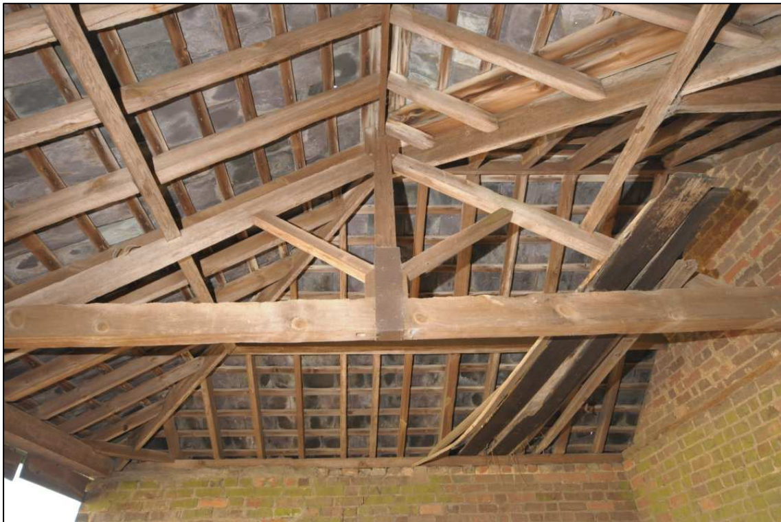
Image 22: North range: compartment C5, roof structure
