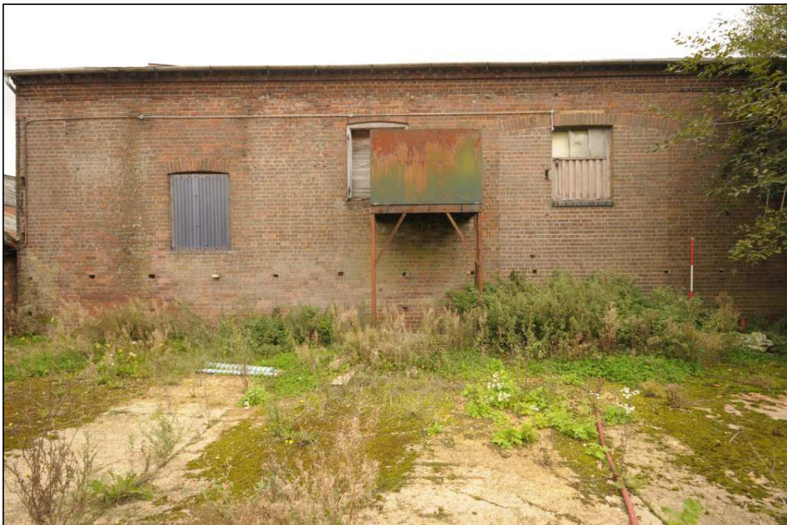
Image 28: East range: exterior of west side
