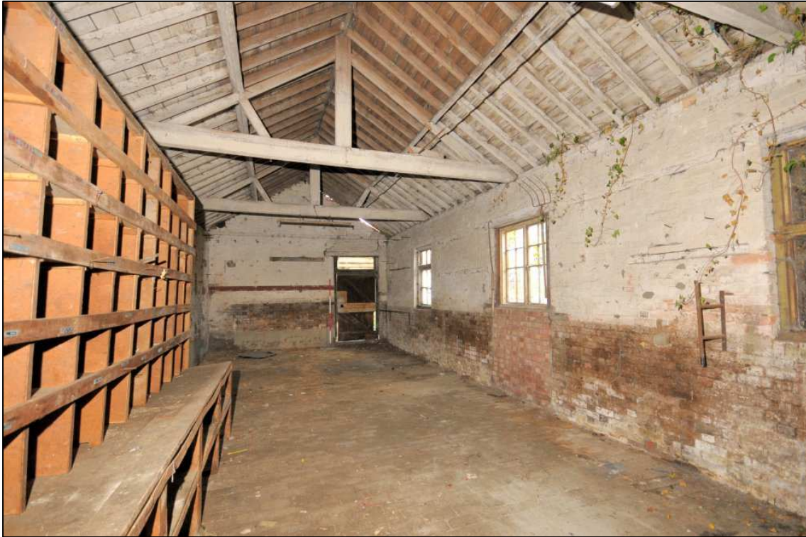
Image 37: South range: interior of compartment C8, looking west
