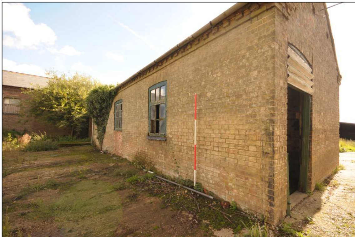
Image 36: South range: exterior of compartment C8, north side and west end
