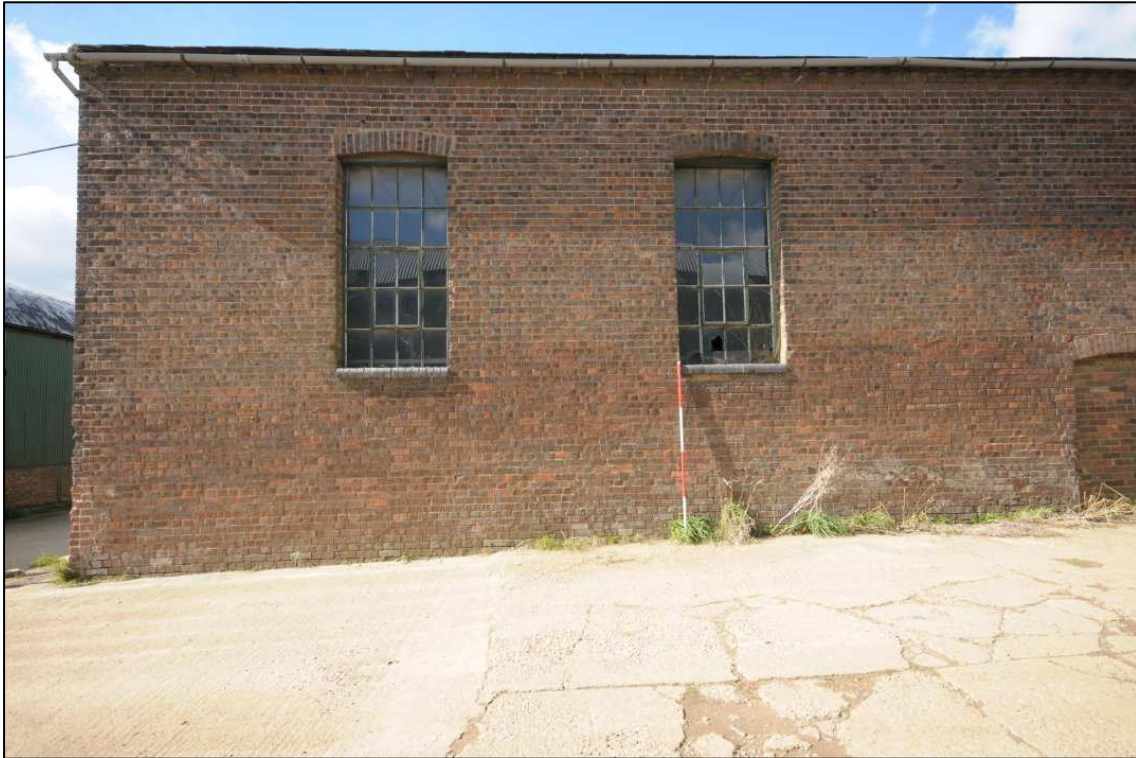
Image 25: East range: east wall, south half
