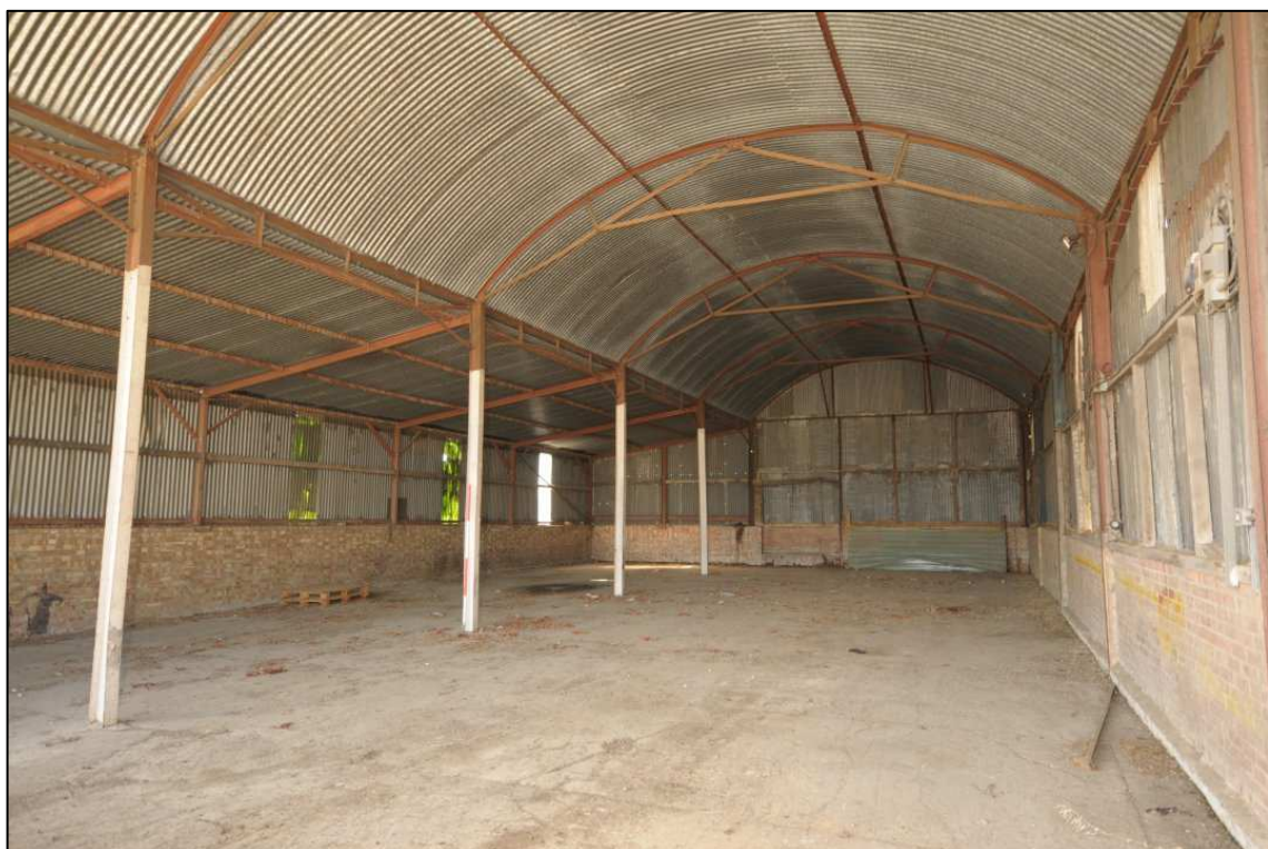
Image 42: Dutch barn to south of farmyard (DB2) Looking west
