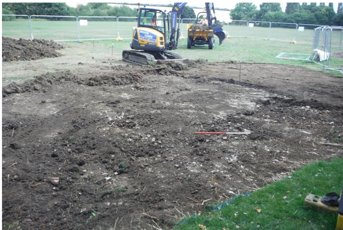
Plate 17: Off-site car park — ground reduction underway
