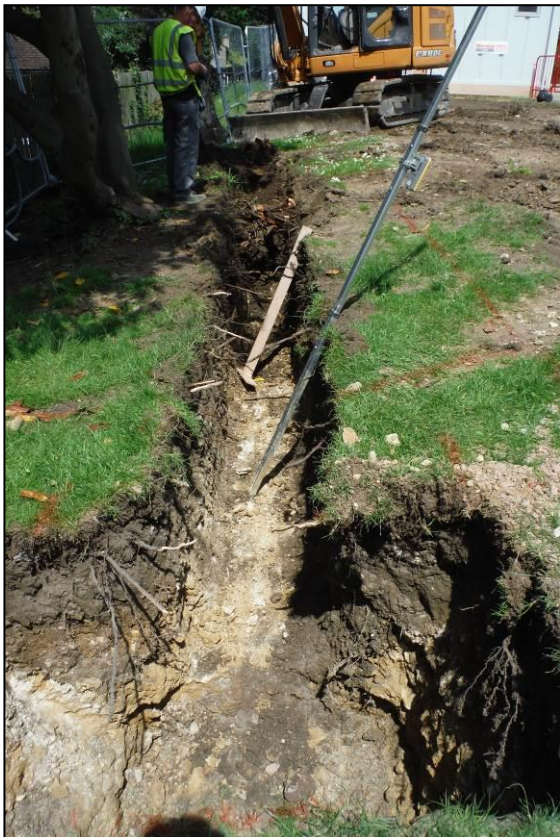
Plate 10: Service Trench 2, looking north
