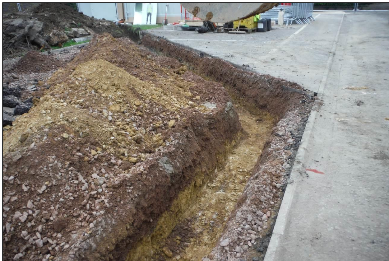
Plate 5: Service Trench 1, looking north
