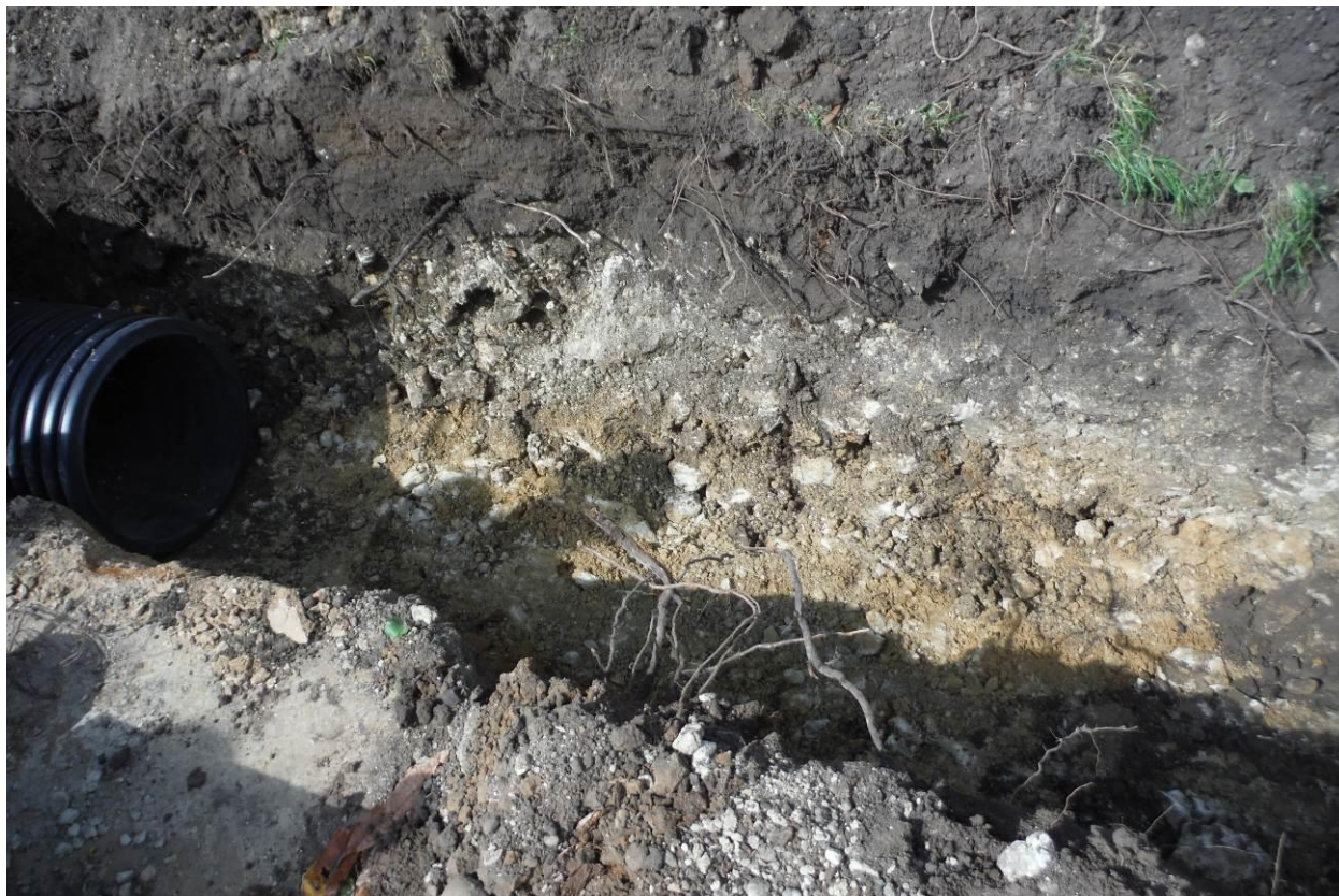
Plate 12: Service Trench 2, northern extent of east-facing baulk section
