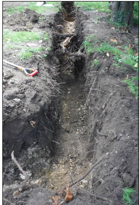
Plate 11: Service Trench 2, looking south
