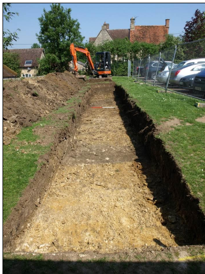
Plate 2: Trial Trench 1, looking north
