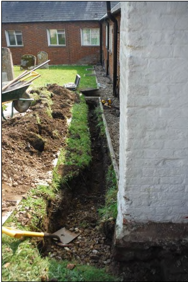
Plate 3: Foul-drain trench, looking east
