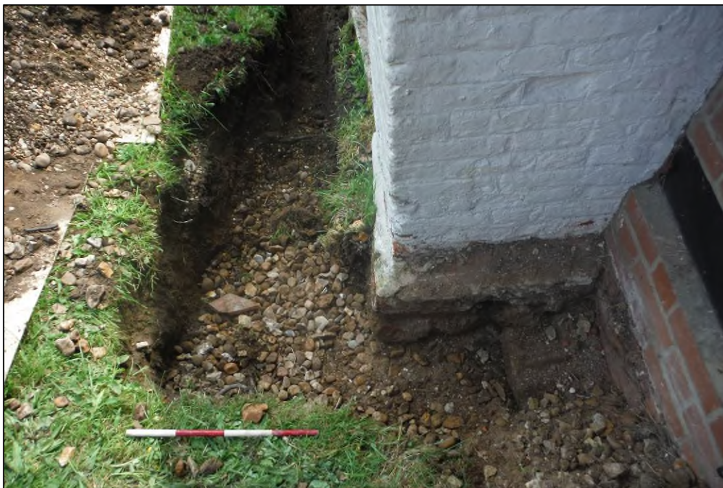
Plate 6: Western section of foul-drain trench, showing foundation of No. 1 Feoffee Almshouses, looking east (scale 0.4m)
