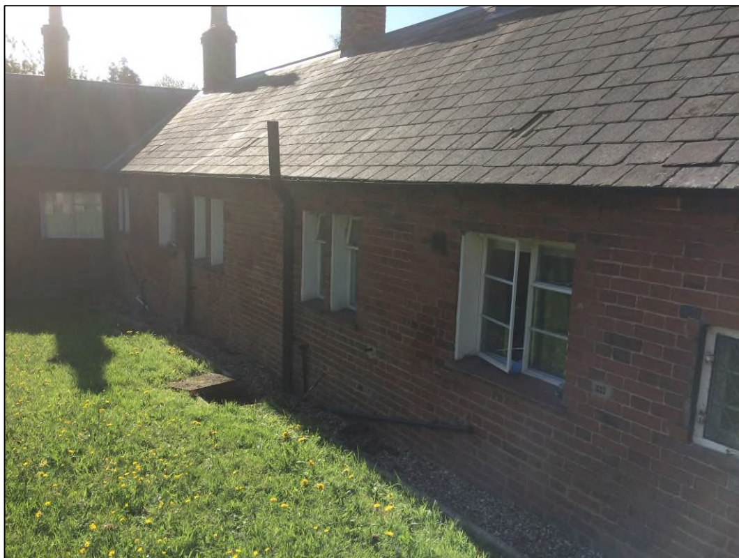
Plate 1: North side of No. 5 Feoffee Almshouses, prior to the works
