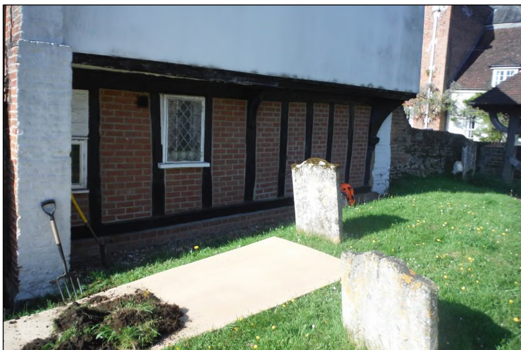
Plate 2: North side of No. 1 Feoffee Almshouses, prior to the works
