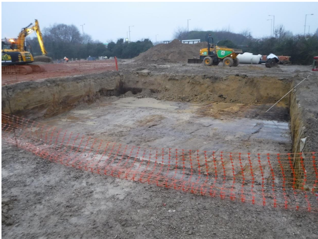
Attenuation tank excavation (AO) (looking north)
