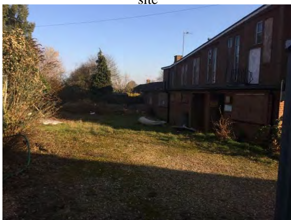
View of the church and eastern side of the site
