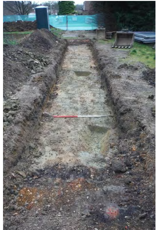
View of Trench 2 looking south
