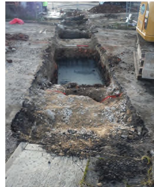
Image 6: Trench 6 – looking south-west (scale 1m)
